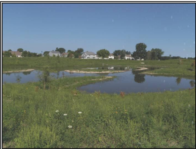
Hollywood Basin After Construction: The storm water wetland provides for reduction in sediment and nutrients and peak flow control for small and large storm events.
