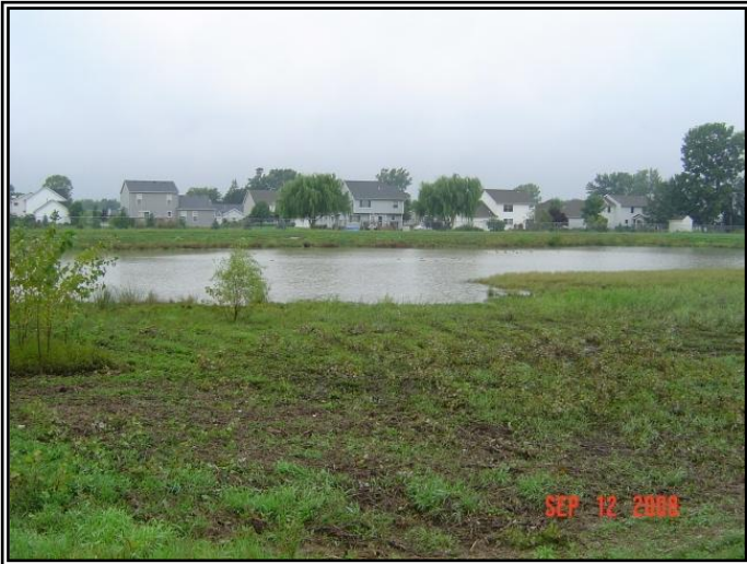
Hollywood Basin Before Construction: Existing detention basin provided virtually no storm water treatment and limited peak flow control.
