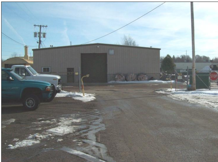
Public Services Utilities Building (PSUB) (Before): PSUB is located at the intersection of Centerville Road and McKee Street in Sturgis, Michigan. Storm water runoff previously would have transported sediment, nutrients, and salt to the storm sewer system.
