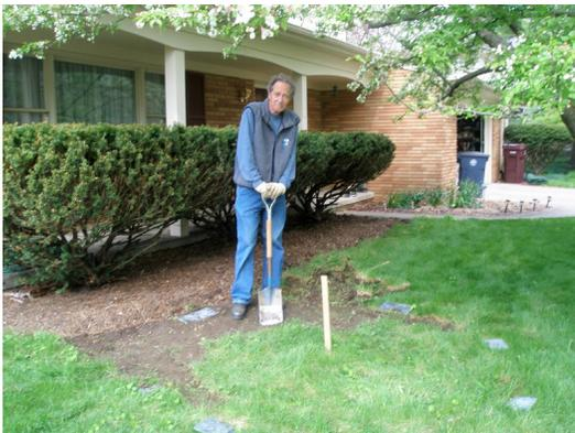
**Roger Moon front yard Before:** This yard in Ann Arbor sent the roof runoff onto a lawn, which then dumped the runoff to the next-door neighbor's driveway. The water then ran down the driveway into a cul-de-sac whose drainage empties into the piped stormwater system and into the Huron River.
