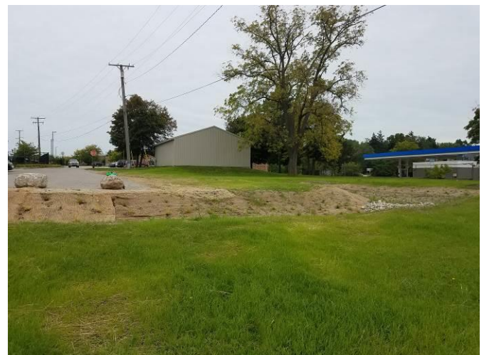
Hogback After: 3-cell bioinfiltration to capture parking/roof runoff.
