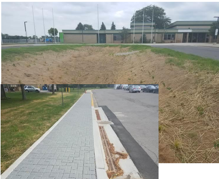
Mitchell School After: Large bioinfiltration cell to capture parking/roof runoff. Porous sidewalk gravel bed storage and drain to capture parking runoff.
