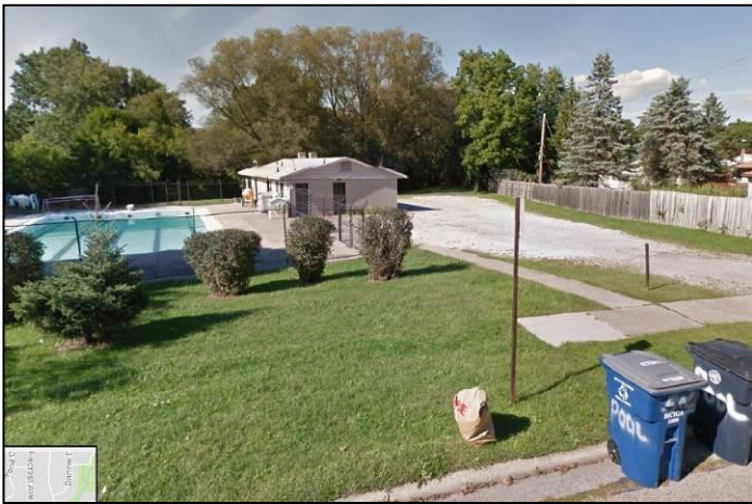
Forestbrooke Before: no stormwater treatment, aging infrastructure, road runoff onto property, direct connection to Swift Run behind pool.
