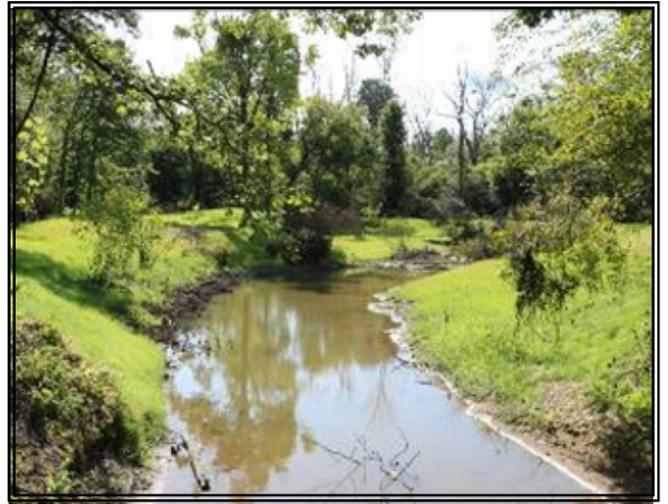
**The Peters Creek Restoration following construction.** Sod mats and erosion blanket were installed for erosion protection, providing immediate cover for late summer storms.
