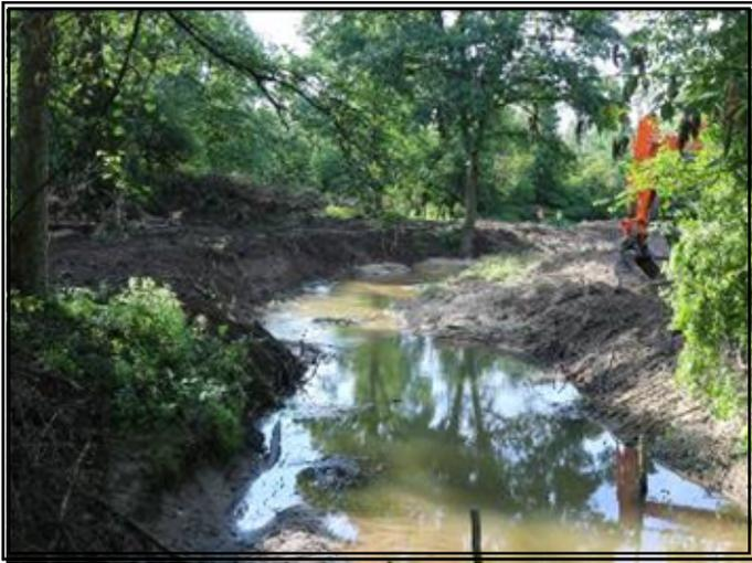
**Peters Creek Stream Restoration (before):** At the start of construction, vegetation and falling trees were removed before the streambanks were shaped to their new contours. Several of the trees were then used as in-stream structures.
