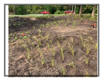
White Pine Trail Site During Construction: Before the wetland restoration road runoff was captured by a storm sewer that exits into the northwest corner of this parcel. Other stormwater onsite flowed directly over a mixture of fill and mowed wetland towards Cedar Creek.
