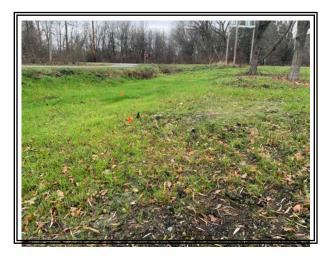
White Pine Trail Site After: Stormwater runoff from one and half acres at this site is treated in a 2,250 cubic foot treatment basin near the road. Over 3,000 native wetland plants, forbs, and trees were planted along the edges of the exposed water areas of the basin, slopes of the overflow berm, and the newly excavated drainage swale.
