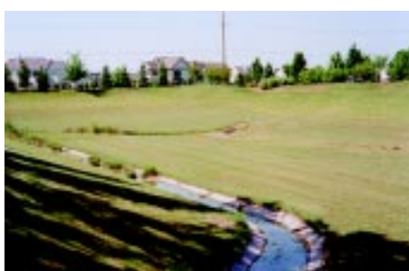
Dry Detention Basin
