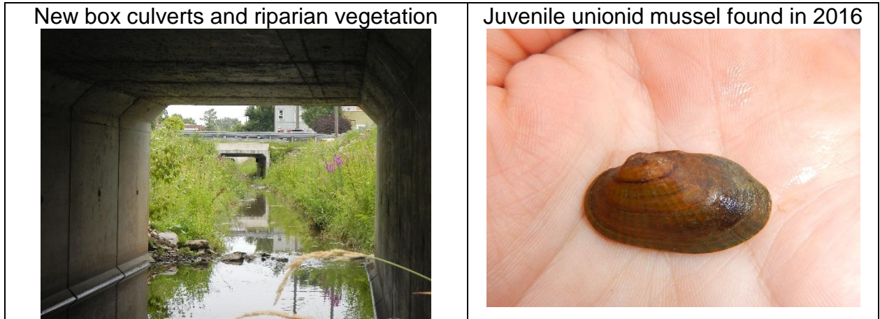
Figure 1. Photographs from Moore Drain.
