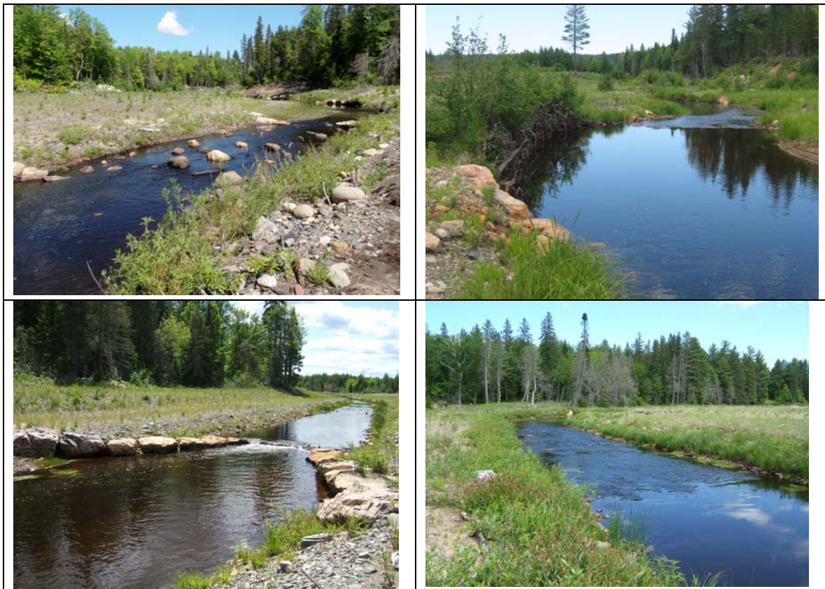
Figure 3. Photographs of the impacted reach 7 years after the dam failed, including some of the instream stabilization structures. Note the regenerating floodplain vegetation.
