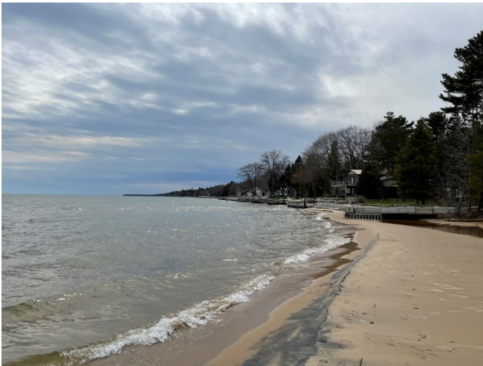
Photo 6: Looking south from the north end of HREA A – Iris Drive in Baldwin Township. Note the significant armoring to the south.
