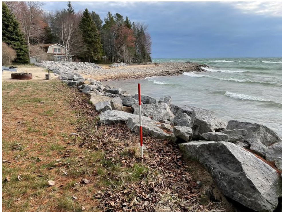
Photo 8: Armored, unarmored, and failed armor in background at HREA C – East Birch Road, Baldwin Township.
