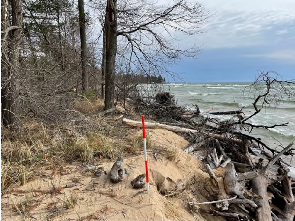
Photo 9: Looking north along EHL in HREA D – Balwin Resort, Baldwin Township. Note the wave cut face and fallen trees.
