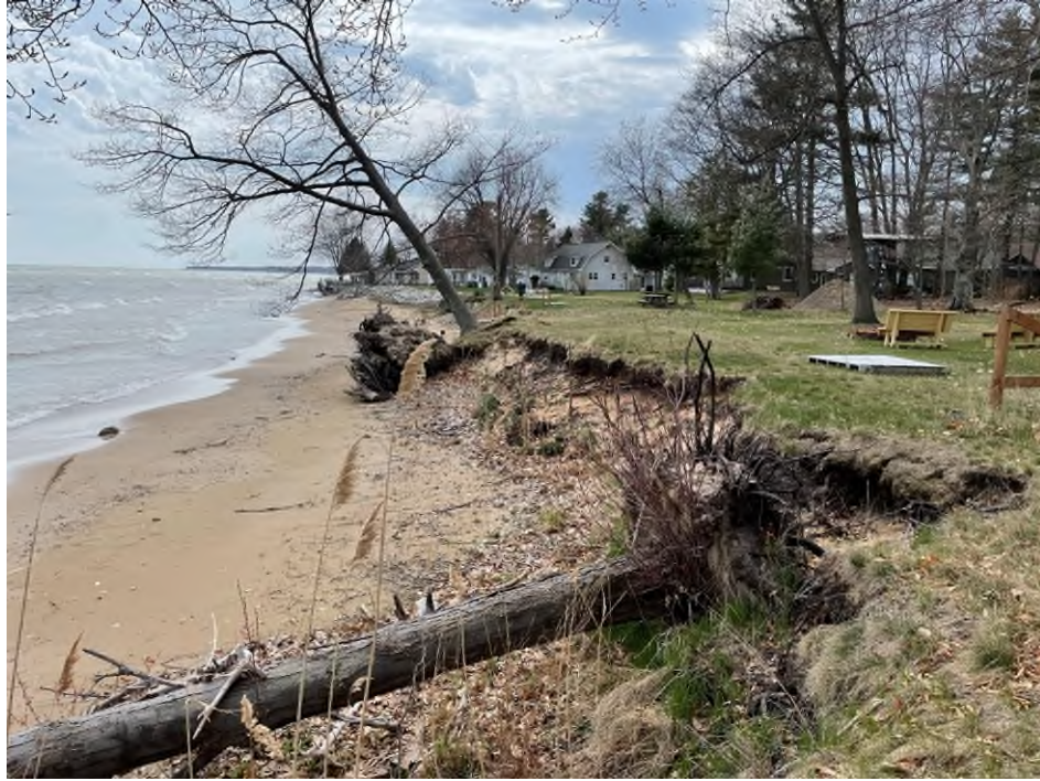
Photo 15: Looking south along EHL in HREA F – Keystone Road, Alabaster Township. Note the actively eroding shoreline and fallen trees.
