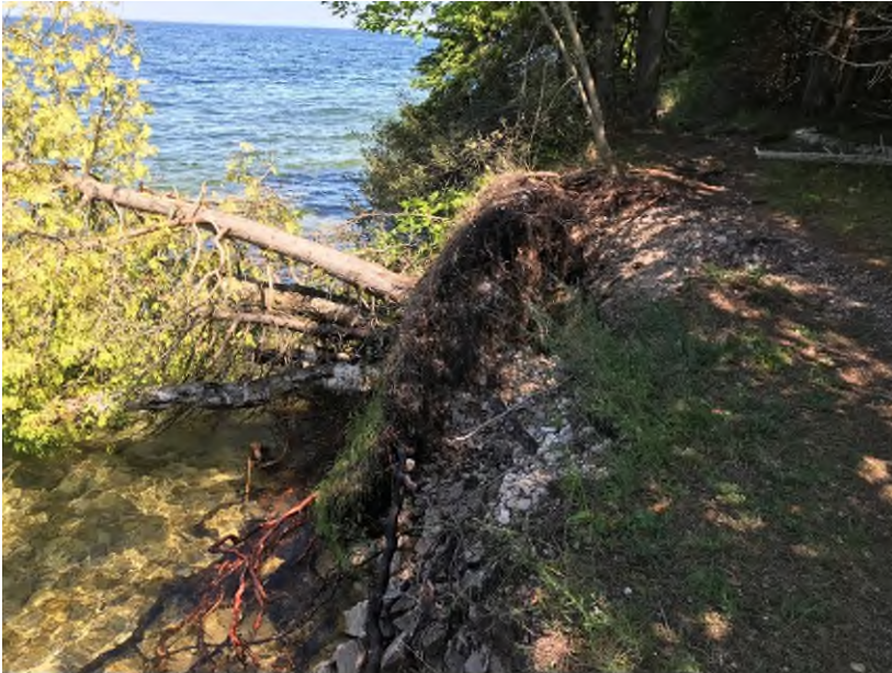
Photo 13. Recent erosion along shoreline Fayette State Park Fairbanks Township T38N R19W Section 5 No proposed designation July 22, 2019
