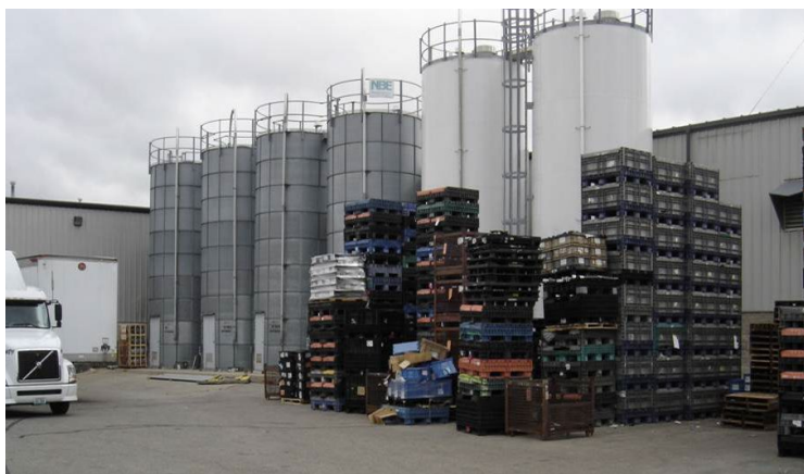
Figure 19 – Good material storage practices at facilities can reduce the potential for spills.
