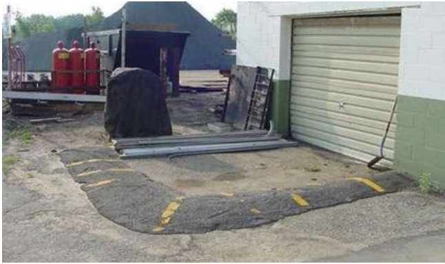
Figure 34 - Curbing is a structural control that can be used to prevent storm water from entering areas where significant materials are stored.
