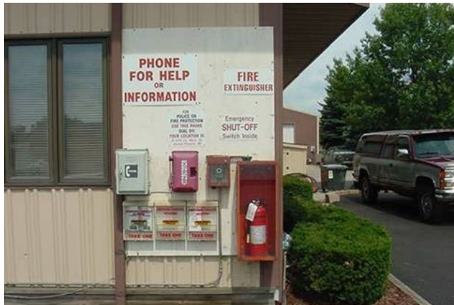
Figure 31 - Signage should be used to convey important information and is considered a necessary structural control in some situations.
