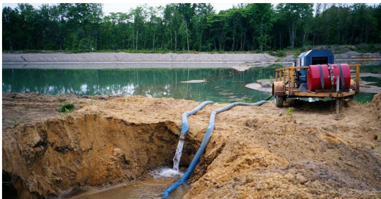
Figure 42 - Mine dewatering water is not authorized under the storm water permit.
