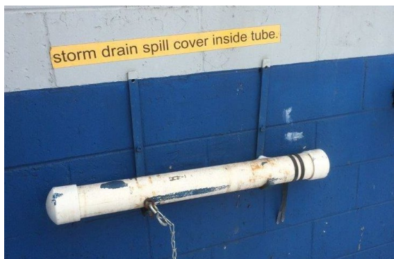
Figure 26 - Signage should be used to identify spill response equipment.
