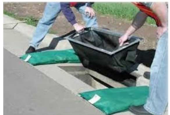
Figure 37 - Catch basin filters can effectively remove sediment from storm water discharges.
