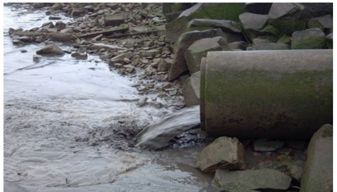
Figure 5 - Outfall to surface waters of the state.
