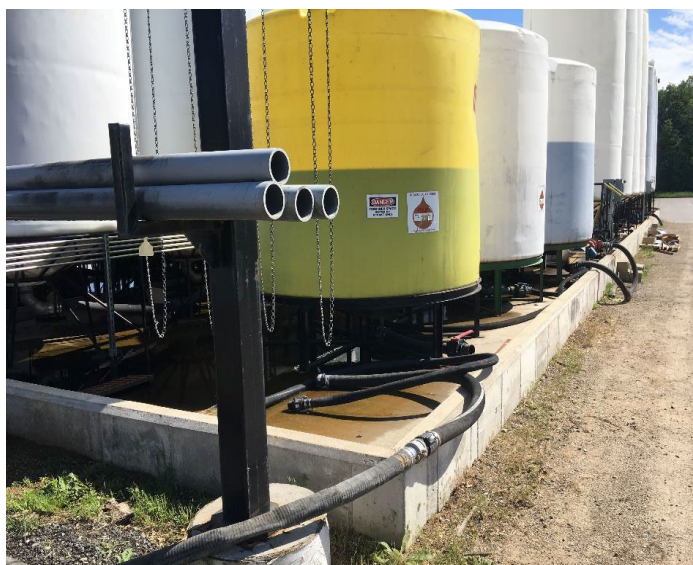
Figure 38 - A STSWCS is required for discharges of storm water to surface waters of the state from regulated secondary containment structures.
