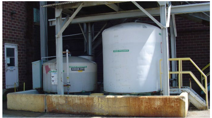
Figure 33 - Secondary containment is intended to protect the environment in the event there is a leak from the storage tanks.
