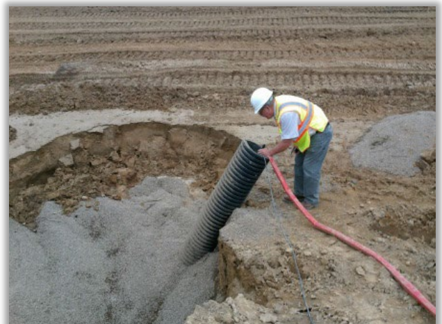
Construction site inspection by a Certified Storm Water Operator
