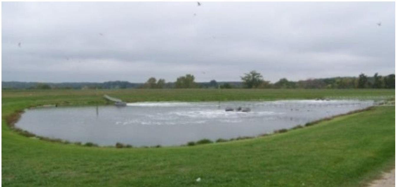
Sanitary Sewage Treatment Lagoon
