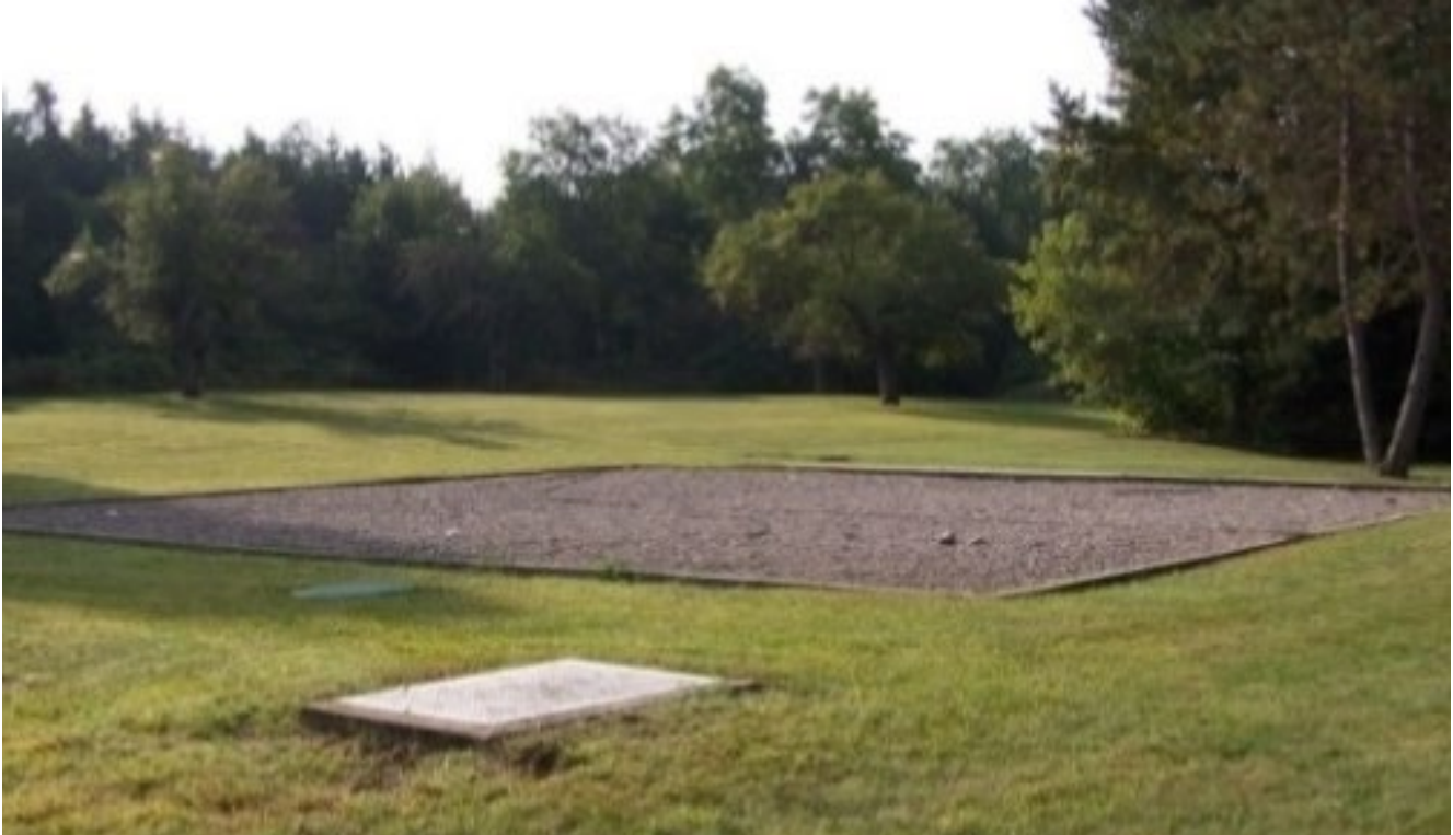
Groundwater Infiltration Bed
