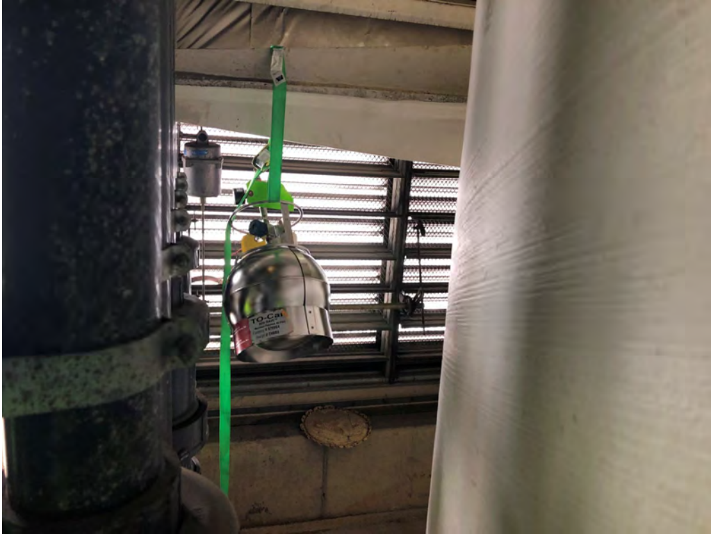
Photo 5: View of sample collection at indoor air (IA) location within scrubber room.
