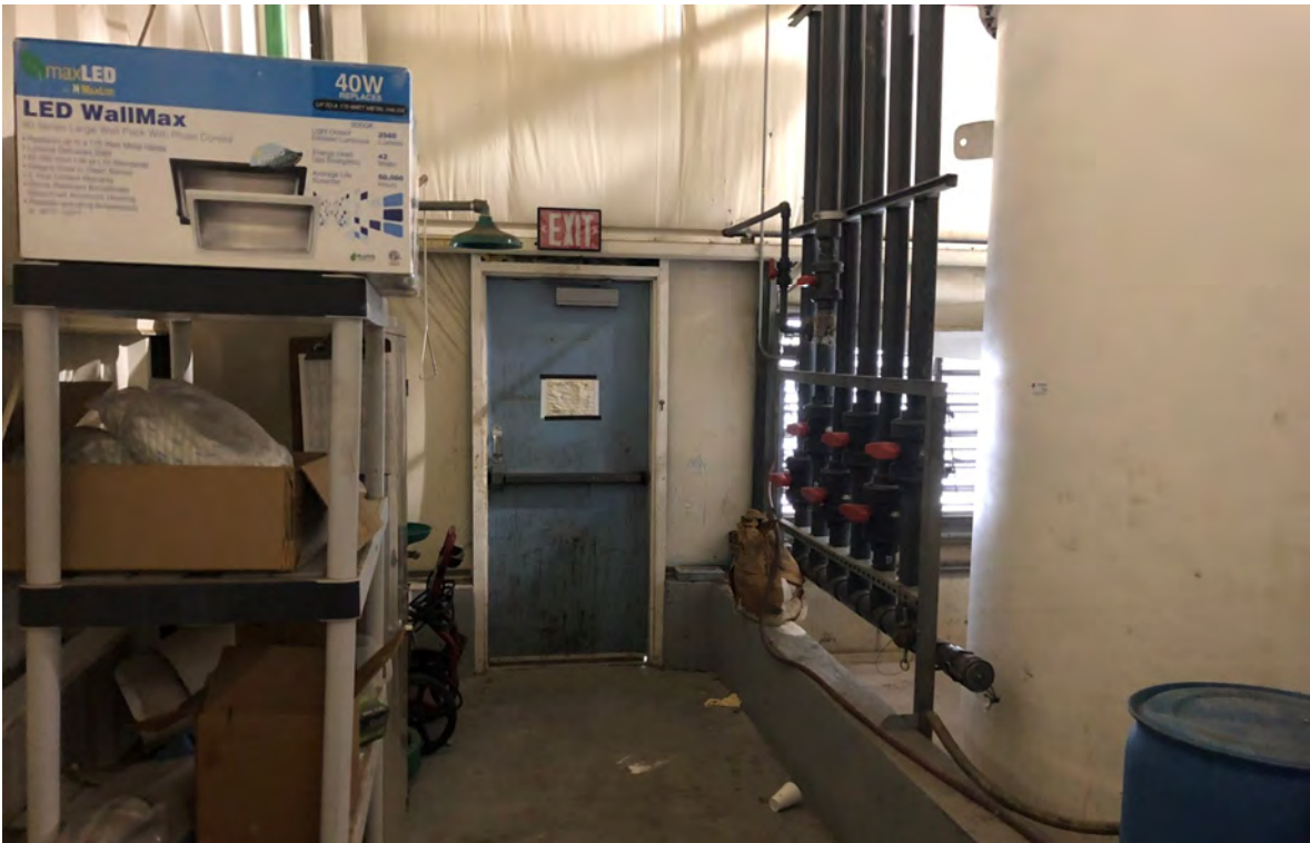
Photo 5: View of northern portion of scrubber room. Sampling area located behind set of vertical pipes on right side of photograph.
