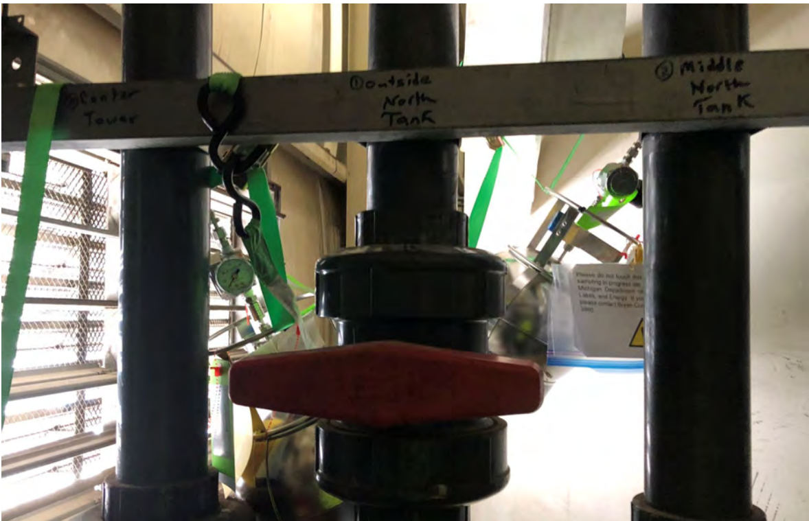
Photo 6: View of sample collection at indoor air (IA) location within scrubber room.
