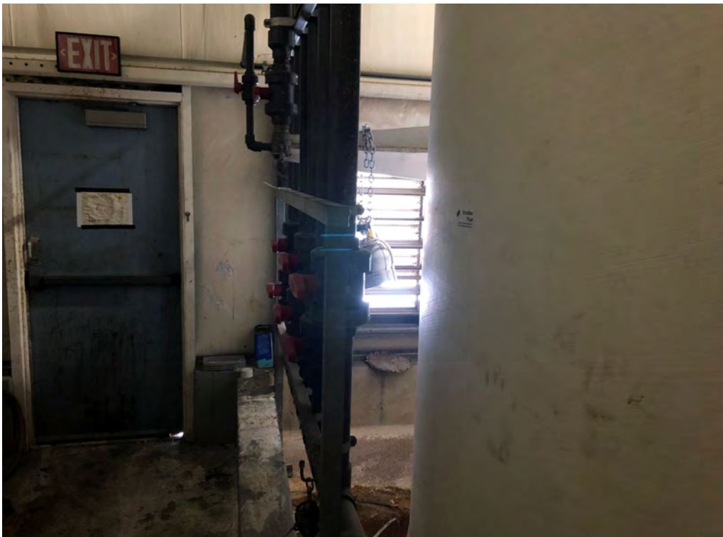
Photo 6: View of sample collection at indoor air (IA) location within scrubber room.
