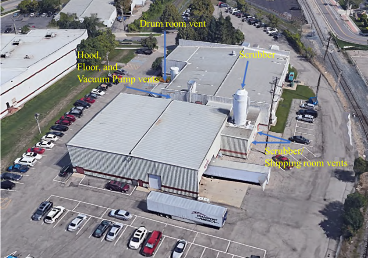
Figure 1: Viant Facility with Fugitive Emission Sources Marked
