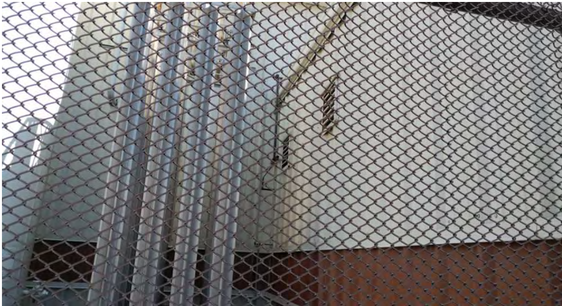
Figure 2 – Drum Room Vents
