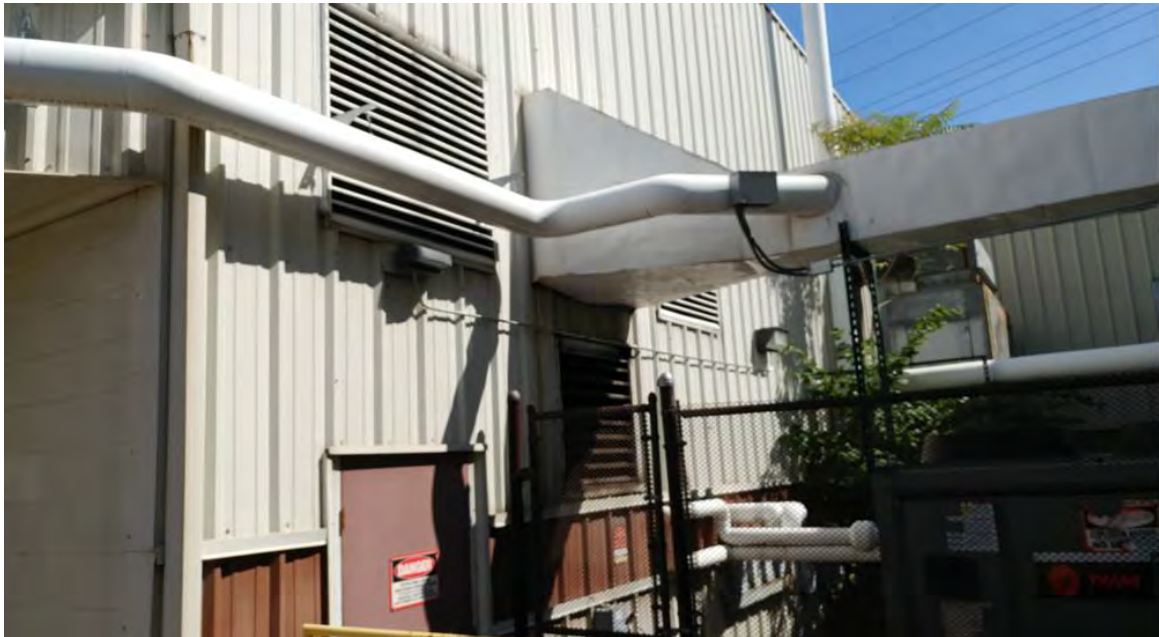
Figure 1 – Hood, Floor, and Vacuum Room Vents
