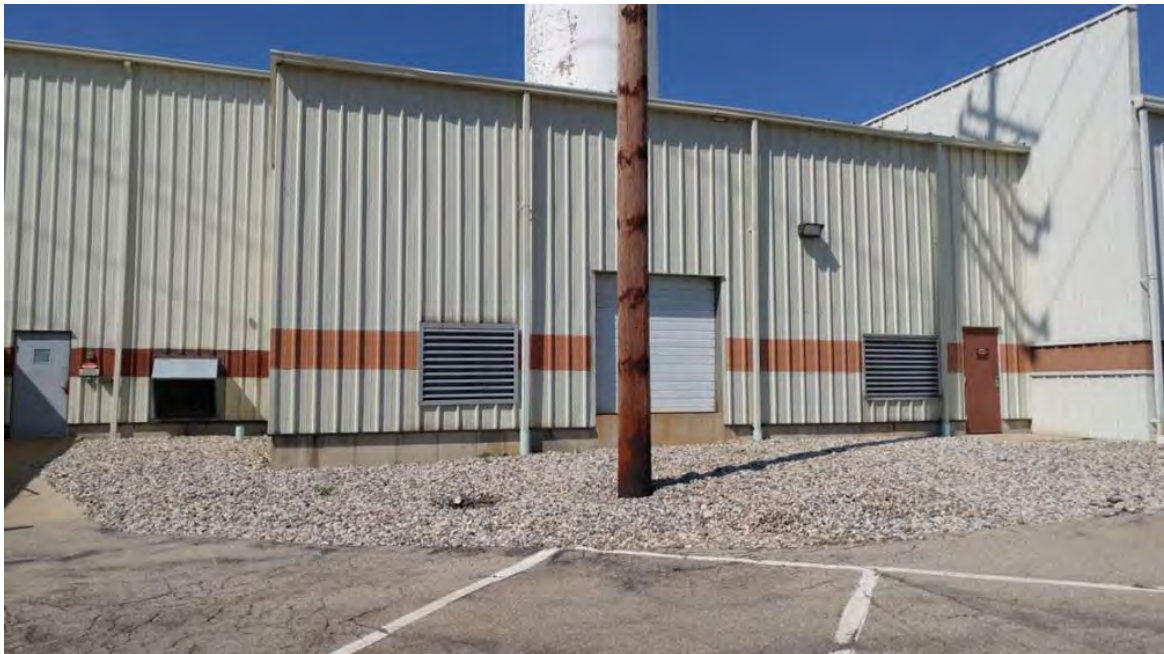
Figure 3 – Shipping Room Vents
