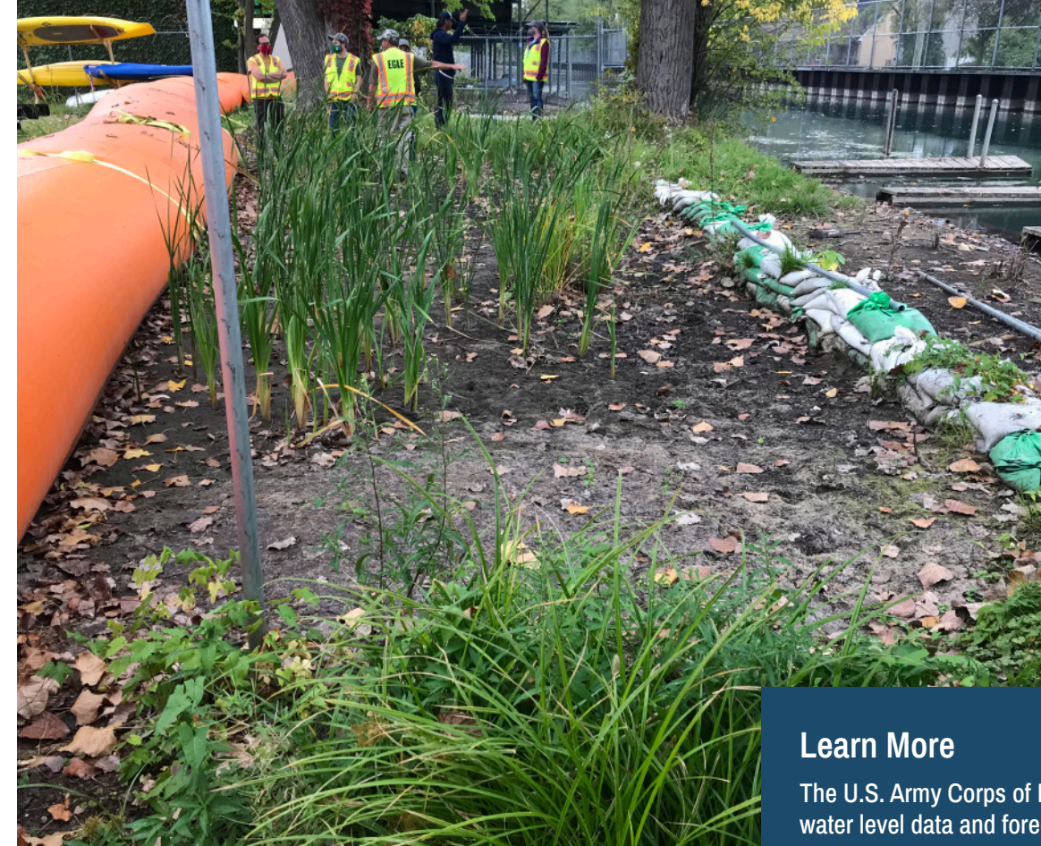
A tiger dam, a tube structure used to hold back water, was installed in Spring 2020 along the canal in the Jefferson-Chalmers area of Detroit next to sandbags that were installed the prior year. (Photo courtesy of EGLE)
