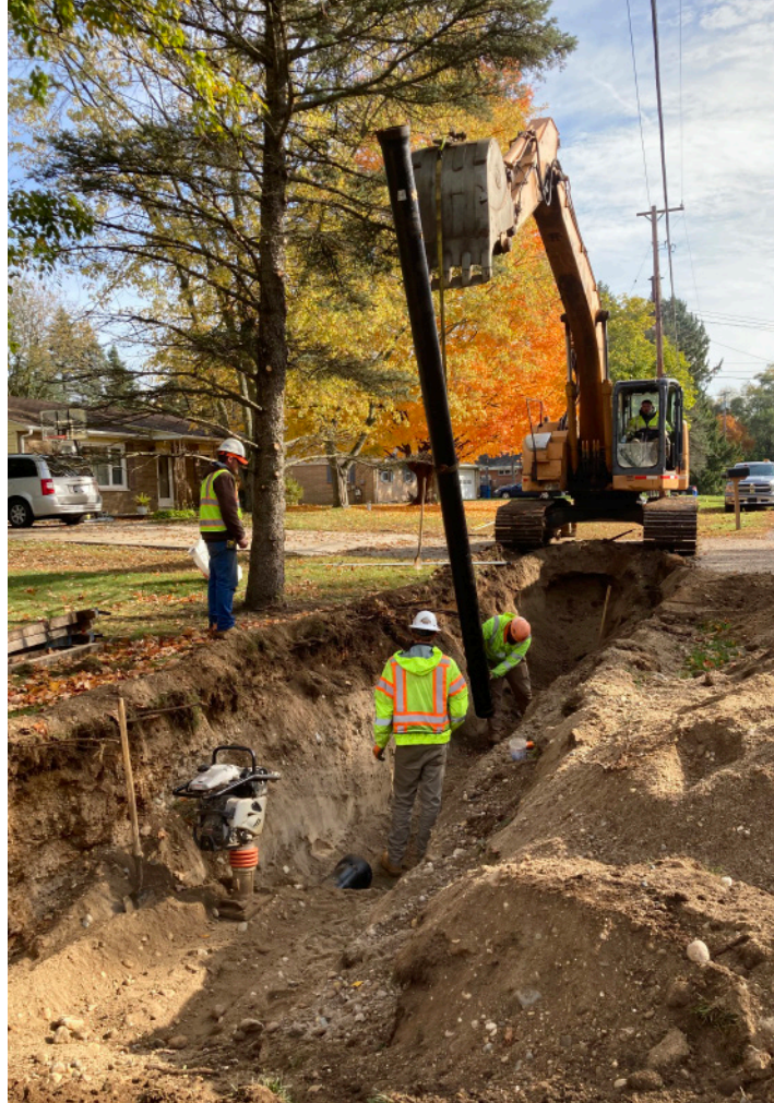
Pipes are replaced in the Kalamazoo area through the Drinking Water State Revolving Fund. (Photo courtesy of Michigan Department of Environment, Great Lakes, and Energy)
