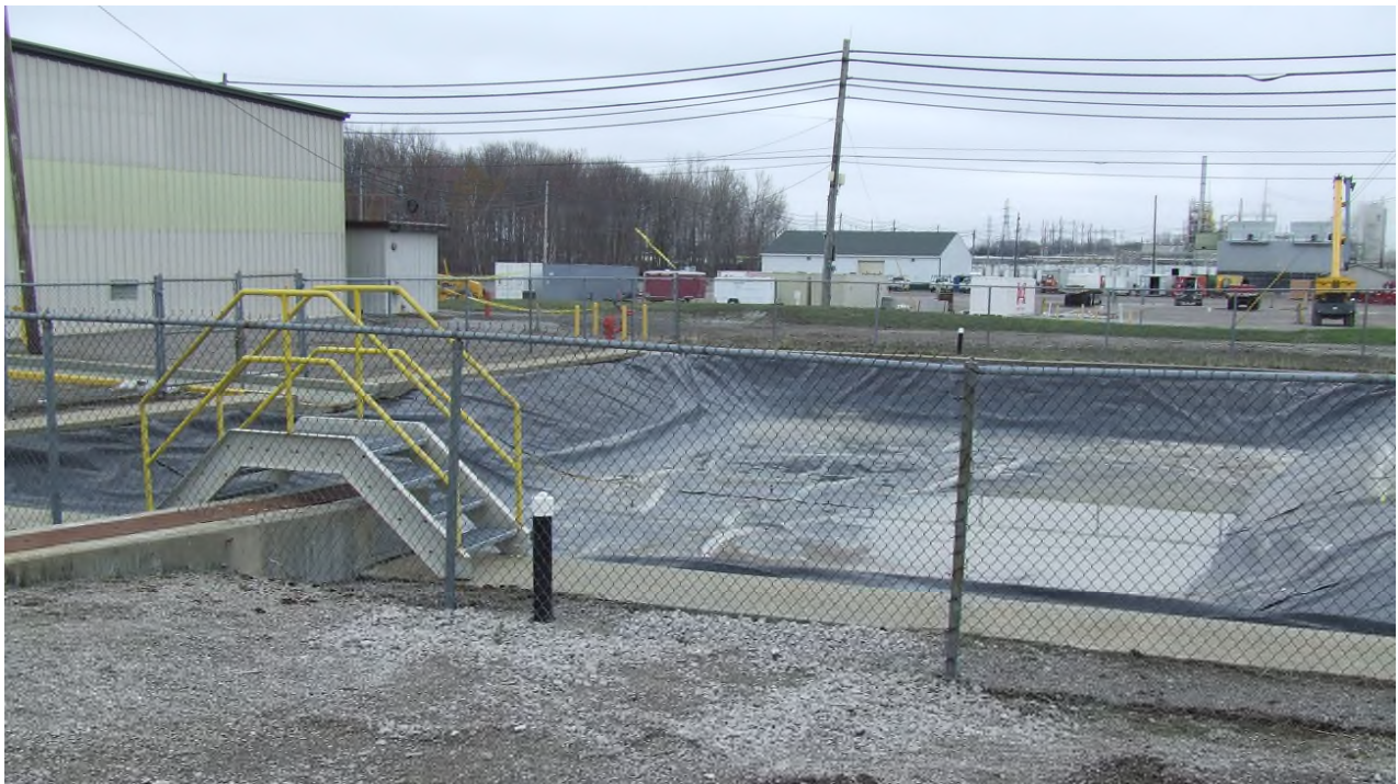
View of secondary containment associated with the hazardous waste storage areas
