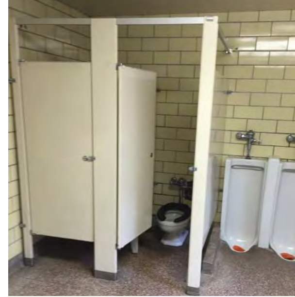
7 Boys Restroom - fixtures too low to meet ADA requirements
