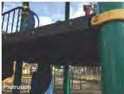
Missing collar pins
