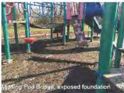
Surfacing: exposed footing
