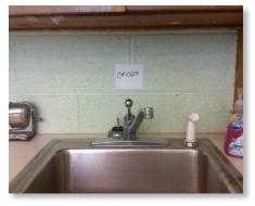
This faucet also has an aerator at the outlet. The aerator should be removed, inspected for particulate accumulations, scrubbed clean, and reinstalled. If particulates are found, the aerator should be periodically checked and cleaned.
