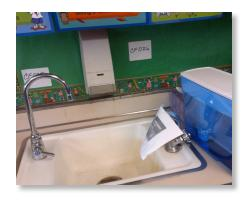
Replacement of this bubbler tap and its connection plumbing with lead-free materials will significantly reduce lead exposure at this location and should be completed. If replacement is not currently feasible, sample results indicate that flushing this tap for 3 minutes prior to each use and for at least 4 minutes following periods of stagnation is likely to reduce lead concentrations and lead exposure. In general, use of this fountain for drinking water should be discouraged.
