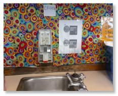
Replacement of this fixture and its connection plumbing with lead-free materials will significantly reduce lead exposure at this location. If replacement is not currently feasible, sample results indicate that flushing this tap for 3 minutes following periods of stagnation is likely to reduce lead concentrations and lead exposure.
