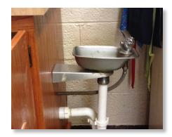
Replacement of this bubbler tap and its connection plumbing with leadfree materials will significantly reduce lead exposure at this location and should be completed. If replacement is not currently feasible, sample results indicate that flushing this tap for 3 minutes following periods of stagnation is likely to reduce lead concentrations and lead exposure.
