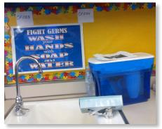
Replacement of this fixture and its connection plumbing with leadfree materials will significantly reduce lead exposure at this location. If replacement is not currently feasible, sample results indicate that flushing this tap for 3 minutes following periods of stagnation is likely to reduce lead concentrations and lead exposure.
