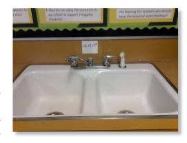
Replacement of this faucet and its connection plumbing with lead free materials will significantly reduce lead exposure at this location. If replacement is not currently feasible, sample results indicate that flushing this tap for 3 minutes following periods of stagnation is likely to reduce lead concentrations and lead exposure.
