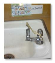
Replacement of this bubbler tap and its connection plumbing with lead free materials will significantly reduce lead exposure at this location. If replacement is not currently feasible, sample results indicate that flushing this tap for 3 minutes following periods of stagnation is likely to reduce lead concentrations and lead exposure.
