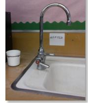
Replacement of this faucet and its connection plumbing with lead free materials will significantly reduce lead exposure at this location. If replacement is not currently feasible, sample results indicate that flushing this tap for 3 minutes following periods of stagnation is likely to reduce lead concentrations and lead exposure.
