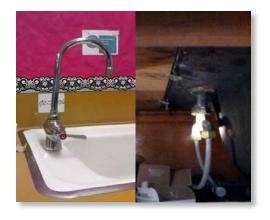
Replacement of this faucet and its connection plumbing with lead free materials will significantly reduce lead exposure at this location. If replacement is not currently feasible, sample results indicate that flushing this tap for 3 minutes following periods of stagnation is likely to reduce lead concentrations and lead exposure.
