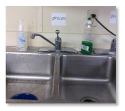
Replacement of this faucet and its connection plumbing with lead free materials will significantly reduce lead exposure at this location. If replacement is not currently feasible, sample results indicate that flushing this tap for 3 minutes following periods of stagnation is likely to reduce lead concentrations and lead exposure.
