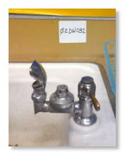
Replacement of this bubbler tap and its connection plumbing with lead free materials will significantly reduce lead exposure at this location. If replacement is not currently feasible, sample results indicate that flushing this tap for 3 minutes following periods of stagnation is likely to reduce lead concentrations and lead exposure.
