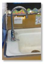
Replacement of this faucet and its connection plumbing with lead free materials will significantly reduce lead exposure at this location. If replacement is not currently feasible, sample results indicate that flushing this tap for 3 minutes following periods of stagnation is likely to reduce lead concentrations and lead exposure.
