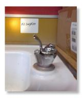
Replacement of this bubbler tap and its connection plumbing with lead free materials will significantly reduce lead exposure at this location. If replacement is not currently feasible, sample results indicate that flushing this tap for 3 minutes following periods of stagnation is likely to reduce lead concentrations and lead exposure.
