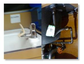
Replacement of this bubbler tap and its connection plumbing with lead free materials will significantly reduce lead exposure at this location. If replacement is not currently feasible, sample results indicate that flushing this tap for 3 minutes following periods of stagnation is likely to reduce lead concentrations and lead exposure.
