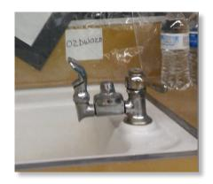
Replacement of this bubbler tap and its connection plumbing with lead-free materials will significantly reduce lead exposure at this location. If replacement is not currently feasible, sample results indicate that flushing this tap for 3 minutes following periods of stagnation is likely to reduce lead concentrations and lead exposure.
