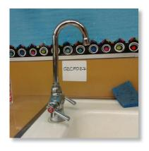
Replacement of this faucet and its connection plumbing with lead free materials will significantly reduce lead exposure at this location. If replacement is not currently feasible, sample results indicate that flushing this tap for 3 minutes following periods of stagnation is likely to reduce lead concentrations and lead exposure.
