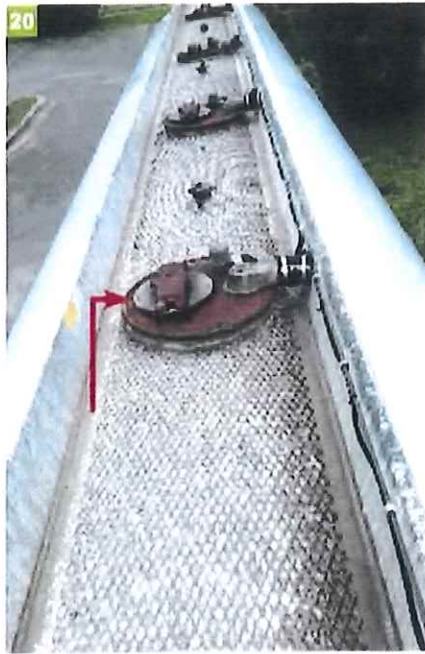
(20) On the manhole, clockwise from left (arrow) are the dome hatch, the Scully device, and the vapor valve.
