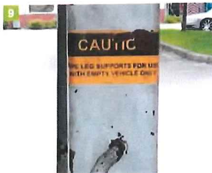
(8) The warning label (arrow) area on this pin-type leg support landing gear is completely faded. (9) This may be the only warning you will get to prevent a catastrophe. Many legs are not marked.
