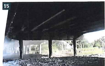
(14) Tanker crash and fire on I-75/U.S. 301 in Ellenton, Florida, in 2008. During this fire, the spilled fuel was allowed to completely burn itself out. [Photos 14 and 15 courtesy of North River (FL) Fire District.] (15) Tanker crash and fire on I-75/U.S. 301 in Ellenton, Florida, in 2008. Note the massive amount of concrete spalling. This overpass is a total loss and the months it took to replace it caused a major transportation crisis in the region. However, no amount of resources could have saved this bridge.
