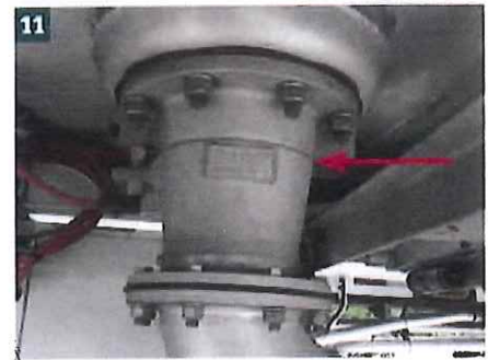
(10) Note the shear point of this cable-operated belly valve housing (arrow). (Photo by author.)
