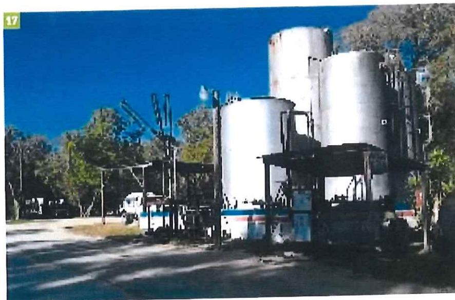
(17) A top-loading fuel dock and tanks.
