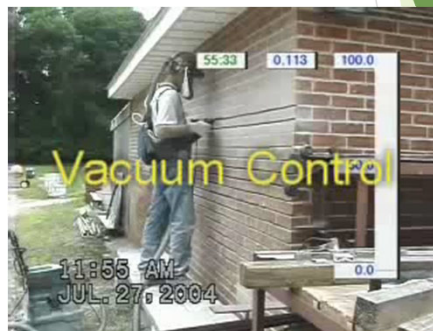
Local ventilation control
