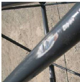
Deformed, cracked, or significantly corroded structural members.
