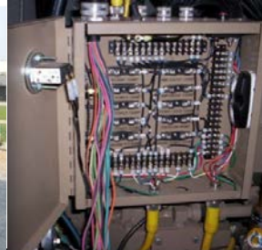
Electrical components and wiring for cracked or split insulation and loose or corroded Terminations.
