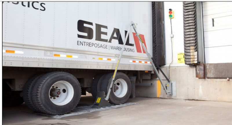
Wheel chock and dock lock light system in use
