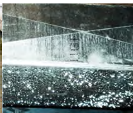
DUCT CONDENSATION
