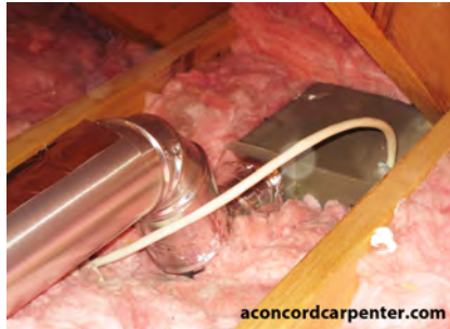
Right-way fan orientation: Air stream turns 2 90-degree angles, which is acceptable.
