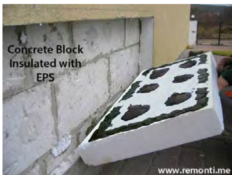
EPS foundation insulation: Installers glue masonry-faced EPS-foam sheets to the block wall.
