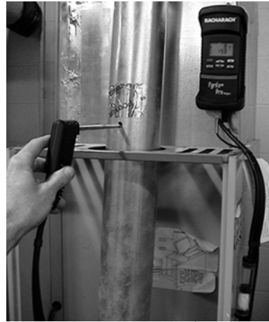
80+ Furnace: Measure draft and sample flue gases in the vent connector above the furnace. Only a licensed heating technician — and not an energy auditor — can perform this test.
