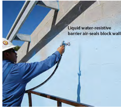
Liquid water-resistant barrier: This retrofit serves two purposes: water proofing and air sealing.
