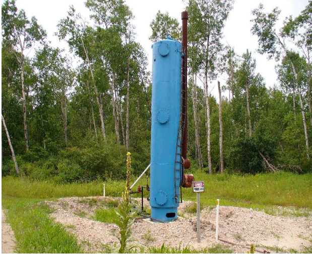
Figure 2: Easily accessible oil field equipment at the West Branch oil fields, Ogemaw County, Michigan.
