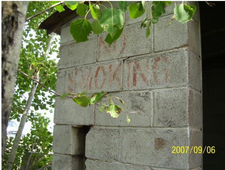
Figure 6. Possible underground storage tank at former Quincy reclamation plant in Mason (Houghton County), Michigan. (Picture taken September 6, 2007. Source: Weston 2007.)
