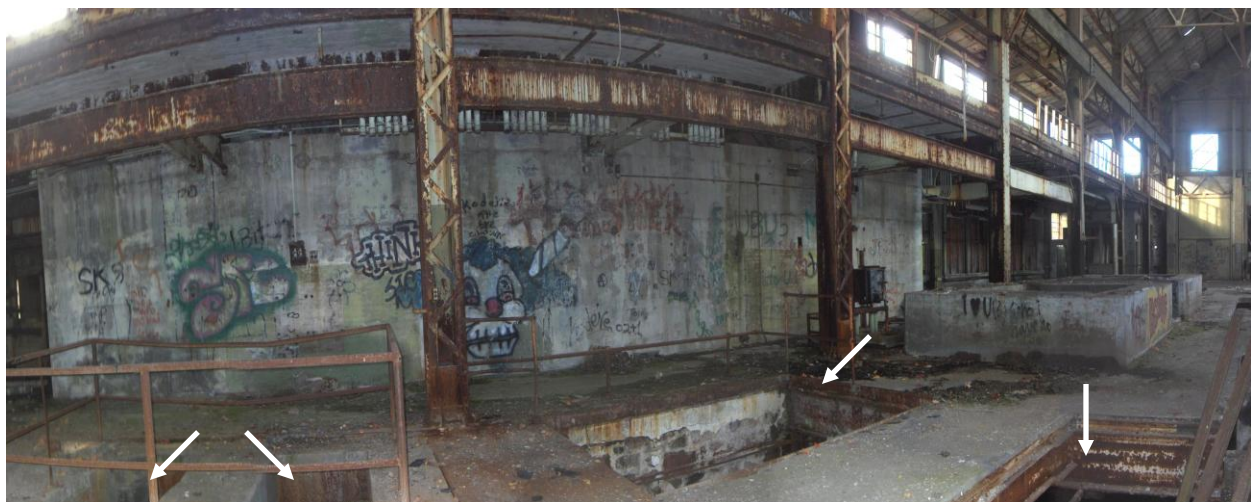
Figure 23. Interior of former Calumet and Hecla Power Plant showing graffiti and floor pits (white arrows), Lake Linden (Houghton County), Michigan. (Photo date unknown. Source: MDNRE.)
