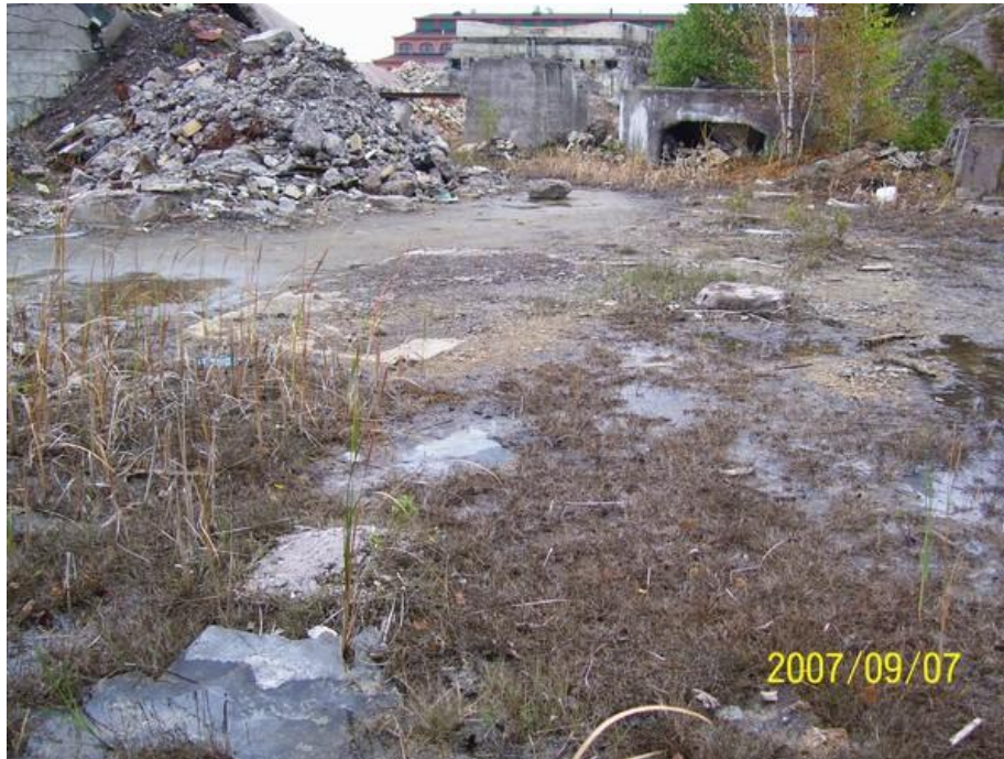
Figure 22. Debris at Mineral Building in Hubbell (Houghton County), Michigan. (Picture taken September 7, 2007. Source: Weston 2007.)
