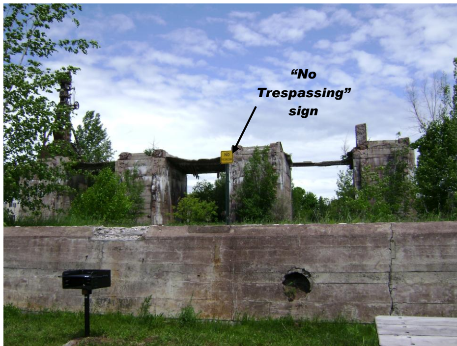
Figure 16. Wall with “No Trespassing” sign separating playground/picnic area from former Ahmeek stamping mill ruins in Tamarack City/Hubbell (Houghton County), Michigan. (Picture taken June 16, 2008. Source: MDCH.)
