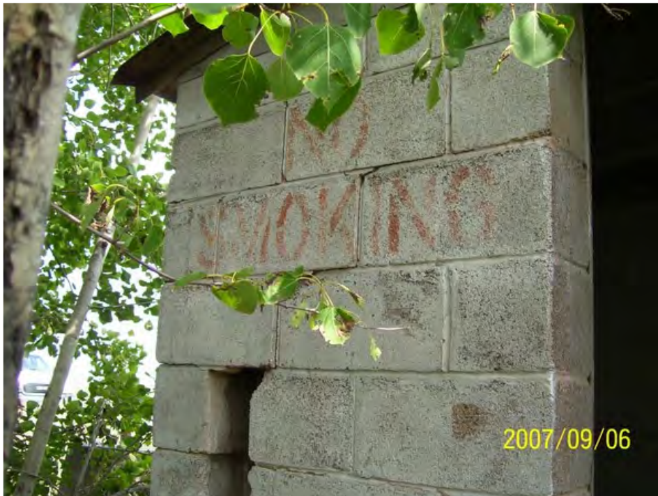
Figure 6. Possible underground storage tank at former Quincy reclamation plant in Mason (Houghton County), Michigan. (Picture taken September 6, 2007. Source: Weston 2007.)
