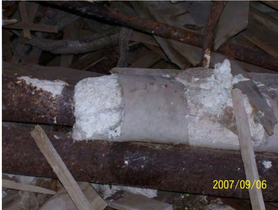
Figure 12. Suspected asbestos-containing material at “Building in Mason,” west of former Quincy Reclamation Plant area (across M-26) in Mason (Houghton County), Michigan. (Picture taken September 6, 2007. Source: Weston2007.)
