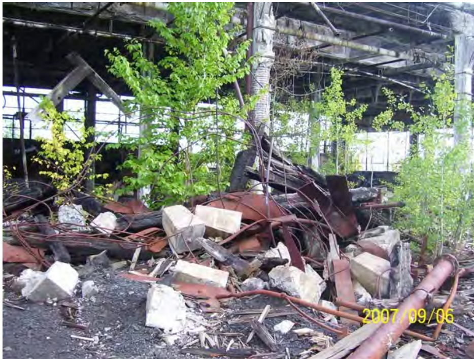
Figure 11. Debris at “Building in Mason,” west of former Quincy Reclamation Plant area (across M-26) in Mason (Houghton County), Michigan. (Picture taken September 6, 2007. Source: Weston 2007.)
