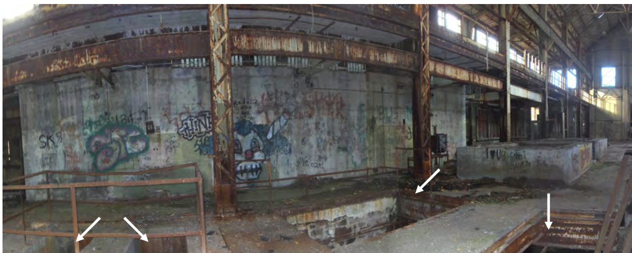
Figure 23. Interior of former Calumet and Hecla Power Plant showing graffiti and floor pits (white arrows), Lake Linden (Houghton County), Michigan. (Photo date unknown. Source: MDEQ.)
