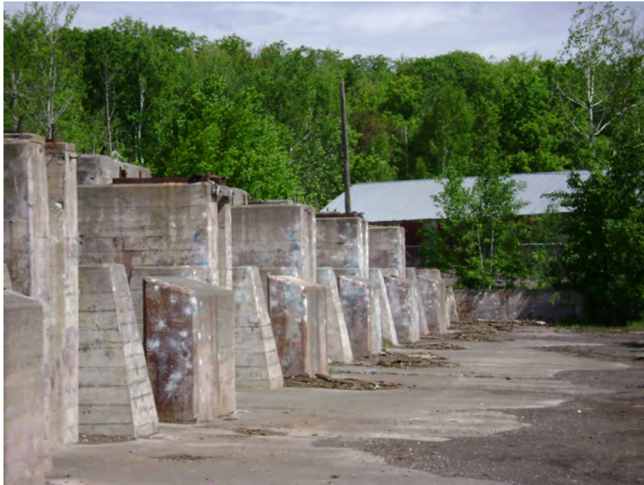
Figure 5. Closer view, with evidence of paintball splatters, of ruins of Quincy reclamation plant in Mason (Houghton County), Michigan. (Picture taken June 16, 2008. Source: MDCH.)
