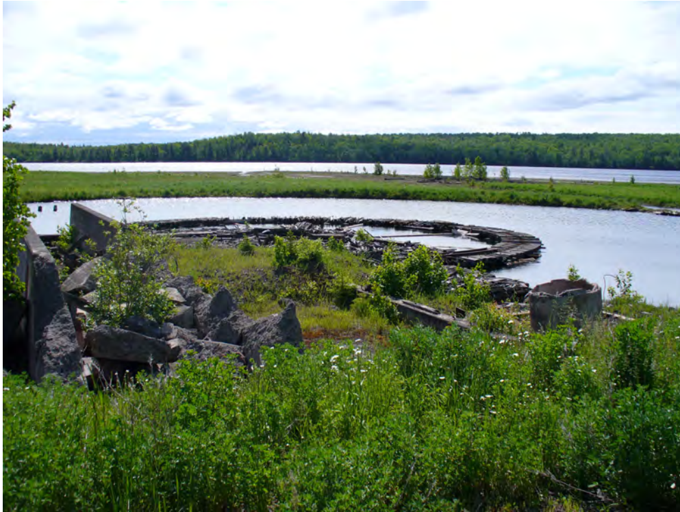
Figure 7. Circular track offshore in Torch Lake at former Quincy reclamation plant in Mason (Houghton County), Michigan. (Picture taken June 16, 2008. Source: MDCH.)
