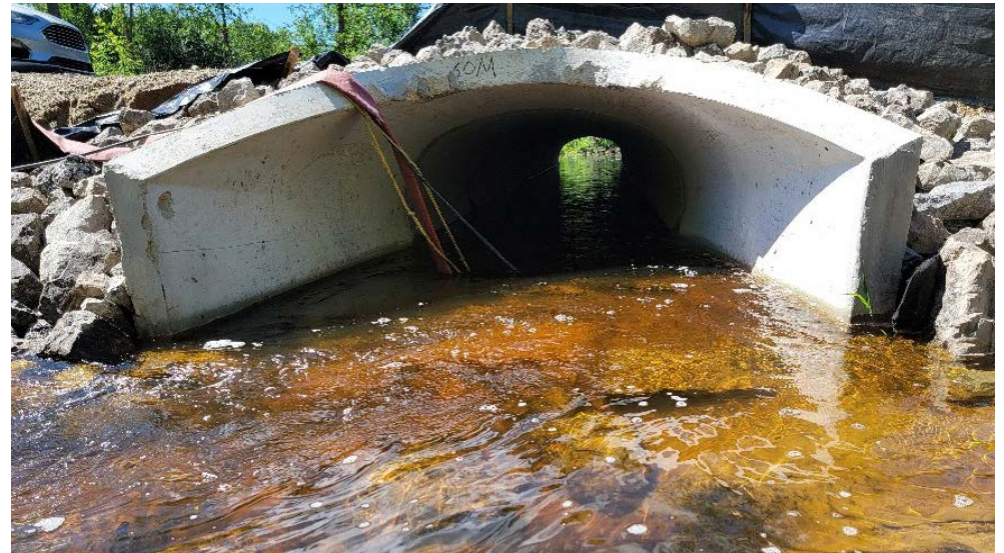
Culvert replacement during construction
