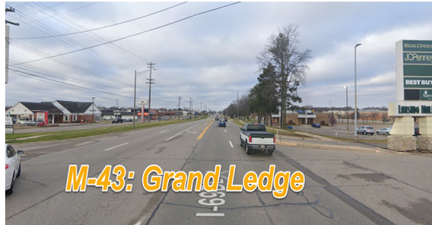
Figure 4.5. Street View Photographs of Pilot Sites
