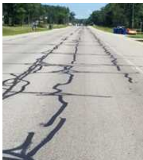
MODERATE CRACK DENSITY 250 LINEAR FEET OF CRACKING
