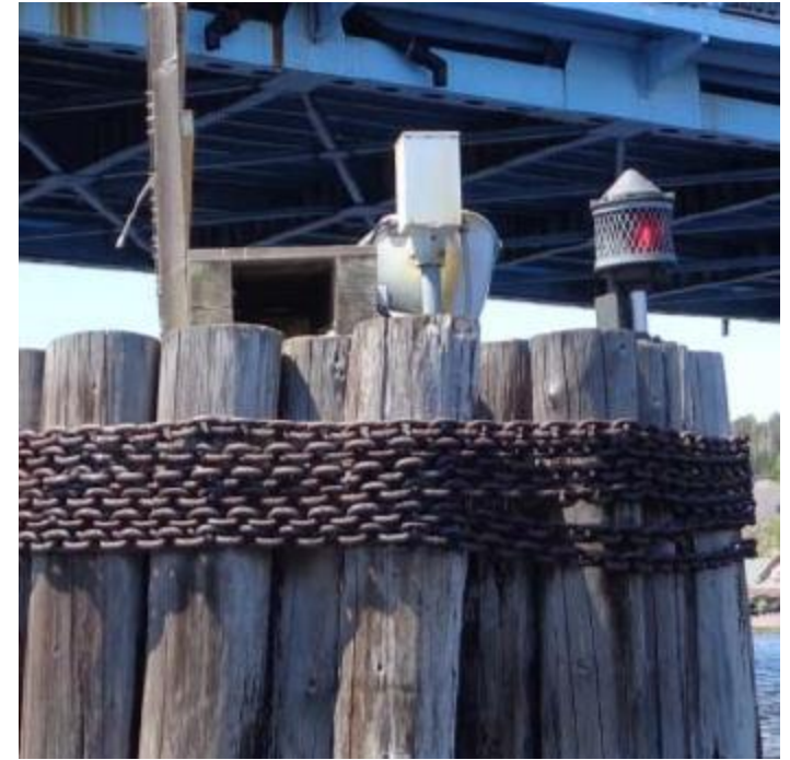
Pier Pile Cluster
