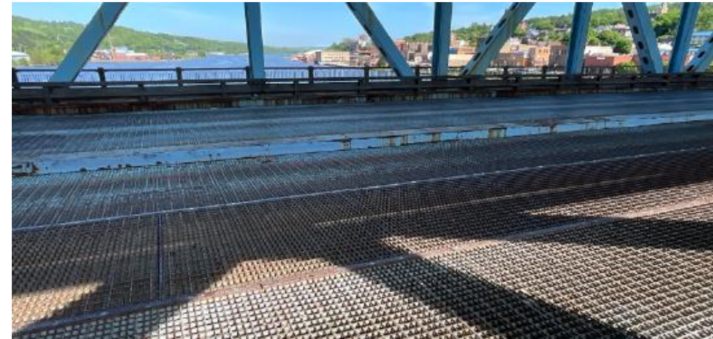
View of Lower Grid Deck
