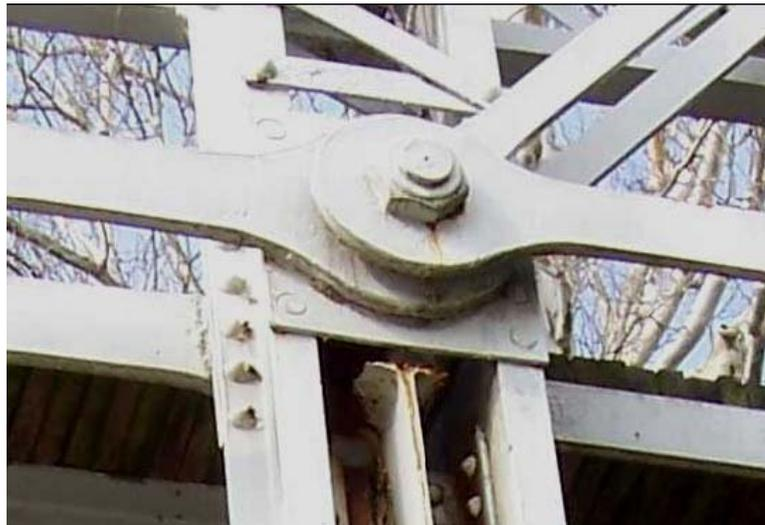
Figure 3: Pinned Truss Connection
