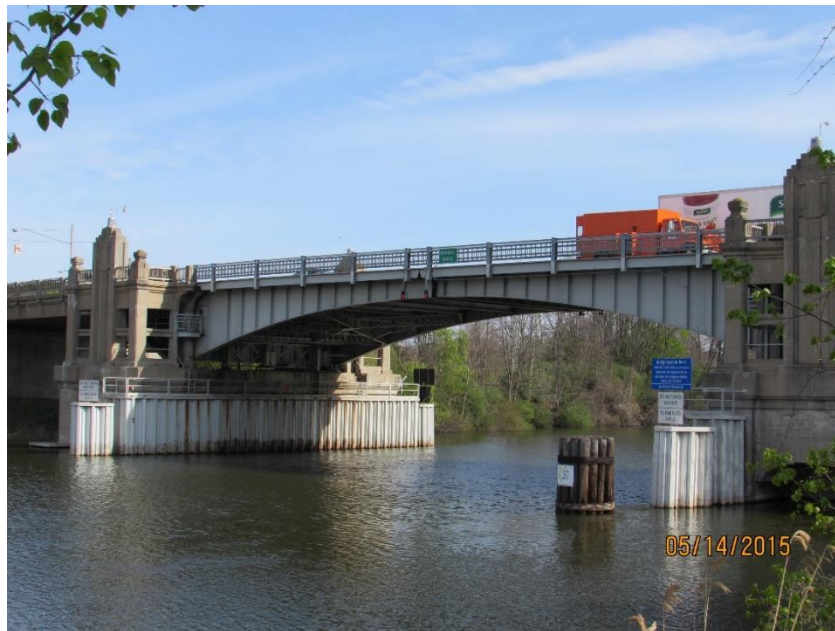
Figure B.03.01 Movable span of Manistee Bascule Bridge
