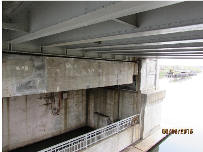
Figure B.03.05 Fracture Critical Steel Cross Girder
