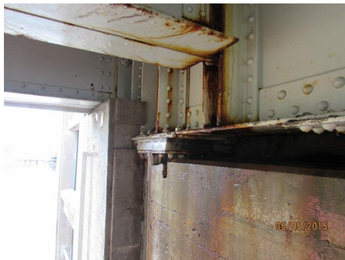
Figure B.03.06 Live Load Shoe/Uplift Bearings
