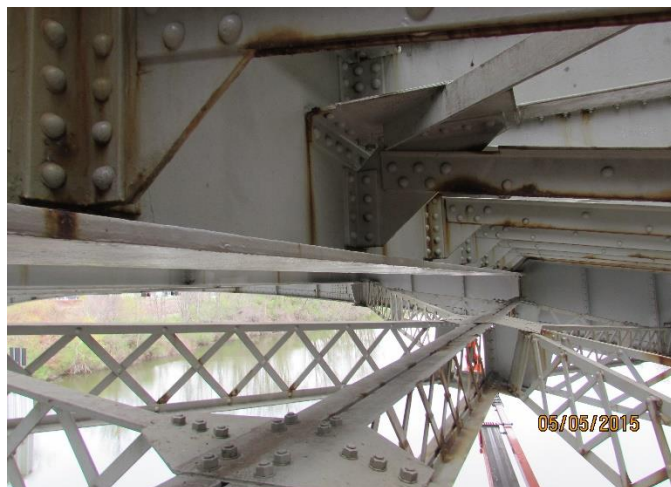
Figure B.03.04 Fracture Critical Floorbeams
