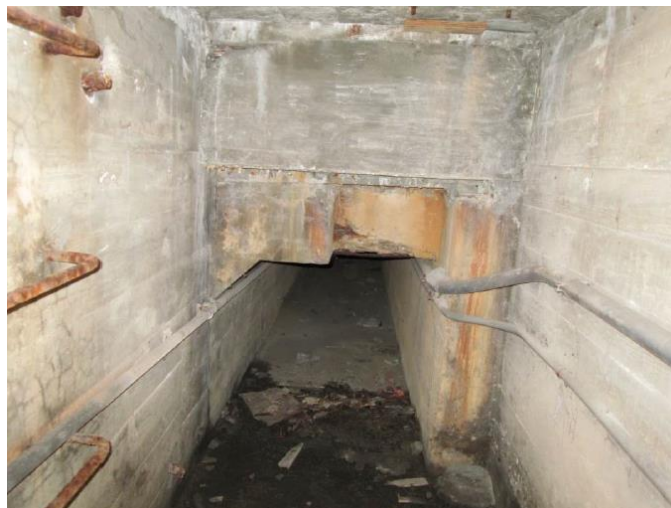
Figure B.03.12 Vaulted Abutments
