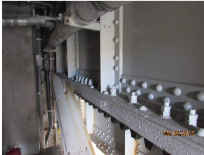
Figure B.03.07 Rack and Frame Support
