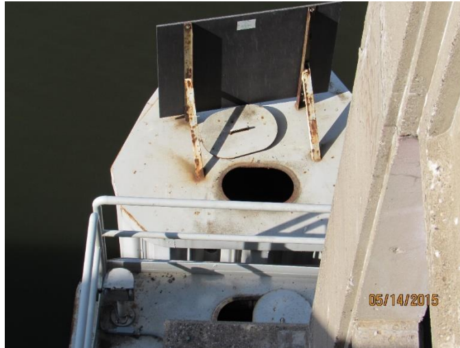
Figure B.03.11 Pile Cluster Interior
