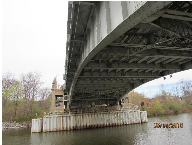
Figure B.03.03 Fracture Critical Primary Girders
