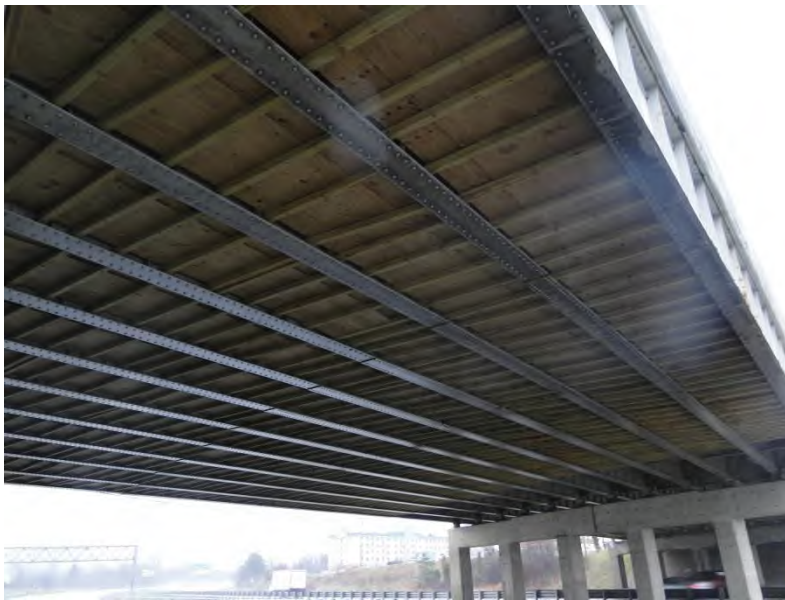
Figure 5.10.04 Structure Where Plywood False Decking Coverage Requires In-Depth Inspection
