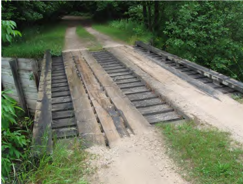
Figure 5.05.06 Timber Running Planks Protecting Timber Deck
