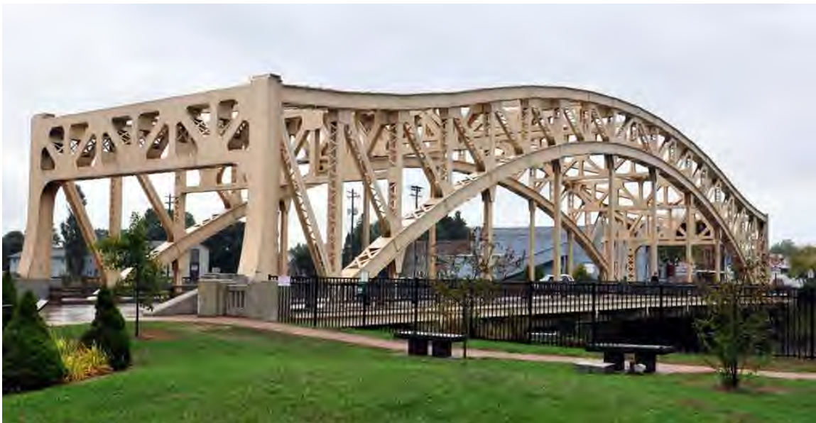
Figure 5.13.16 Steel Through Arch with Fracture Critical Floor Beams and Suspension Hangers
