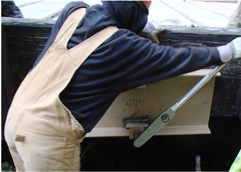
Figure 5.11.05 Post Tensioning Glulam Deck Panels
