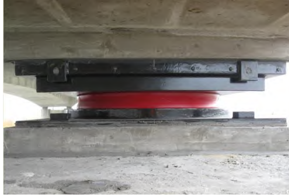
Figure 5.16.07 Disk Bearing
