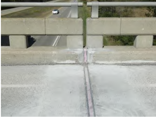
Figure 5.08.07 Parapet Railing Item 36A = 0
