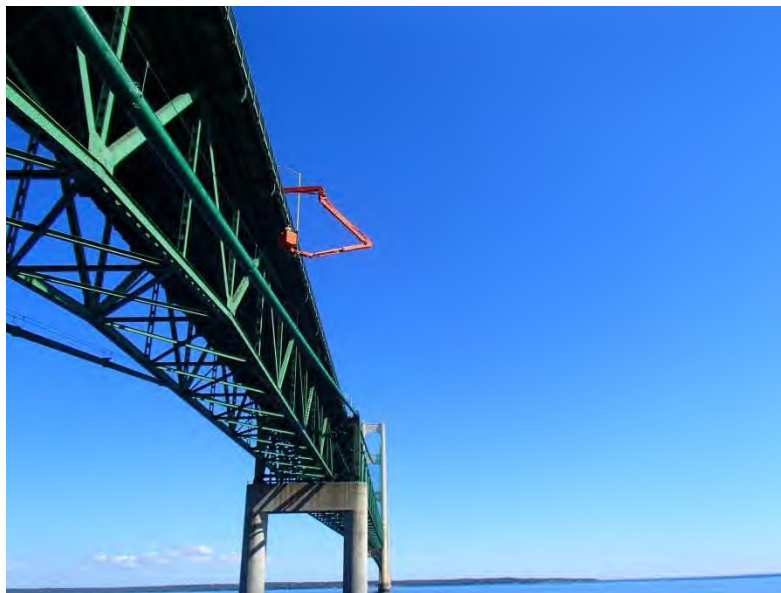
Figure 5.02.01 Utilization of an Under-Bridge Inspection Unit during Routine Inspection
