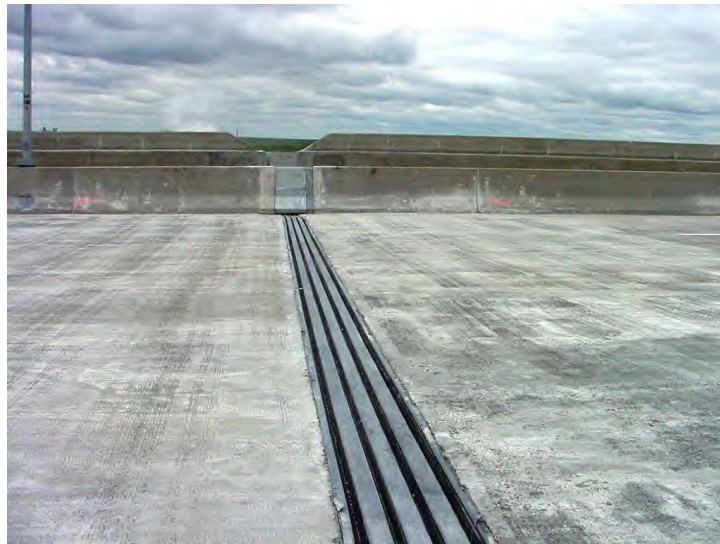
Figure 5.06.05 Assembly Joint with Seal
