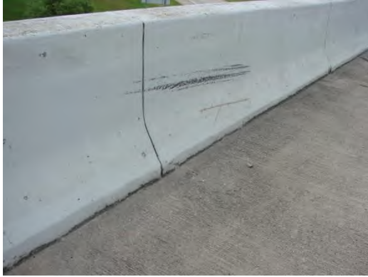
Figure 5.08.01 Type 5 Railing Item 36A = 1
