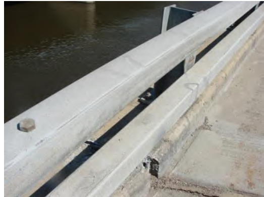
Figure 5.08.04 Two Tube Railing Item 36A = 1
