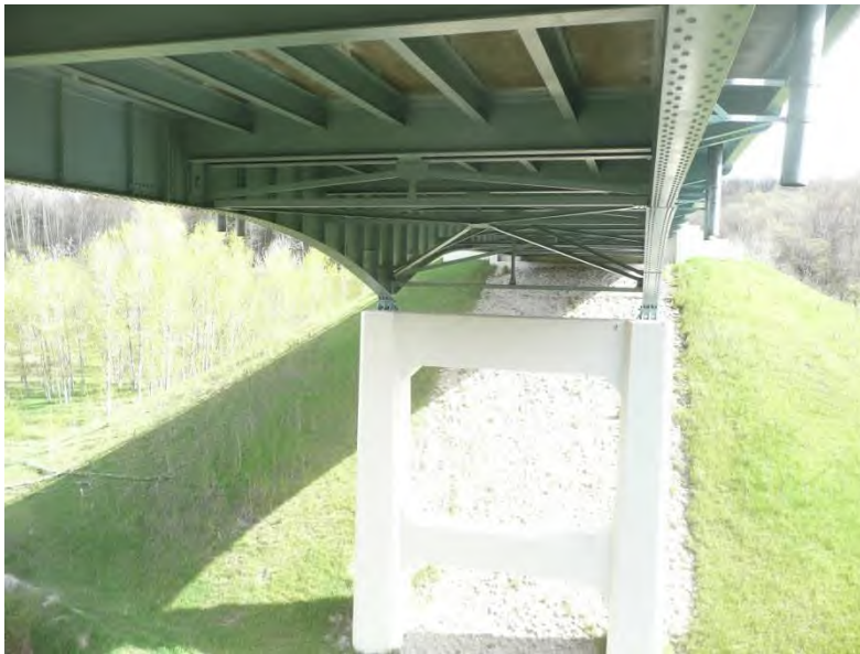
Figure 5.18.01 Two Column Pier Supporting Fracture Critical Structure
