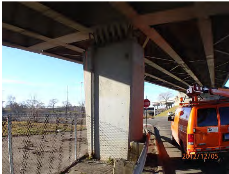
Figure 5.18.02 Element 234 Reinforced Concrete Column
