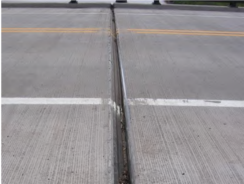
Figure 5.06.02 Full Depth Strip Seal
