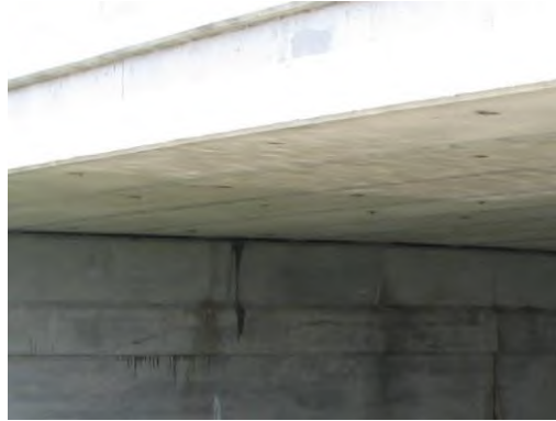
Figure 5.16.04 Enclosed/Concealed Bearing
