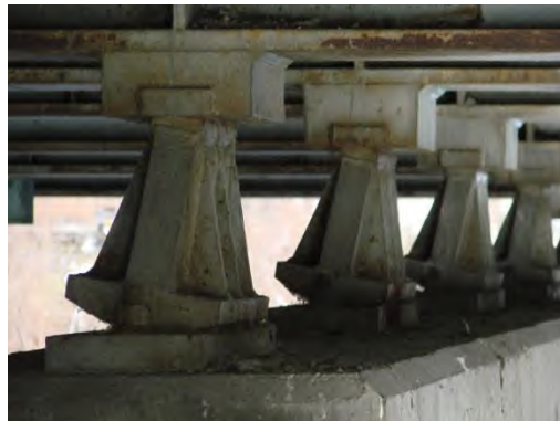
Figure 5.16.03 Movable Bearing
