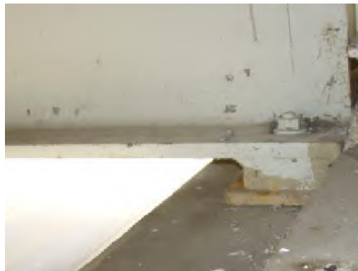
Figure 5.16.05 Fixed Bearing
