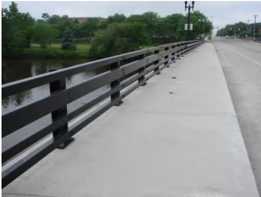
Figure 5.08.03 Four Tube Bicycle Railing Item 36A = 1
