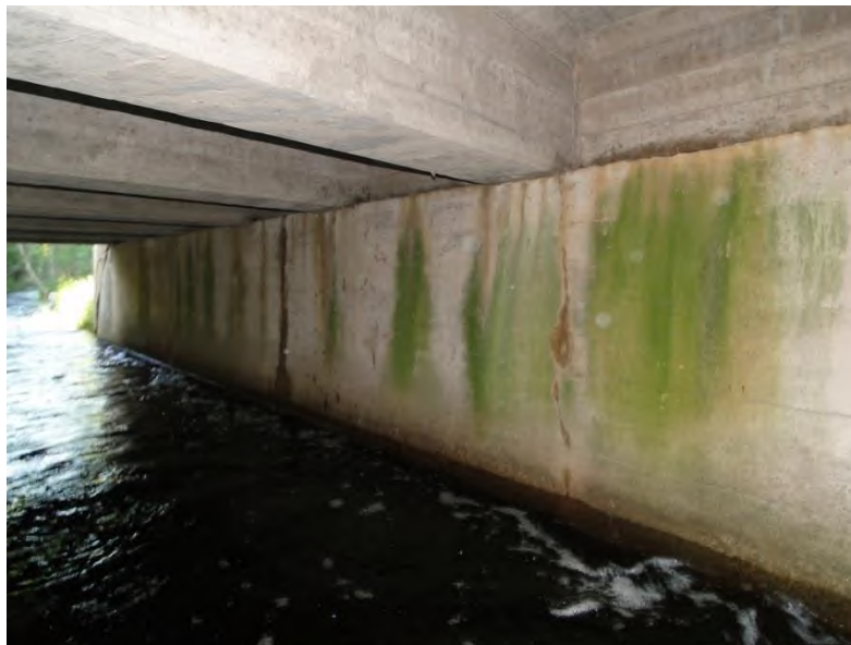
Figure 5.13.01 Uniform Depth Concrete Tee Beams
