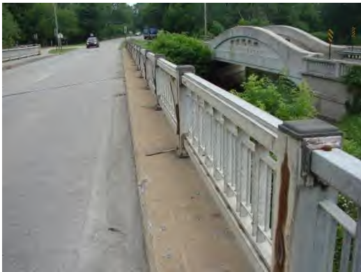
Figure 5.08.09 R4 Railing Item 36A = 0
