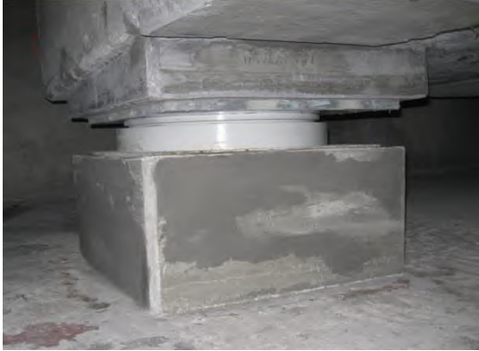
Figure 5.16.06 Pot Bearing
