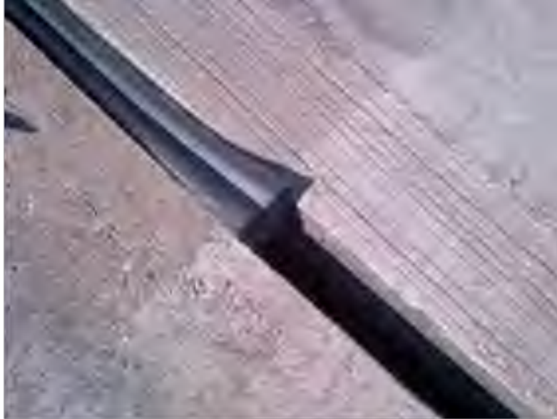
Figure 5.06.04 Compression Joint Seal
