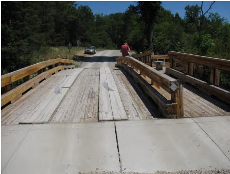
Figure 5.09.05 Designated Pedestrian Walkway on Nail Laminated Deck
