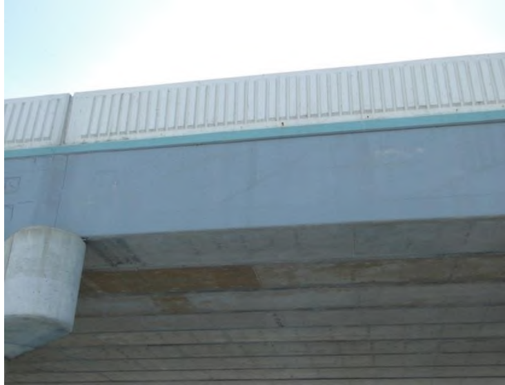
Figure 5.13.03 Concrete Surface Coating on Side-by-Side Box Beams
