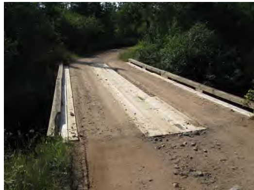
Figure 5.08.10 Timber Brush Block Item 36A = N
