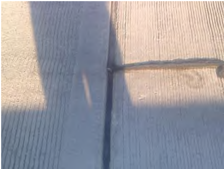
Figure 5.06.03 Pourable Joint Seal
