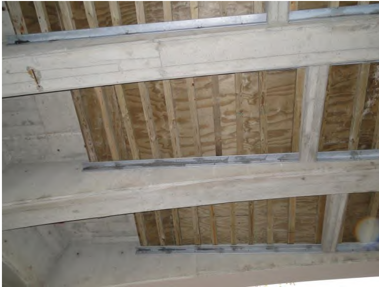
Figure 5.10.01 Tee Beam Superstructure with Plywood False Decking
