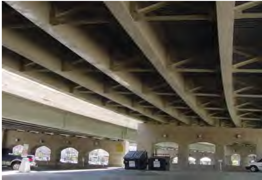
Figure 5.13.09 Curved Steel Plate Girders with Primary Cross Frame Diaphragms
