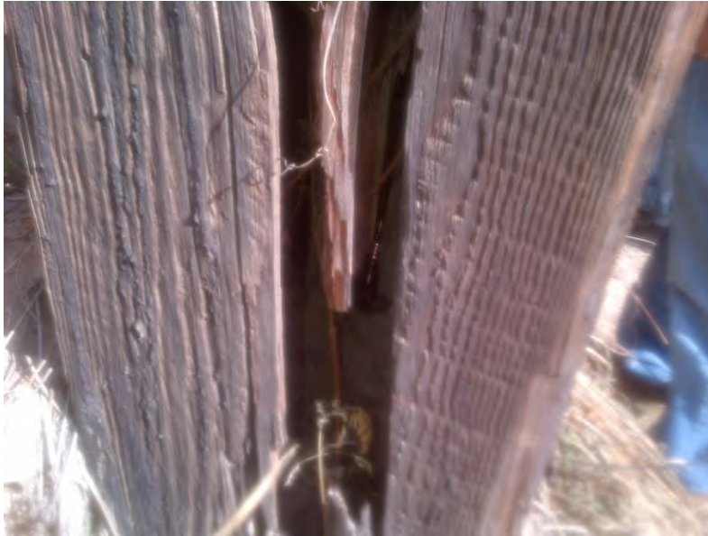
Figure 5.18.05 Hollow Timber Column
