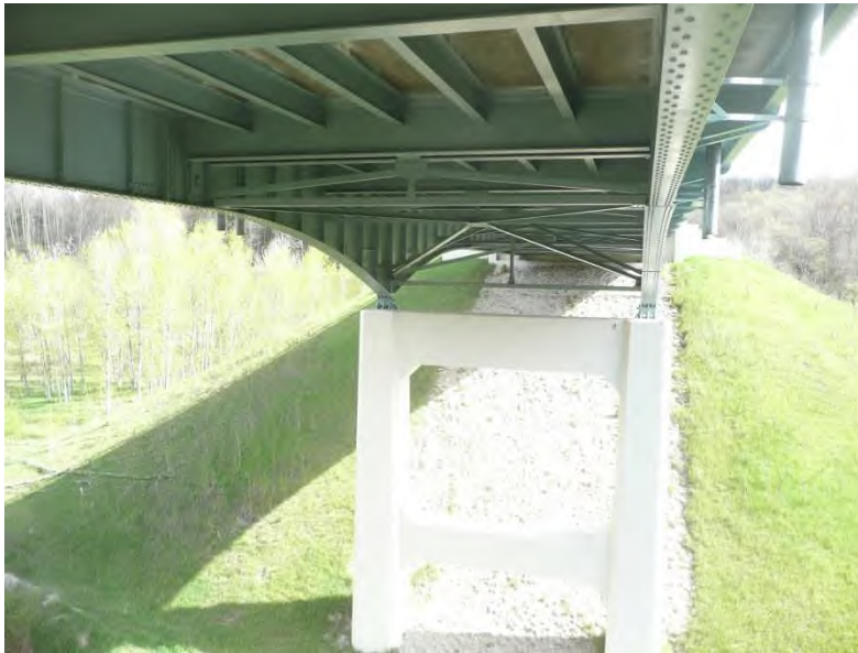
Figure 5.13.11 Non-Redundant Fracture Critical Two Girder Superstructure System
