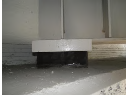
Figure 5.16.02 Elastomeric Bearing
