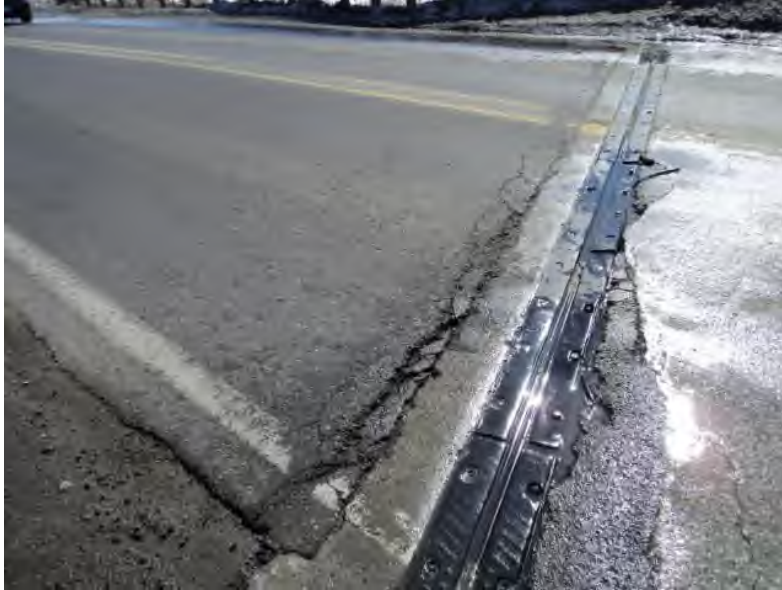
Figure 5.06.09 Other Joint – Block Out Style
