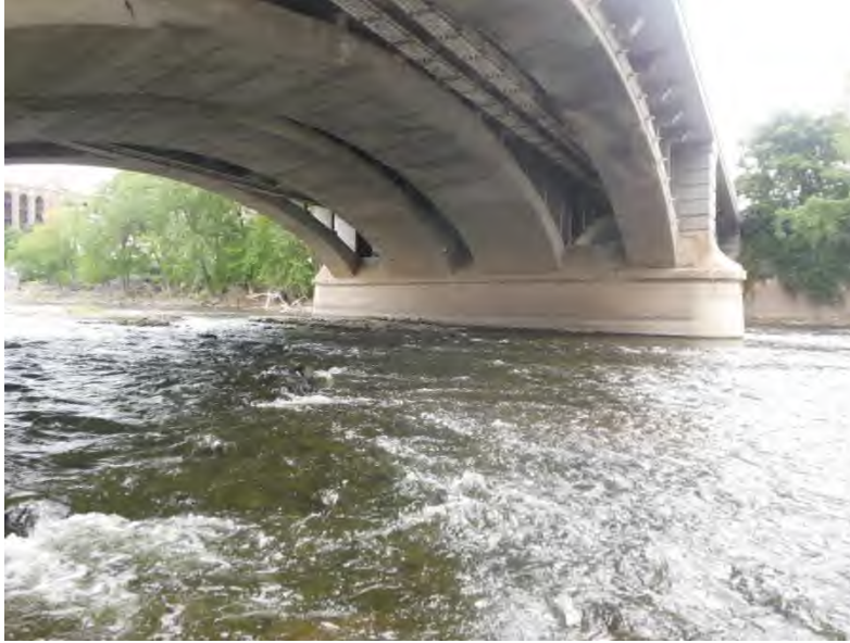
Figure 5.13.06 Open Spandrel Concrete Arch with Multiple Ribs
