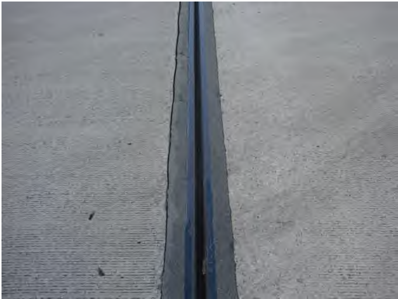
Figure 5.06.08 Other Joint – Partial Depth Strip Seal
