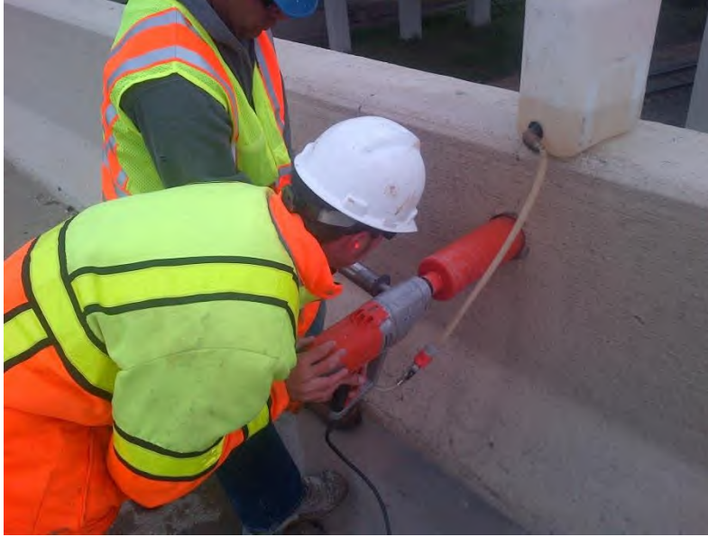
Figure 5.08.27 Coring Concrete Railing for ASR Testing
