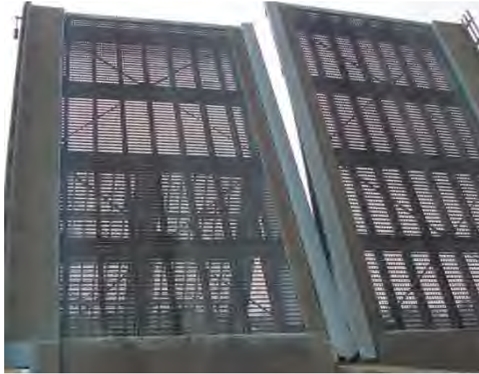
Figure 5.11.04 Twin Bascule Welded Steel Grid Decks
