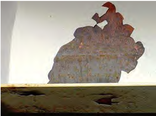
Figure 5.14.04 Cracking/Peeling/Curling
