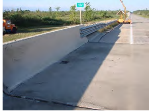
Figure 5.08.02 Type 4 Railing Item 36 A=1
