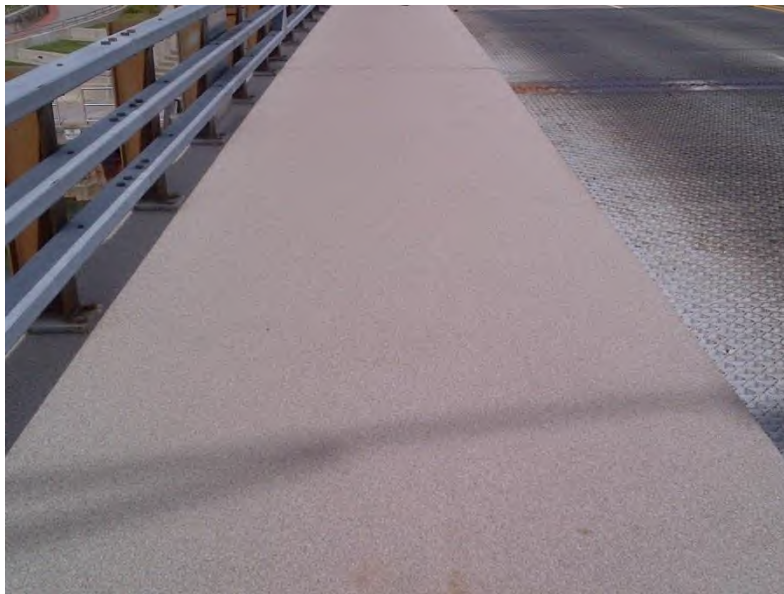
Figure 5.09.03 Concrete Filled Steel Grid with Wearing Surface
