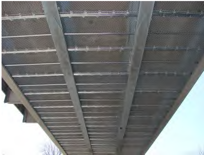
Figure 5.10.05 Typical Maintenance Sheeting
