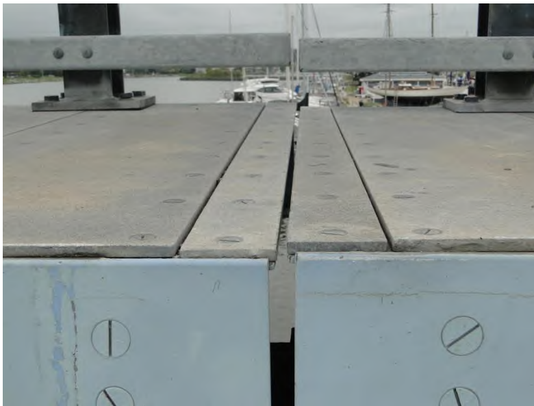
Figure 5.06.06 Open Expansion Joint
