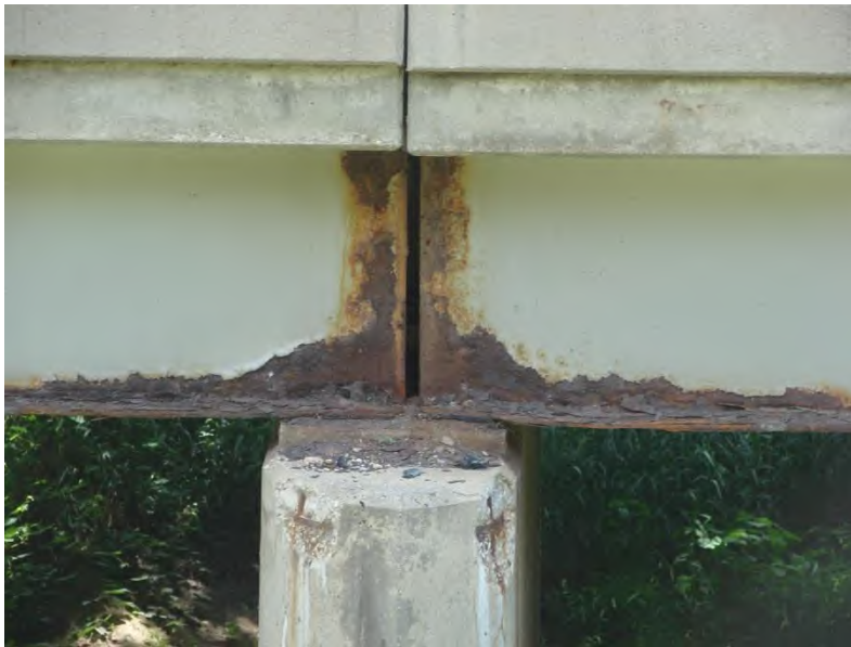
Figure 5.15.01 Identification of Beam End Corrosion Requires In-Depth Inspection
