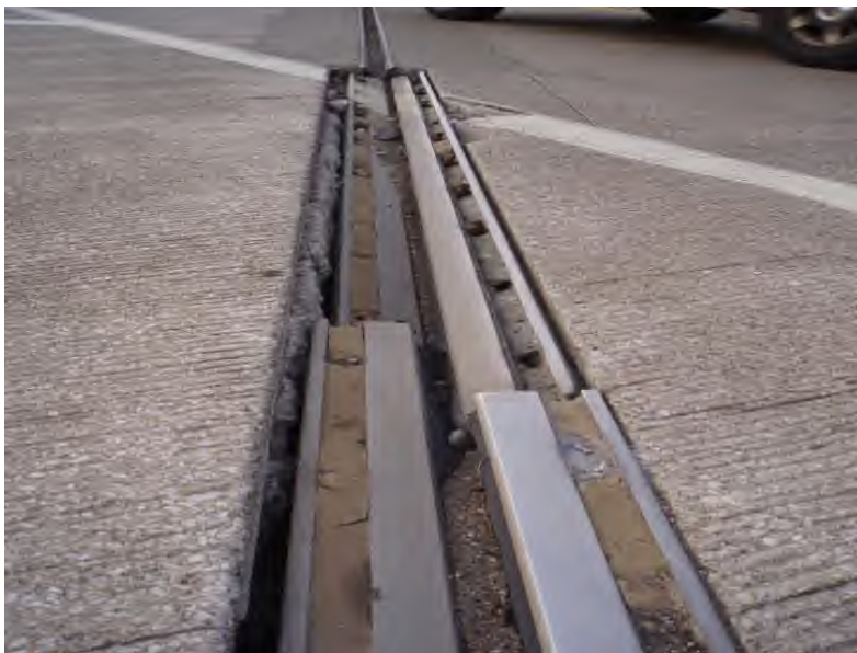
Figure 5.06.10 Mixed Joint Consisting of Elements 300 and 306
