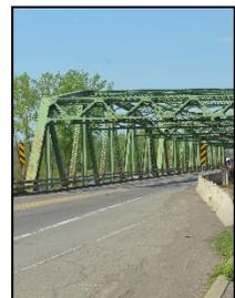
Figure 3: Truss bridge
