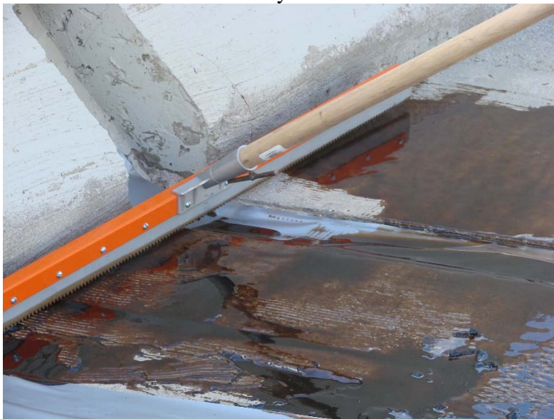
Figure 18 Notched squeegees (1/4 inch) spread thin overlay epoxy at the correct thickness.
