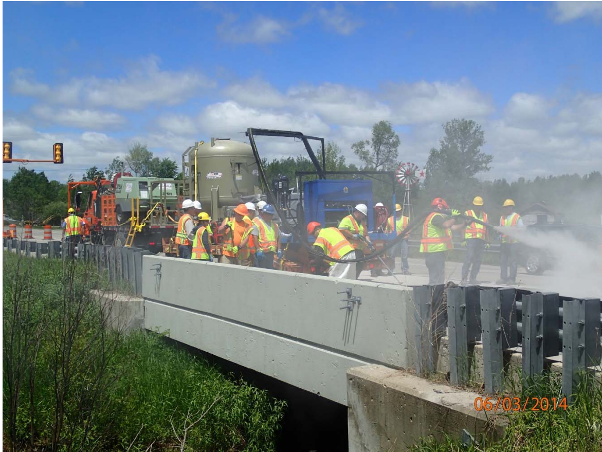
Figure 21 Blast pot delivering aggregate to operator
