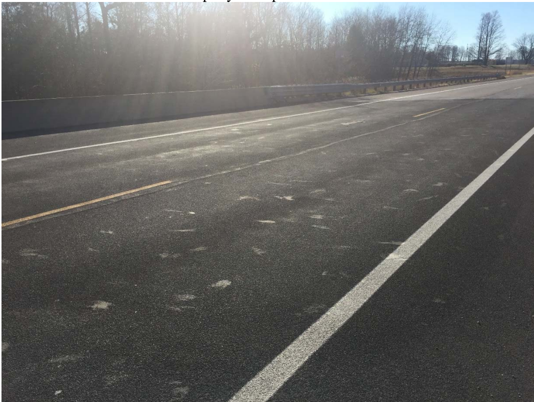
Figure 17 Drip locations appear “wet”, and are easily peeled up.
