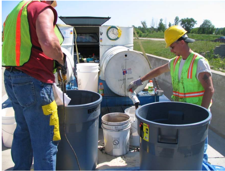
Figure 14 Contained mixing station with calibrated containers and a clock ensures the material is mixed accurately.
