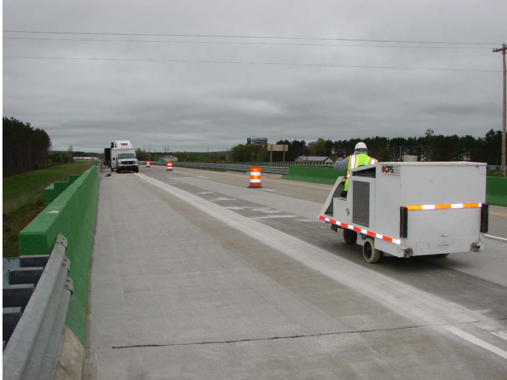
Figure 3 Shotblasting in preparation of a thin epoxy overlay.
