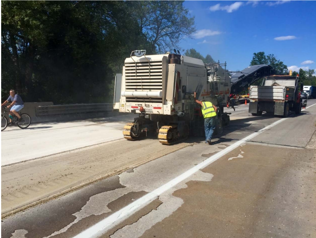
Figure 12 - Removal of thin epoxy overlay by fine tooth mill.
