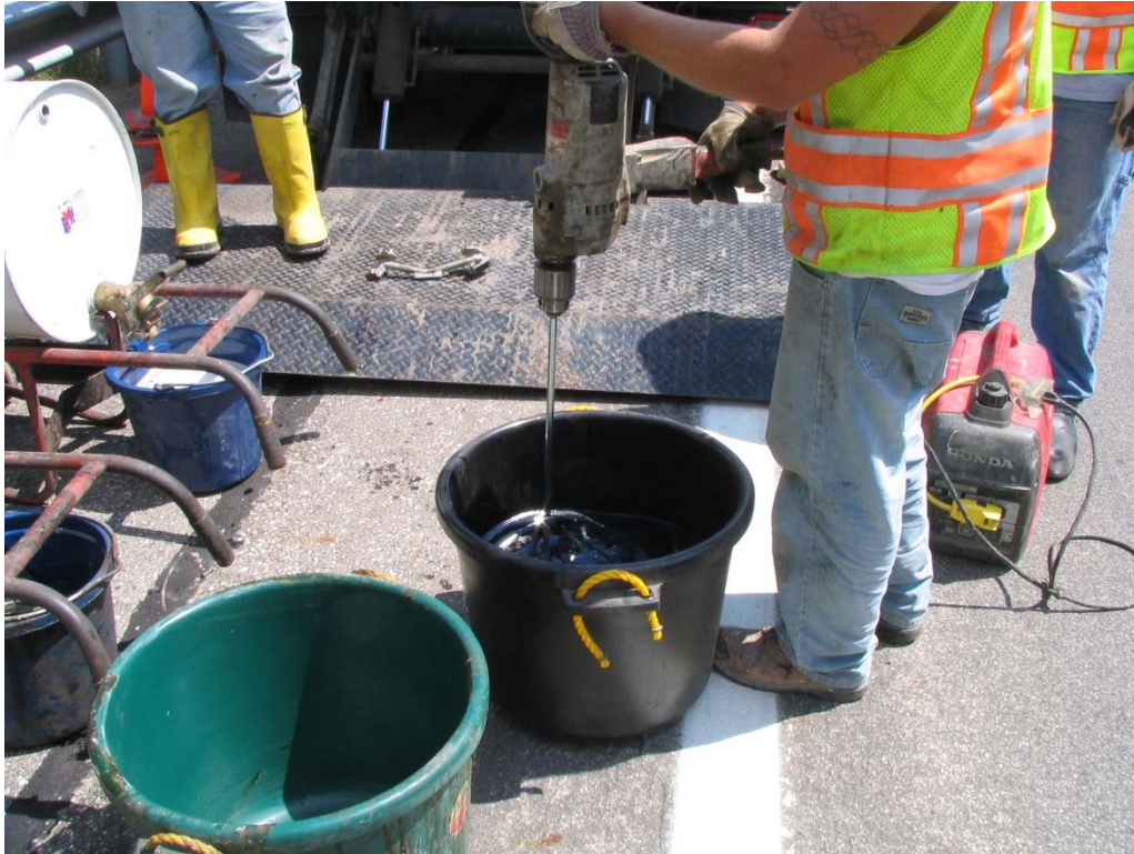
Figure 15 An electric drill with Jiffy® type mixing paddle combines the resin and hardener.
