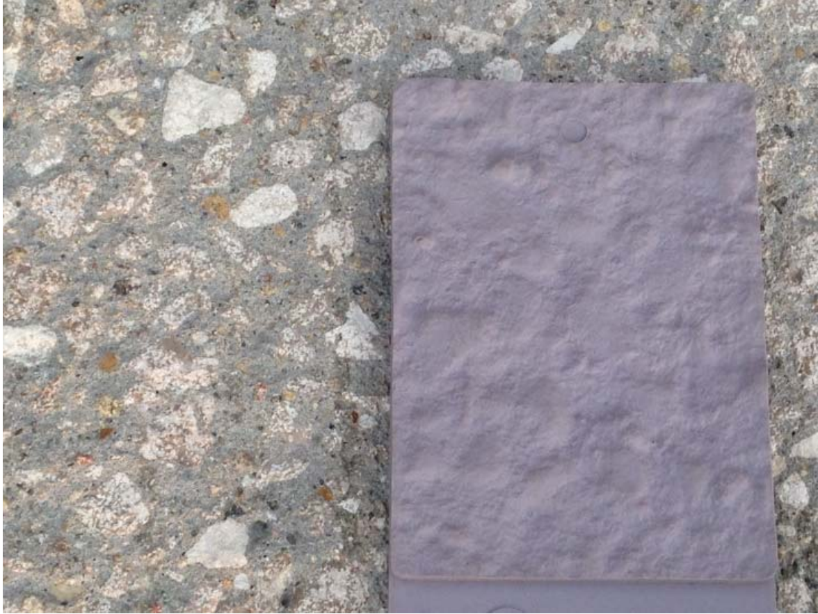
Figure 9 Proper profile provided by shotblasting for a thin epoxy overlay (Note the amount of exposed aggregate)
