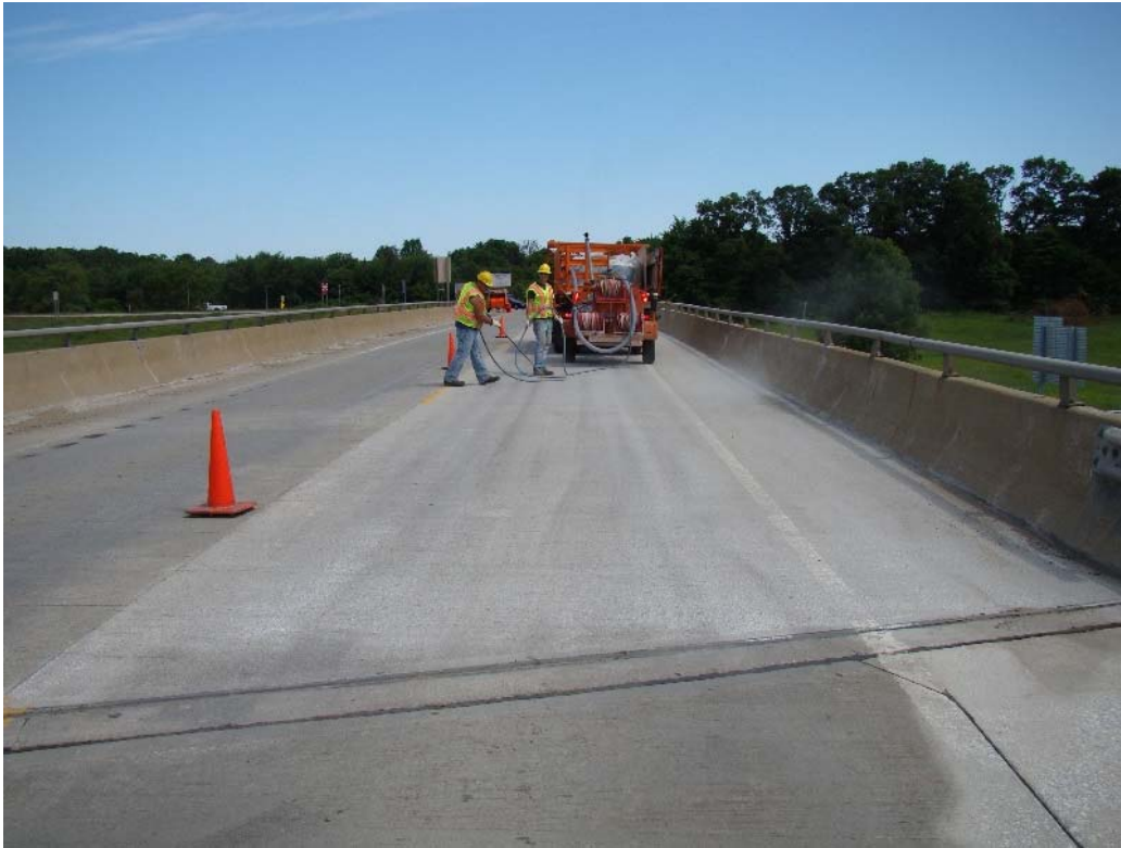
Figure 11 Dry compressed air is used to remove loose surface particles.
