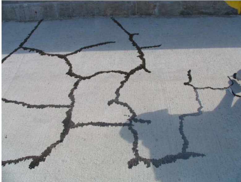
Figure 2 Crack chasing operation
