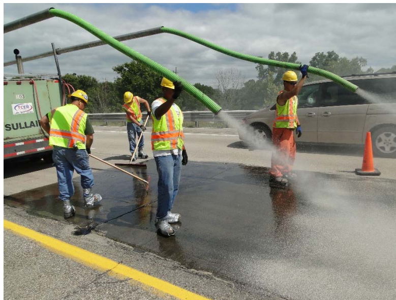
Figure 20 Two venturi units spreading aggregate substantially increase production.
