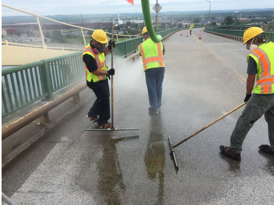
Figure 19 Asphalt seal-coating brushes are used to spread healer sealer epoxy from deck surface.
