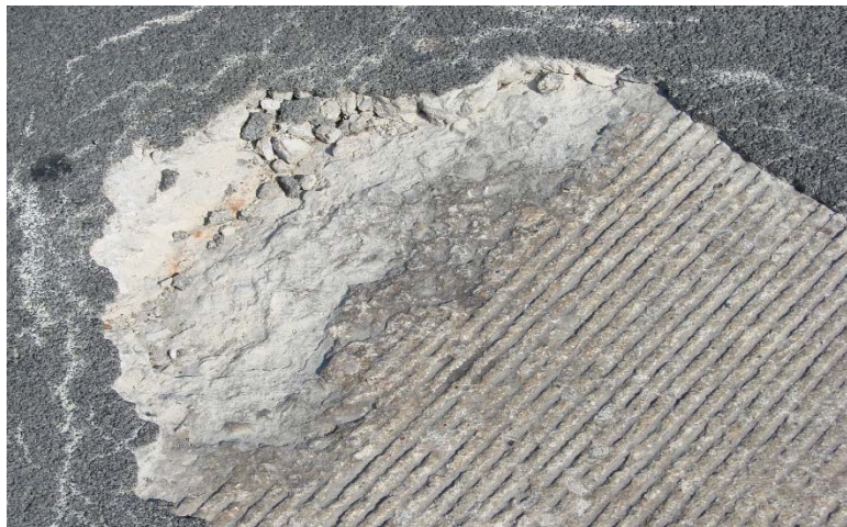
Figure 8 Thin overlay failure due to improper surface preparation.
