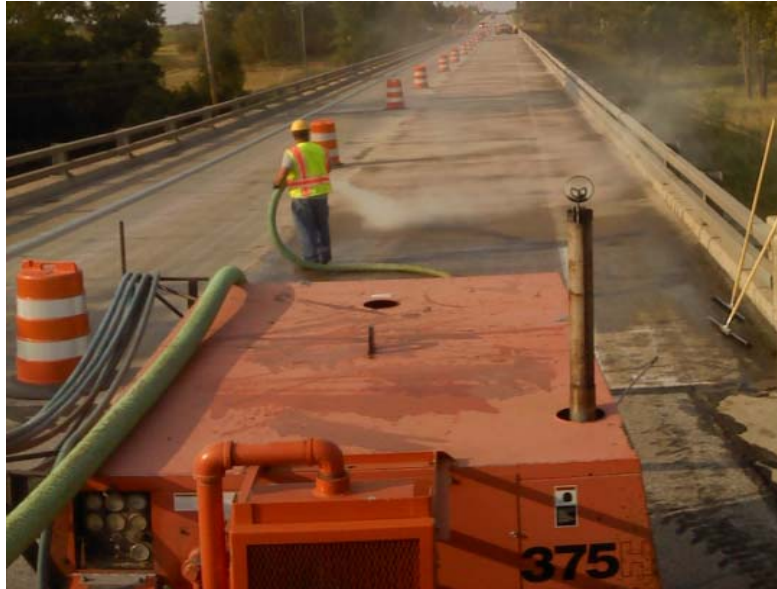
Figure 26 Sand placement during a healer sealer application.
