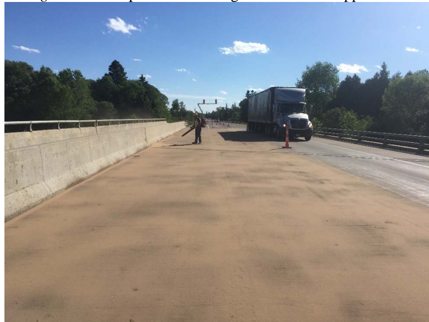
Figure 27 - Excess sand removal from healer sealer application.
