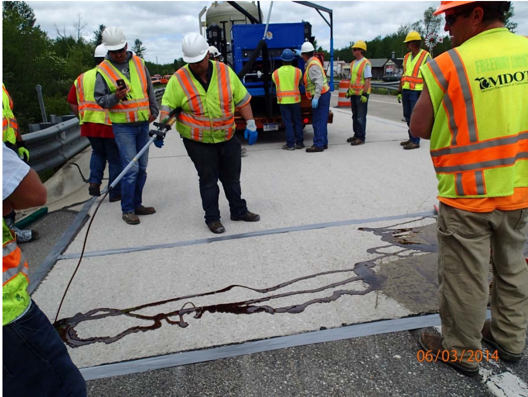
Figure 16 A Lily Epoxy Dispensing Pump delivers Part A and Part B to a mixing nozzle where the epoxy is dispensed onto the deck.
