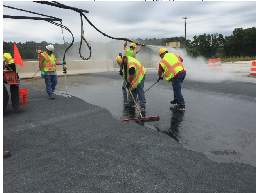
Figure 22 – Full Epoxy Operation
