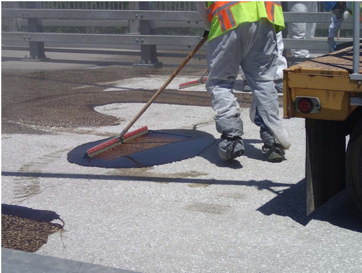
Figure 1 Flooding a bridge deck with a thin overlay epoxy
