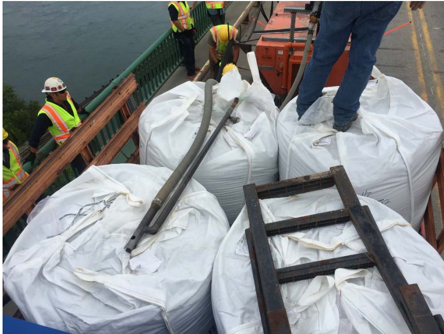
Figure 23 A modified aggregate drop pipe for venturi systems
