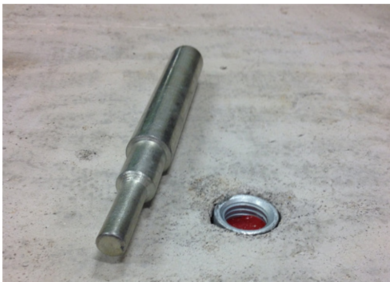
Figure 28. Anchor flush with concrete surface prior to seating plug with the setting tool.
