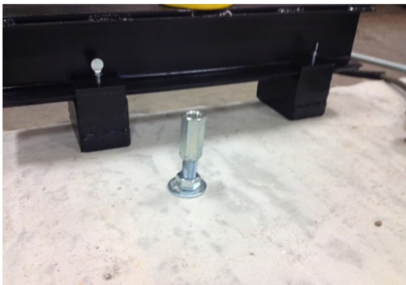
Figure 27. Coupling nut threaded halfway onto anchor. Some coupling nuts have stoppers at the halfway mark.
