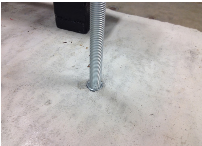
Figure 29. Temporary threaded rod fully seated in the anchor.
