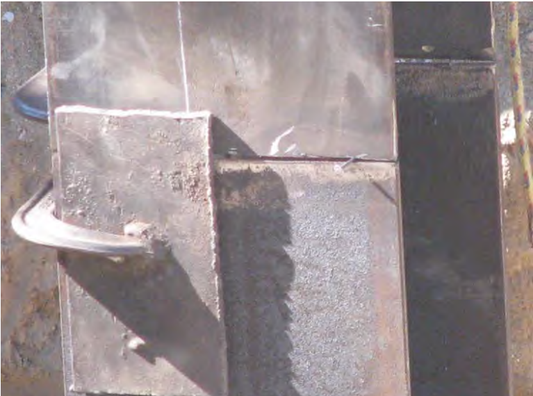
Figure 22. Good fit up and alignment. Groove weld showing progression of passes.
