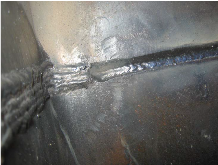
Figure 28. Additional passes being added to the root pass.
