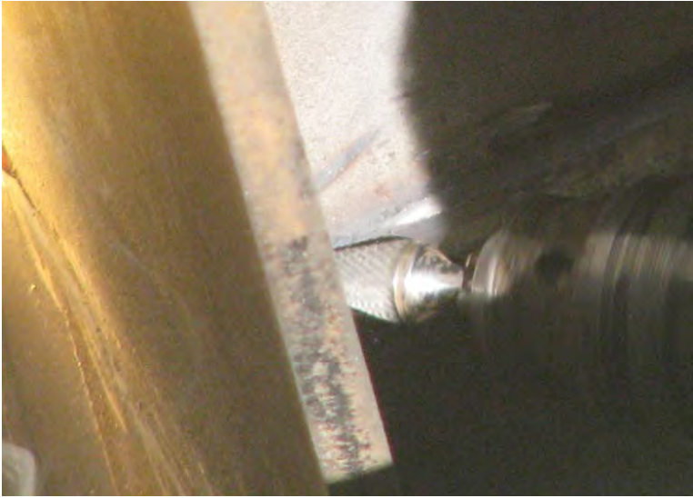
Figure 25. Back gouging with a die grinder.
