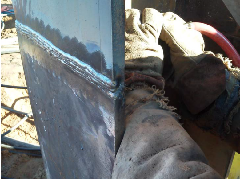
Figure 29. Back gouging to sound metal before welding the back side.
