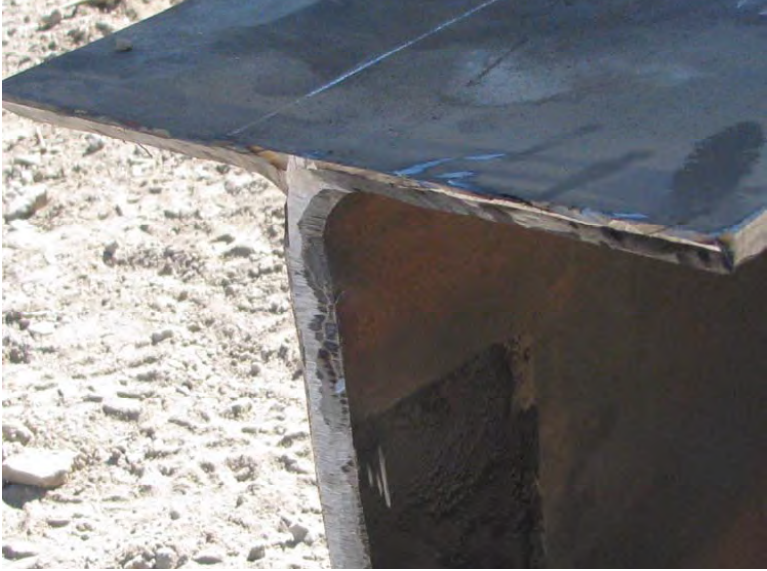
Figure 21. H-Pile beveled for a full penetration groove weld.
