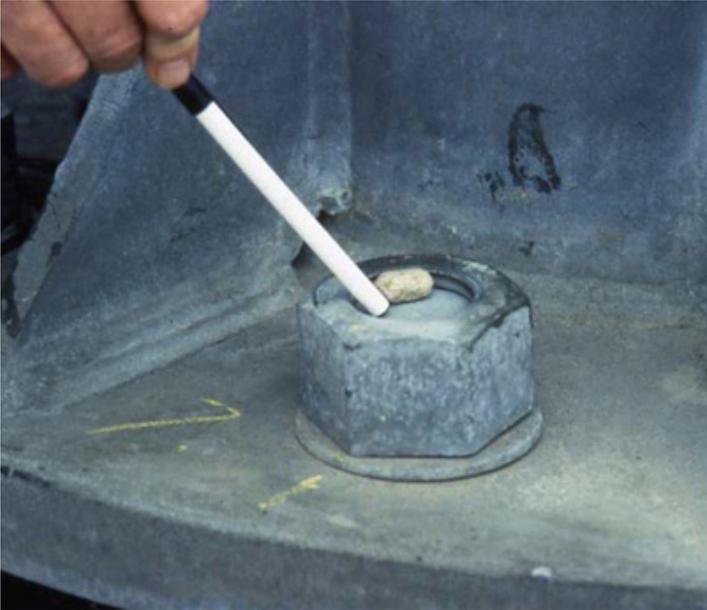
Figure 32: Insufficient anchor bolt projection from nut.
