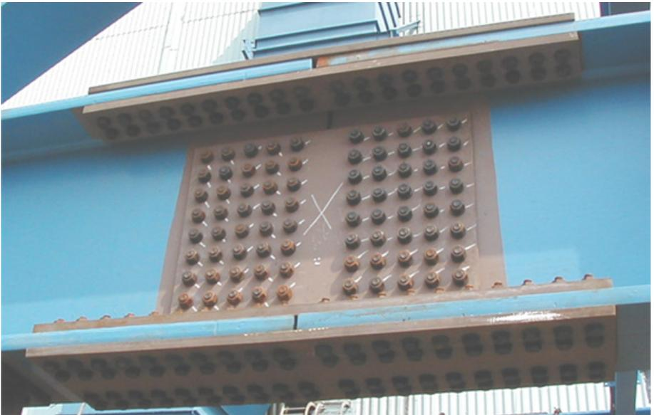
Figure 21: Inspect the TON match marks to ensure the bolts have been properly pre-tensioned.
