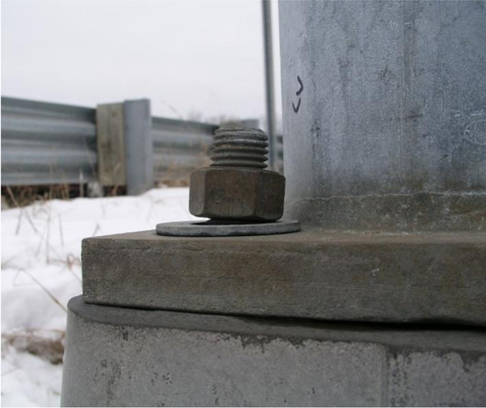
Figure 30: Misaligned anchor bolt that may be acceptable if beveled washers are used.
