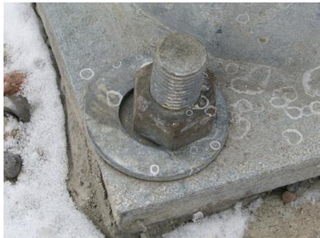
Figure 25: Incorrect washer size.
