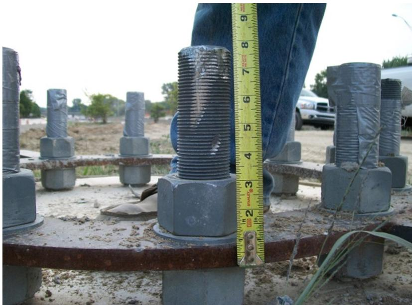
Figure 26: Damaged anchor bolt threads.
