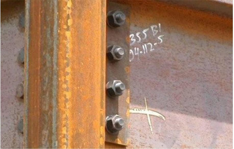
Figure 20: Acceptable bolt stick-out.
