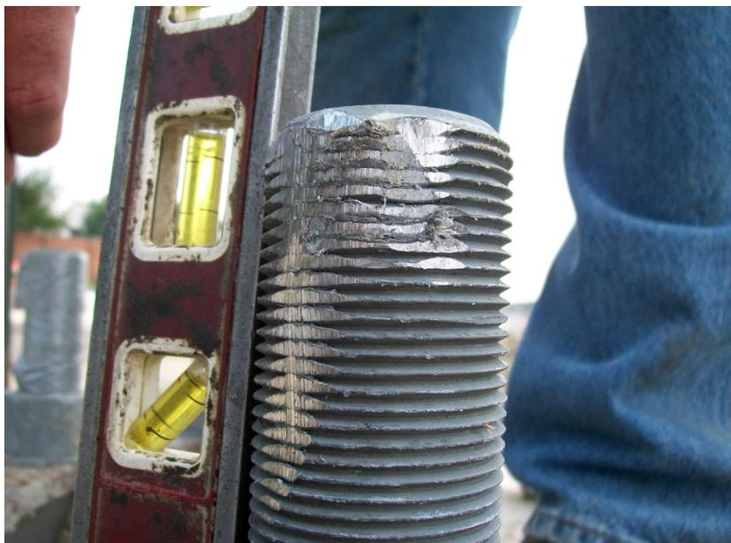
Figure 27: Damaged anchor bolt threads.
