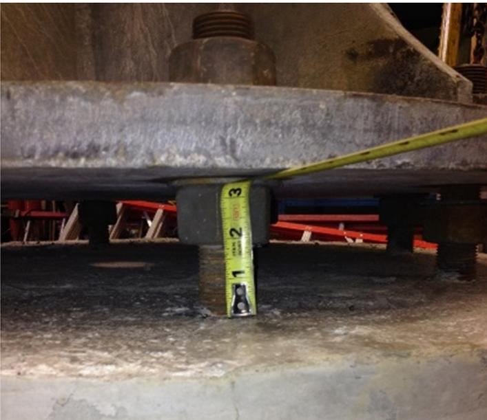
Figure 33: Standoff distance greater than 1 inch.
