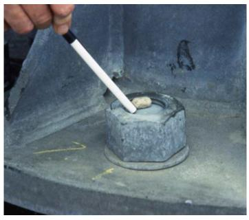
Figure 32: Insufficient anchor bolt projection from nut.
