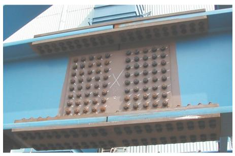
Figure 21: Inspect the TON match marks to ensure the bolts have been properly pre-tensioned.
