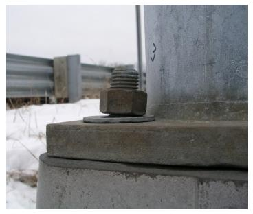
Figure 30: Misaligned anchor bolt that may be acceptable if beveled washers are used.
