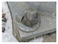
Figure 25: Incorrect washer size.
