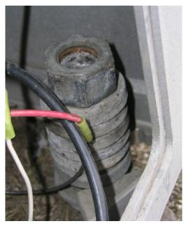
Figure 28: Stacked washers and insufficient anchor bolt projection.
