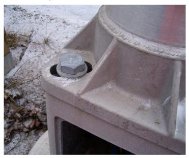
Figure 31: Anchor bolt hole and washer incompatibility.
