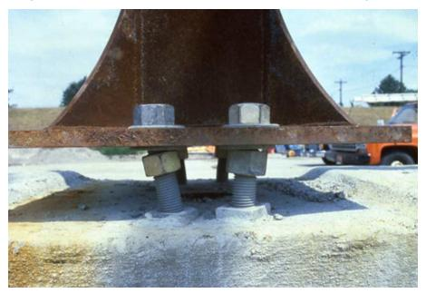
Figure 29: Misaligned anchor bolts greater than 1:40 out-of-plumb.
