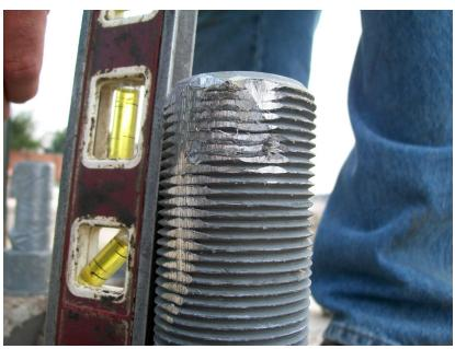
Figure 27: Damaged anchor bolt threads.
