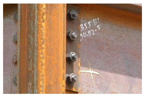
Figure 20: Acceptable bolt stick-out.
