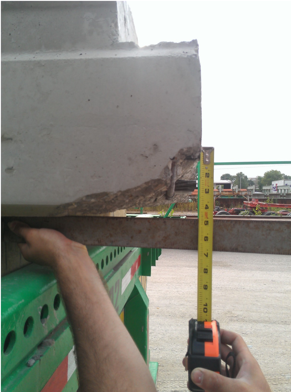
Figure 7. Spalled bottom corner at end of box beam.
