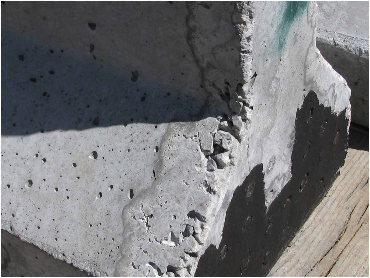
Figure 4. Moderate honeycombing at end of PCI beam.
