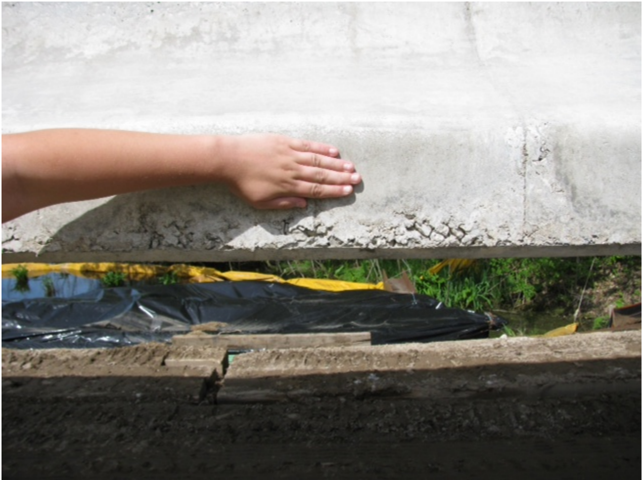
Figure 3. Moderate honeycombing along MI 1800 girder.
