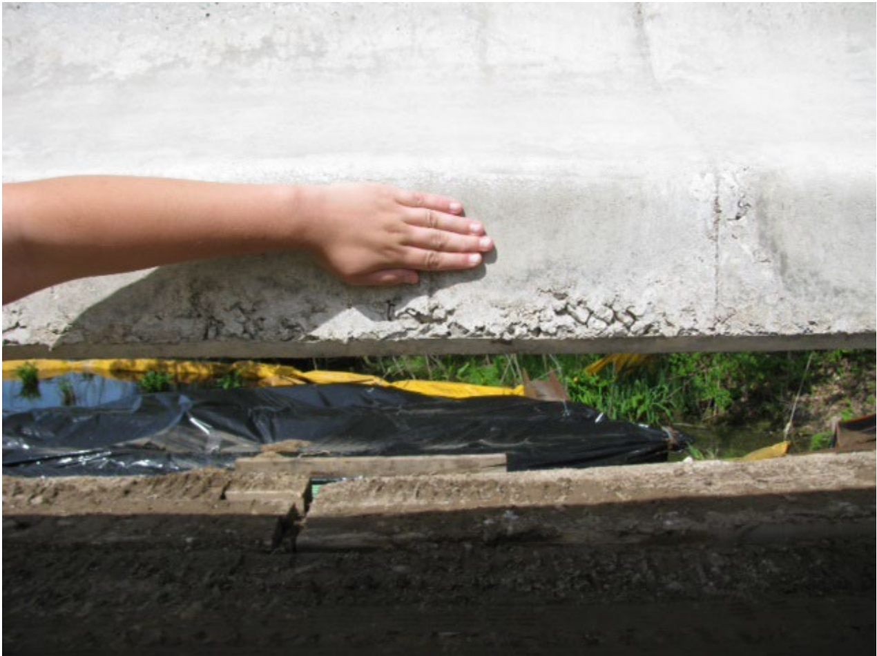
Figure 3. Moderate honeycombing along MI 1800 girder.
