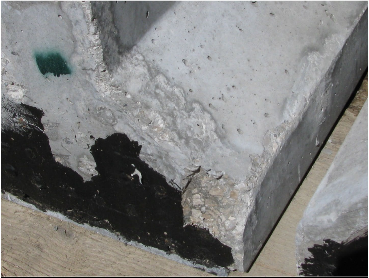
Figure 5. Broken corner at end of PCI beam.
