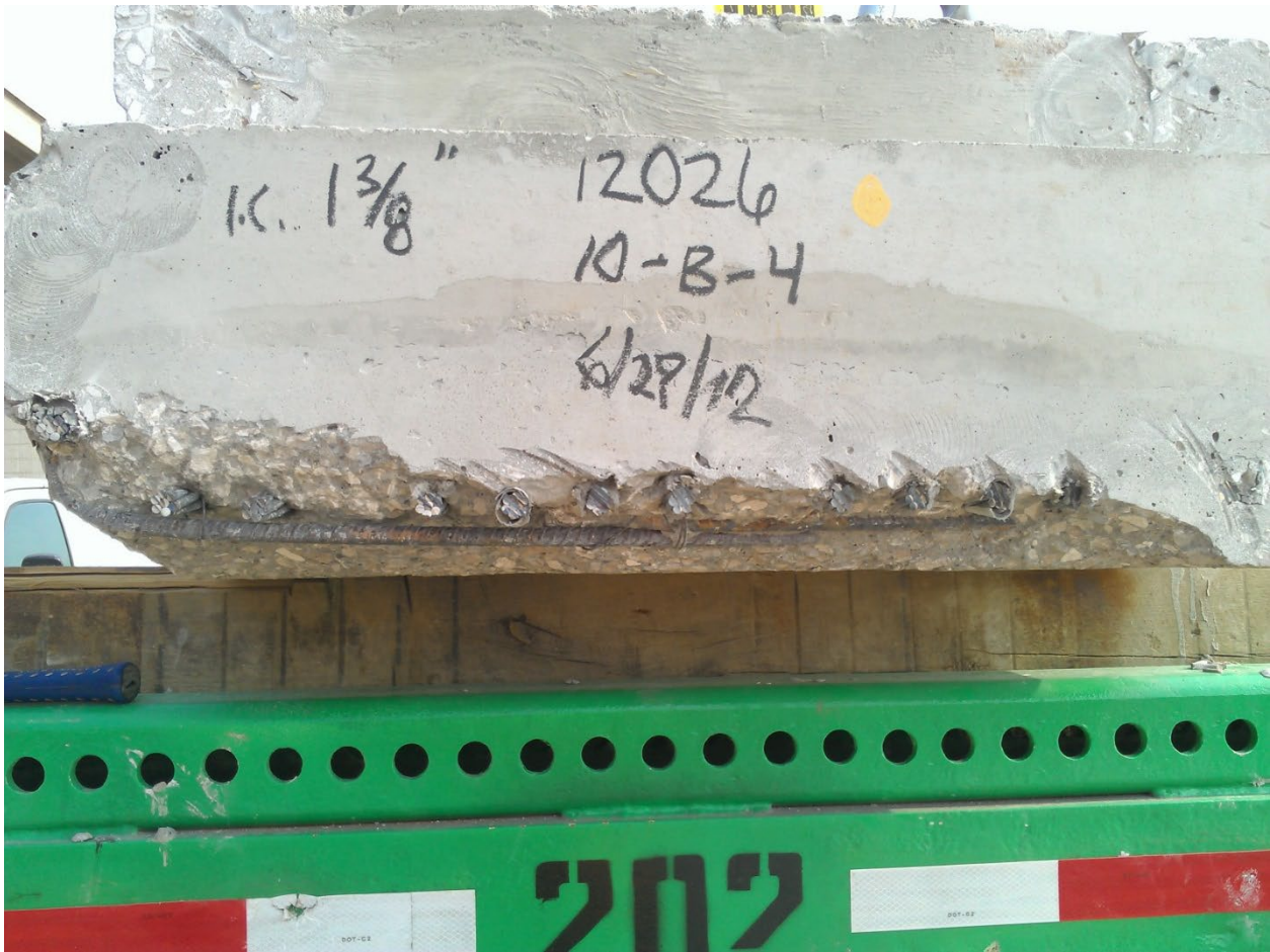
Figure 6. Spalled bottom corner at end of box beam.
