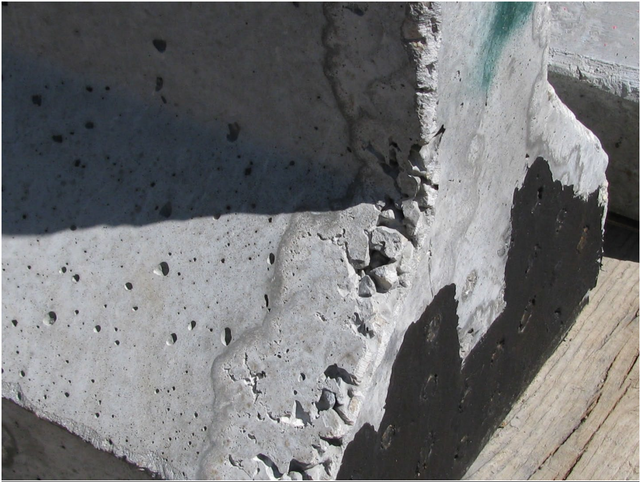
Figure 4. Moderate honeycombing at end of PCI beam.
