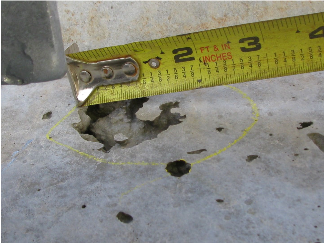
Figure 1. Air holes greater than 3/4" in any direction and greater than 3/8" deep.
