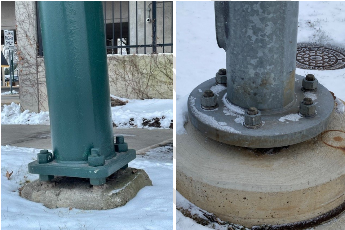
Figure 8.7.7: Steel strain pole square foundation with four anchor bolts (left, note misalignment), newer style drilled shaft foundation with six anchor bolts (right)
