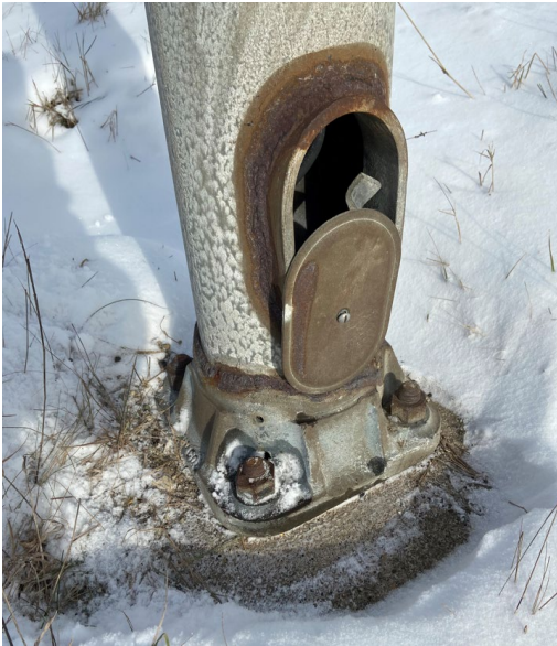
Figure 8.11.19: Non-frangible pole structure vertical support column (upright), loosely covered handhole
