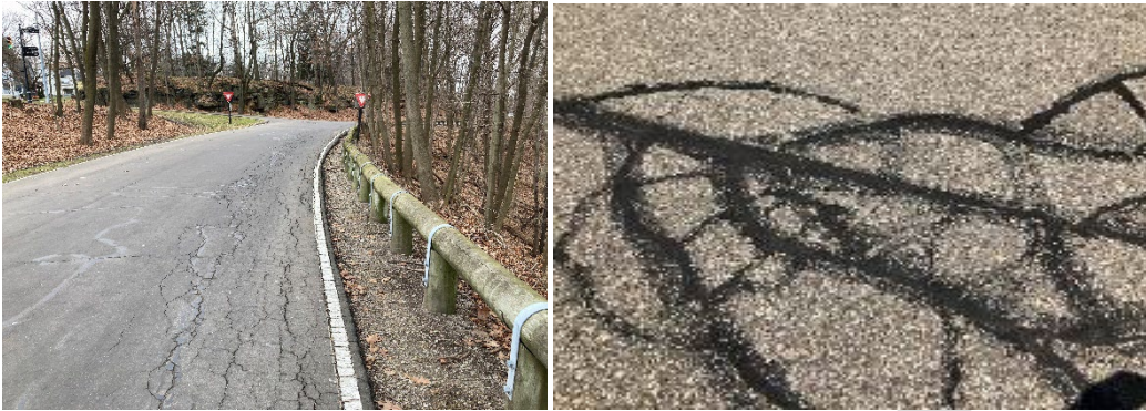
Figure 8.2.7: Pavement and shoulder alligator cracking
