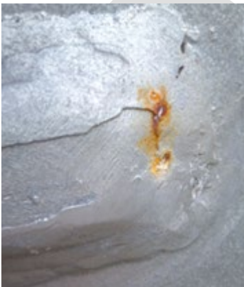
Figure 8.4.14: Vertical structure connection, rust bleeding through galvanizing at welded gusset plate arm to vertical structure upright
