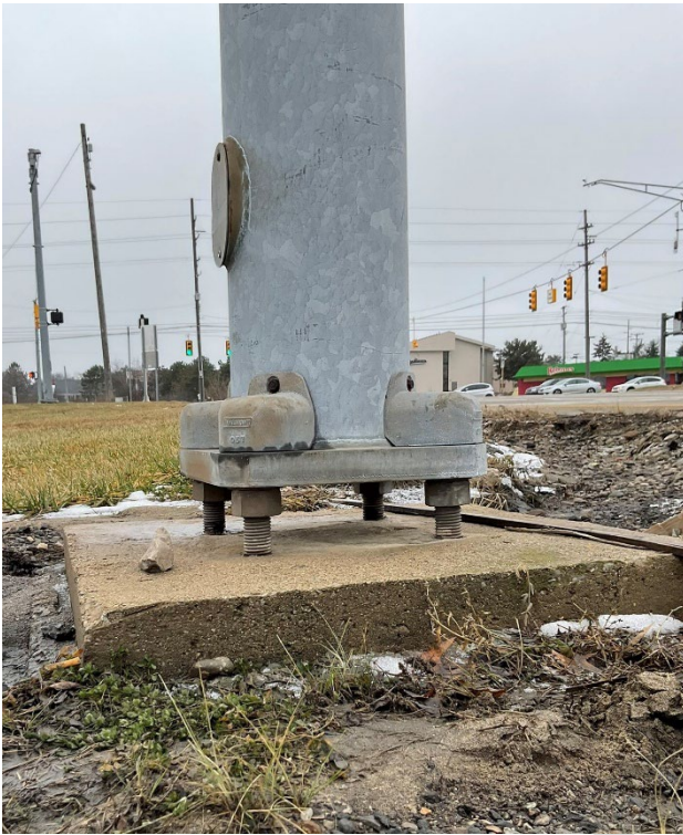
Figure 8.7.10: Steel strain pole foundation with excess standoff distance and nut covers
