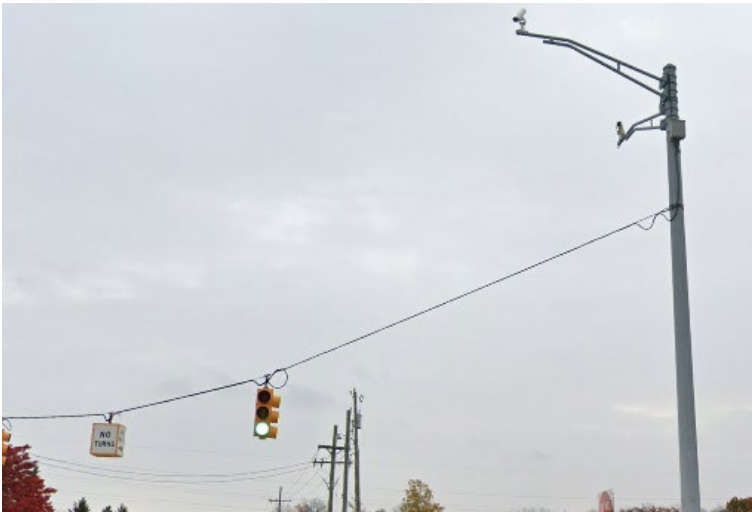
Figure 8.7.20: Cameras mounted on luminaire truss arms
