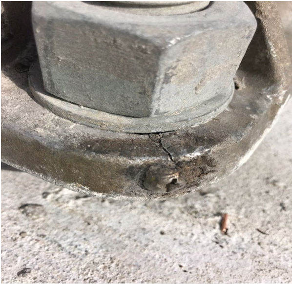
Figure 8.11.14: Non-frangible pole structure base plate crack
