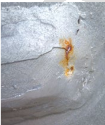
Figure 8.10.13: Vertical structure connection, rust bleeding through galvanizing at welded gusset plate arm to vertical structure upright
