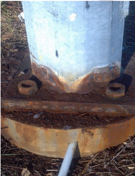
Figure 8.11.15: Non-frangible pole structure base plate, corrosion of base plate, anchor bolts, and nuts and inadequate bolt projection
