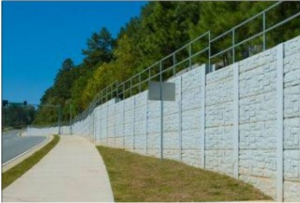
Figure 8.3.29: Soldier pile wall with precast lagging (note: anchors not shown)
