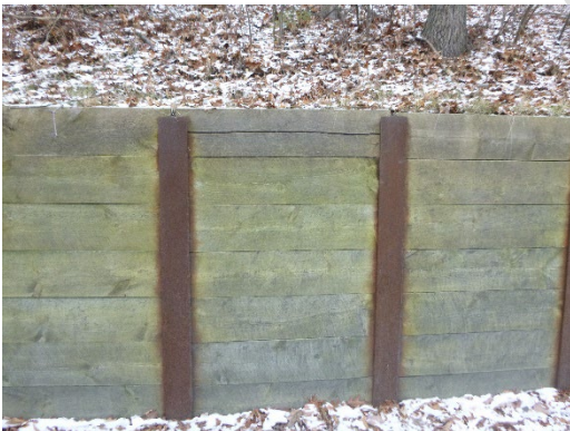
Figure 8.3.20: Timber lagging is split along top
