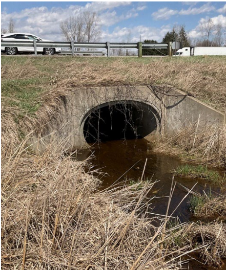
Figure 8.2.30: Concrete barrel culvert
