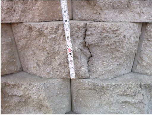
Figure 8.3.22: Vertical split in modular block
