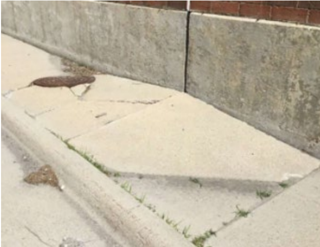
Figure 8.3.41: Wall settlement
