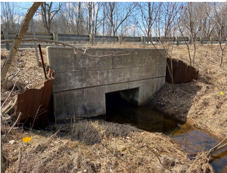
Figure 8.2.24: Concrete headwall and metal sheet pile wingwalls
