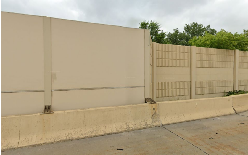
Figure 8.8.2: Noise wall mounted on crash barrier
