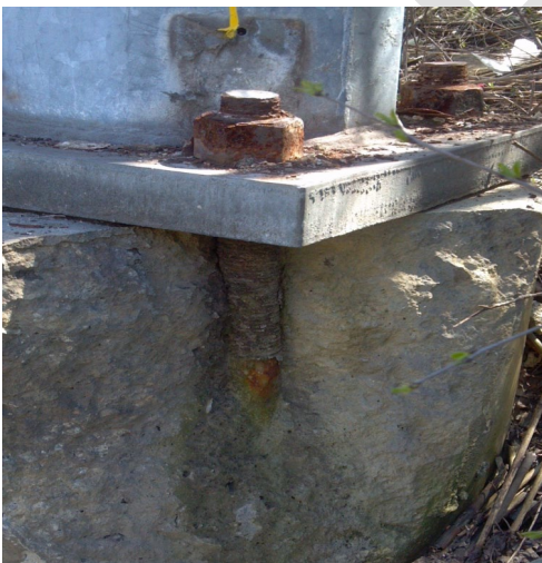
Figure 8.11.6: Concrete foundation, exposed anchor bolt in damaged foundation
