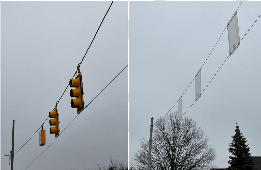
Figure 8.7.17: Span wire supporting signals and sign (left), span wires supporting signs (right)
