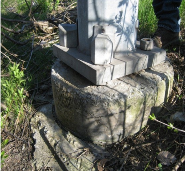
Figure 8.11.5: Non-frangible concrete foundation deterioration
