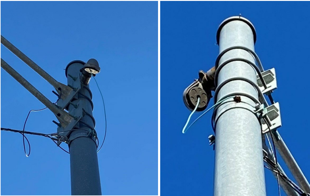
Figure 8.7.14: Steel strain pole bracket assembly connections for luminaire arms
