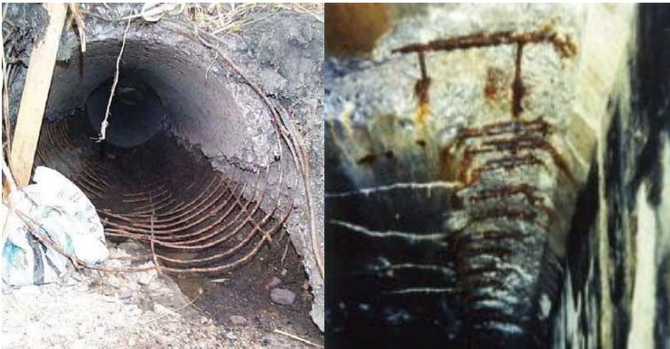
Figure 8.2.33: Concrete barrel deterioration
