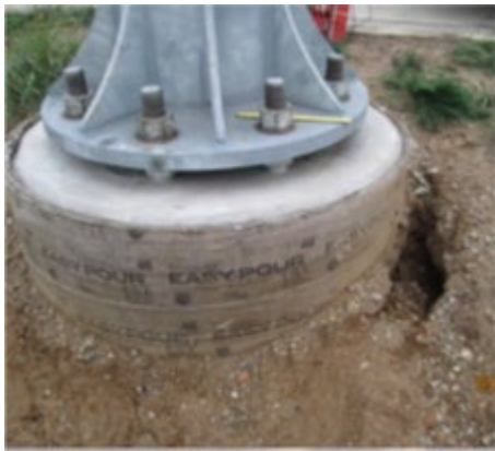
Figure 8.4.6: Erosion of soil around a truss or cantilever structure foundation
