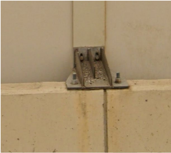
Figure 8.8.10: Noise wall attachment to concrete barrier
