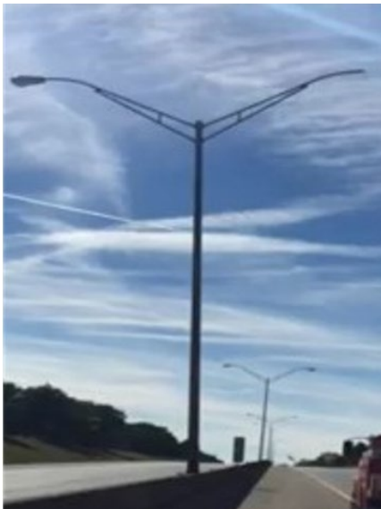
Figure 8.11.23: Luminaire and luminaire arm element, missing luminaire head
