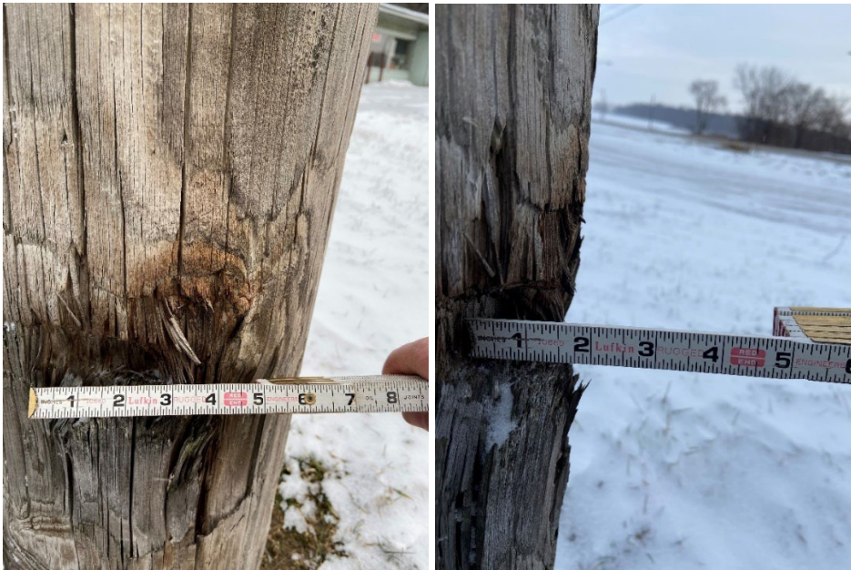
Figure 8.5.11: Measuring impact damage
