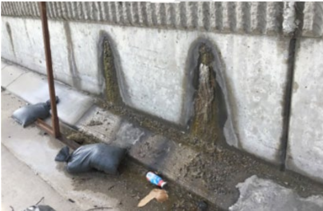
Figure 8.3.15: Weep holes/wall drainage
