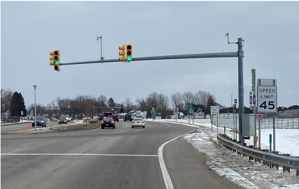
Figure 8.9.13: Mast arm structure with single arm
