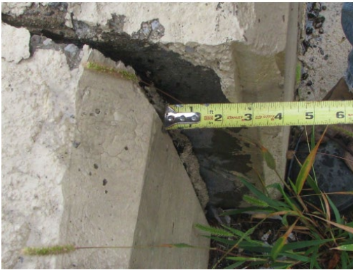
Figure 8.3.35: Wall displacement
