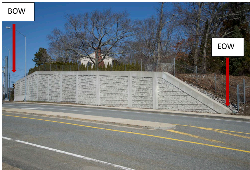
Figure 8.3.7: Typical wall facing inspection limits
