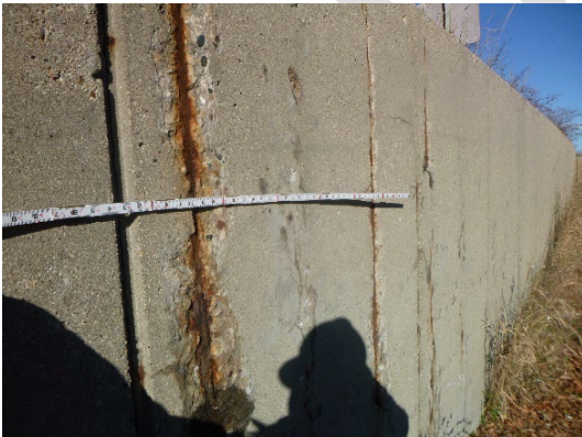
Figure 8.3.9: Corroded wall reinforcing
