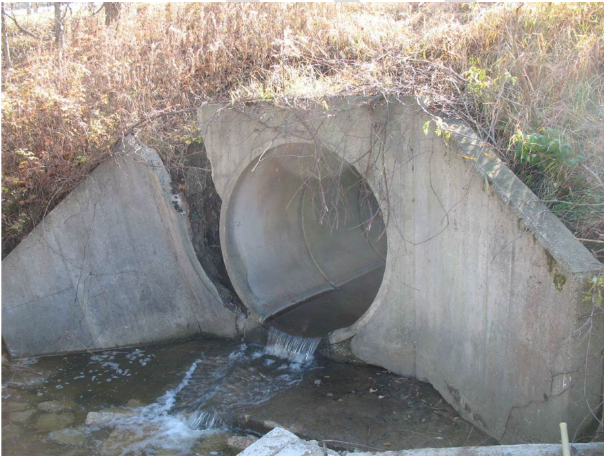
Figure 8.2.4.4.26: Concrete foundation and wingwall damage due to scour
