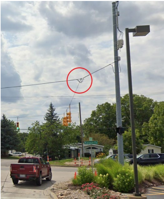
Figure 8.7.3: Steel strain pole with suspended/hanging box span configuration (suspension circled)
