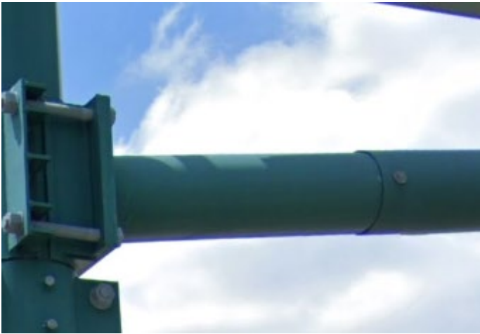
Figure 8.9.14: Mast arm member splice with connection bolt
