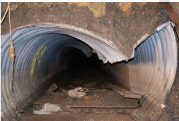
Figure 8.2.29: Loss of vertical alignment in a corrugated metal culvert
