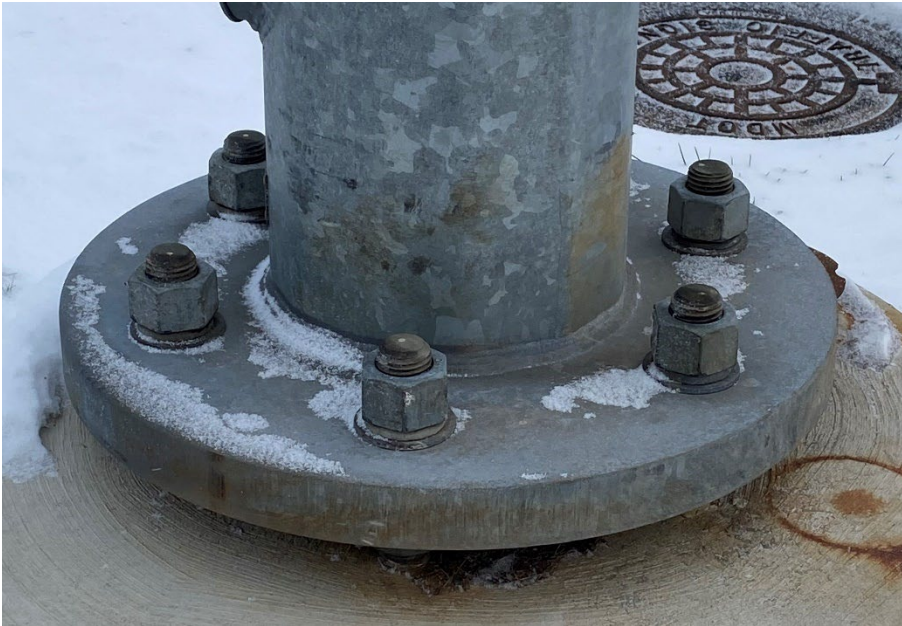
Figure 8.7.11: Steel strain pole base plate with six anchor bolts
