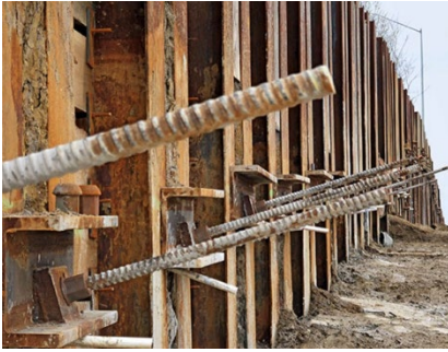
Figure 8.3.36: Wall anchor
