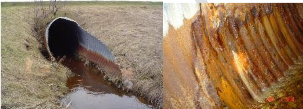
Figure 8.2.35: Loss of protective coatings contributing to corrosion
