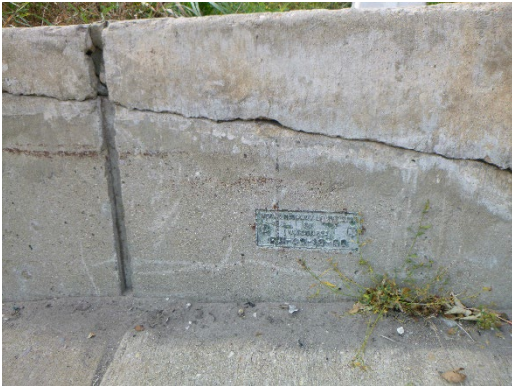
Figure 8.3.8: Horizontal structural cracking
