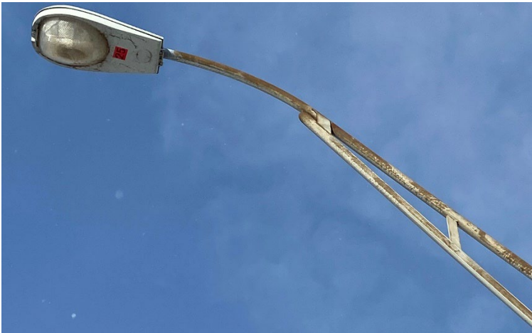
Figure 8.7.19: Luminaire and luminaire truss arm
