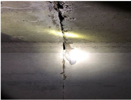
Figure 8.2.32: Spalling within a box culvert
