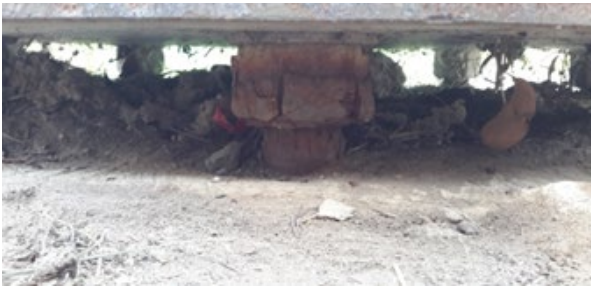
Figure 8.10.7: Leveling nut and anchor bolt corrosion with section loss
