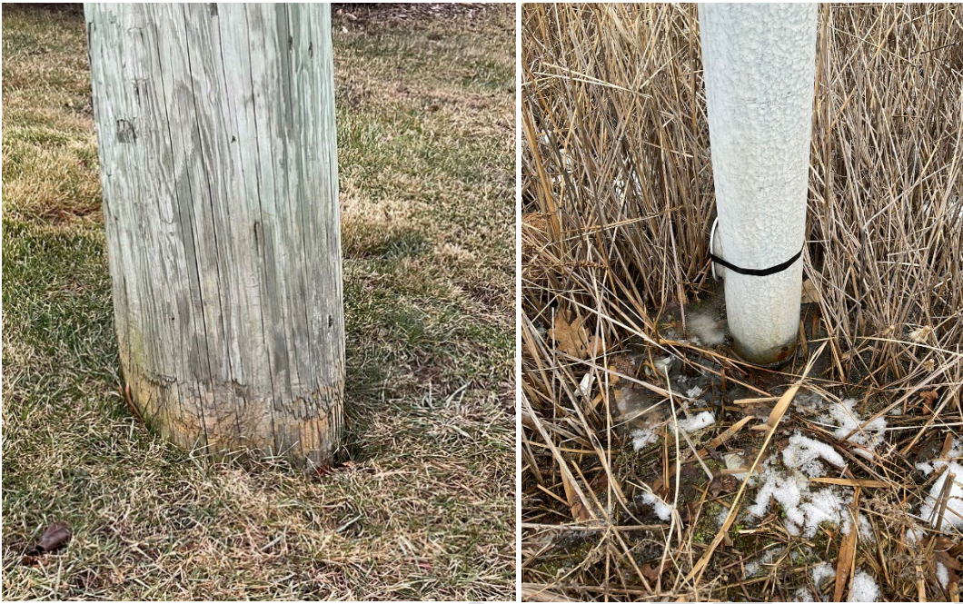
Figure 8.5.9: Wood pole embedment (left), steel pole embedment (right)
