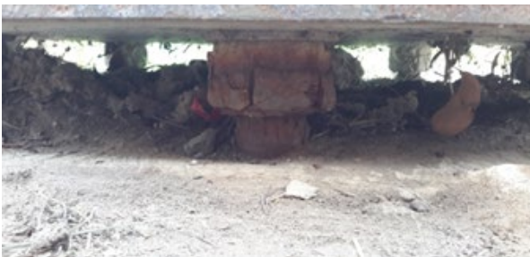
Figure 8.4.9: Leveling nut and anchor bolt corrosion with section loss
