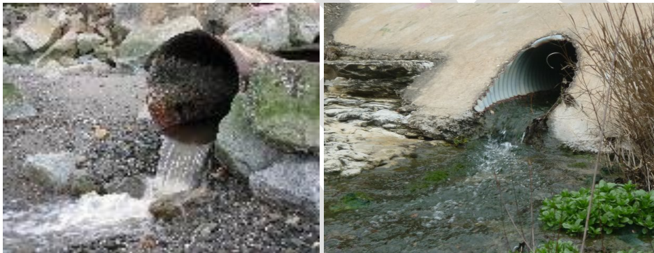
Figure 8.2.12: Stream channel poor vertical alignment (left) and horizontal alignment (right)
