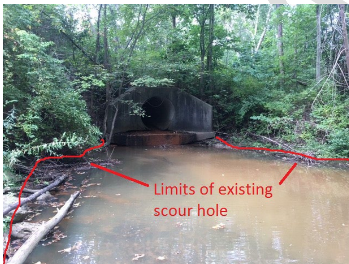
Figure 8.2.4.427: Perched outlet with large scour hole
