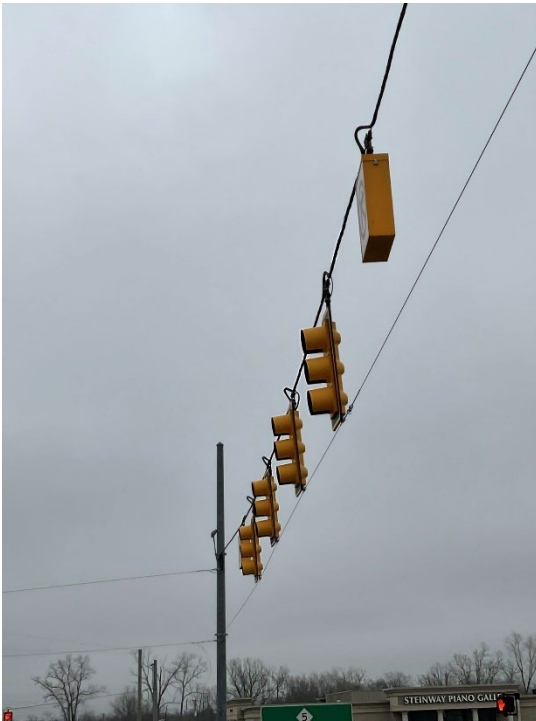
Figure 8.7.15: Steel strain pole span wire supporting signals and sign
