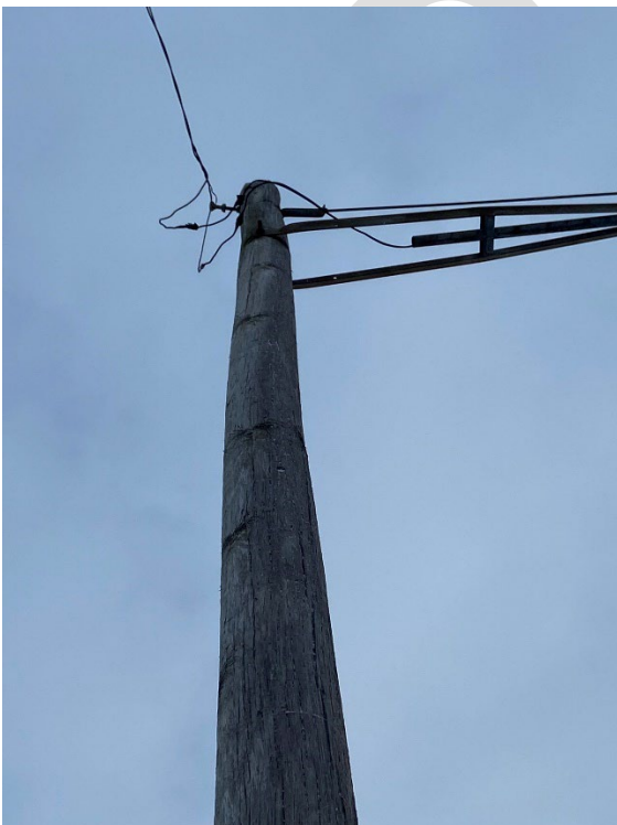
Figure 8.5.8: Minor crook in wood pole
