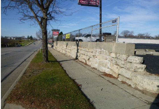
Figure 8.3.21: Typical square-stone masonry wall
