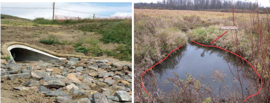
Figure 8.2.20: No scour (left), scour hole (right)
