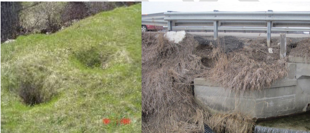
Figure 8.2.10: Example of embankment issues due to piping (left) or erosion (right)
