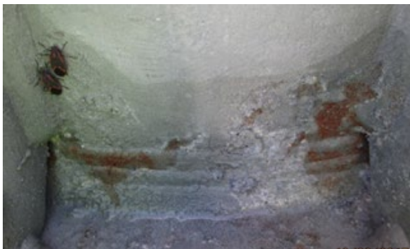
Figure 8.4.10: Cantilever or truss structure base plate and vertical support, rust underneath galvanizing repair
