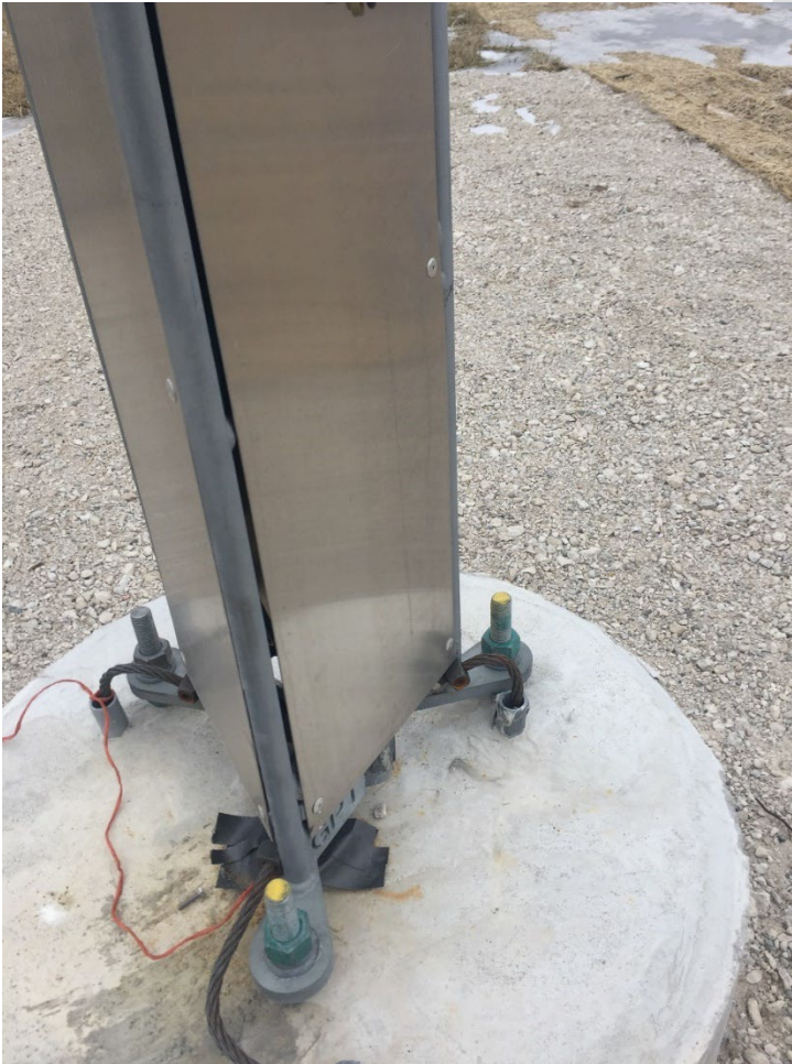
Figure 8.14.5: ESS tower base plate
