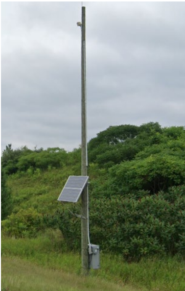
Figure 8.5.4: Embedded wood pole supporting ITS infrastructure
