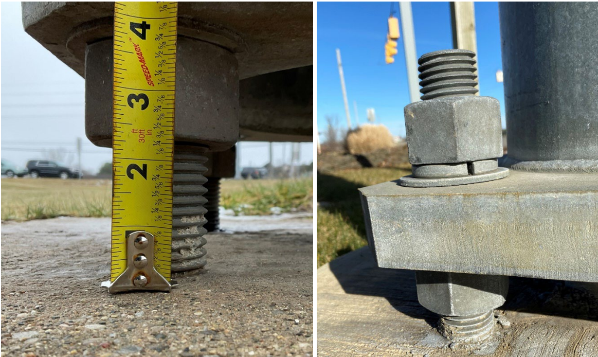
Figure 8.7.8: Excess anchor bolt standoff distance (left), fully compressed lock washer (right)
