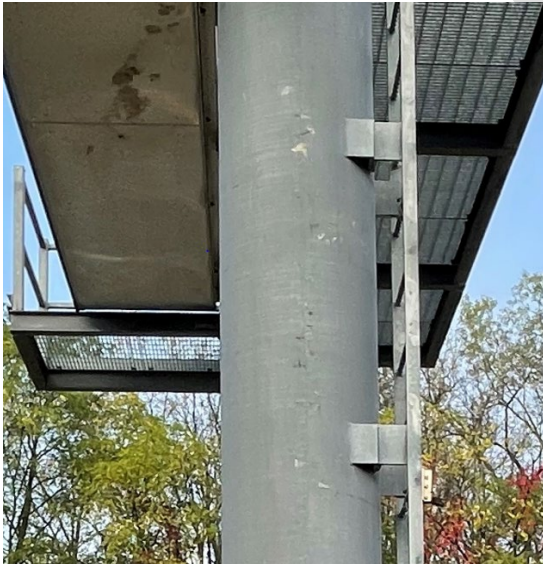
Figure 8.10.10: Vertical structure column (upright) with minor coating damage
