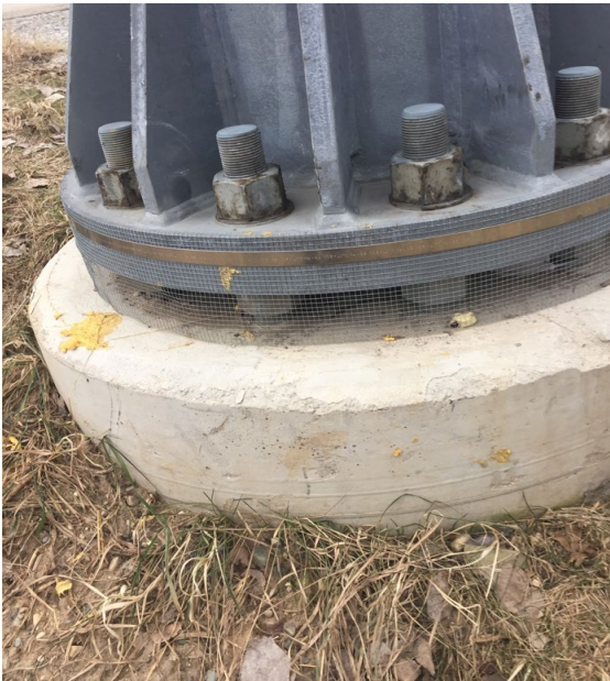
Figure 8.10.4: DMS support structure foundation, minor spalling
