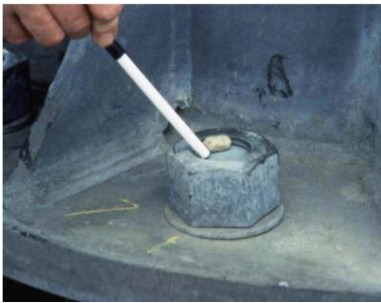
Figure 8.4.8: Cantilever or truss structure anchor bolts and leveling nuts, anchor nut without fully engaged threads
