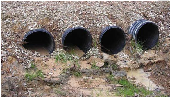
Figure 8.2.11: Culvert erosion—early-stage gully/rill erosion between the culverts
