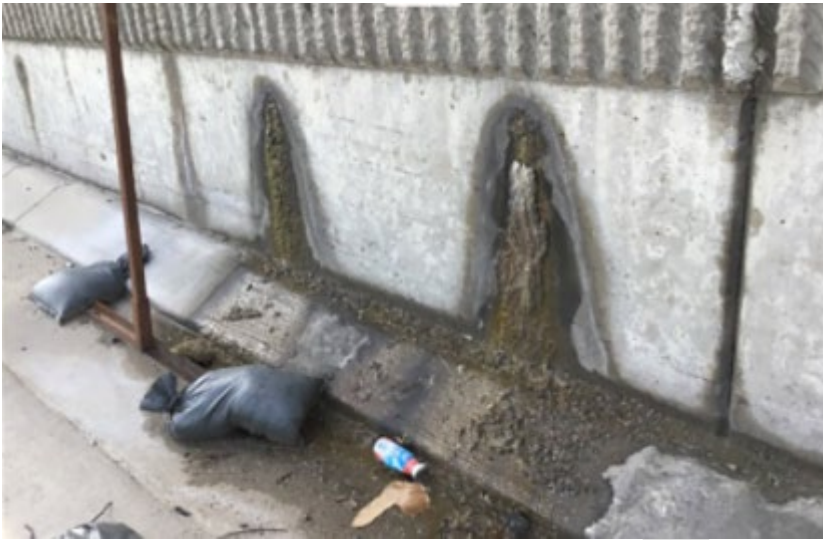
Figure 8.3.12: Retaining wall concrete abrasion
