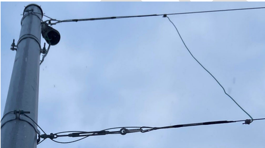
Figure 8.7.16: Span wire assemblies attached to steel strain pole band clamps
