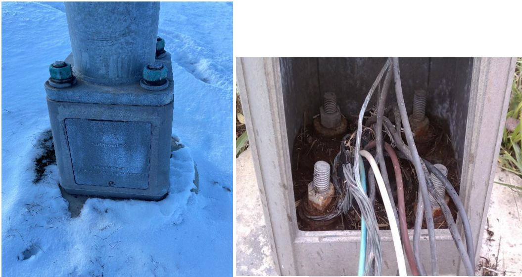
Figure 8.11.12: Frangible transformer base, panel door present (left), corrosion and debris in transformer base interior with missing panel door, and exposed wires (right)
