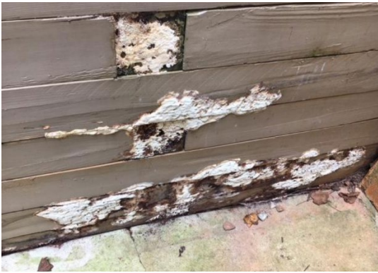
Figure 8.3.19: Timber lagging splitting
