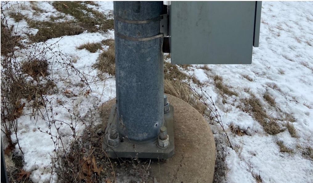
Figure 8.9.8: Mast arm base plate with four anchor bolts
