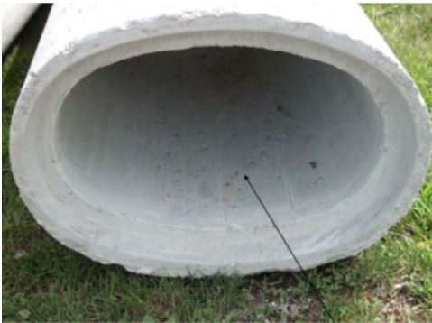
Figure 8.2.37: Elliptical concrete barrel
