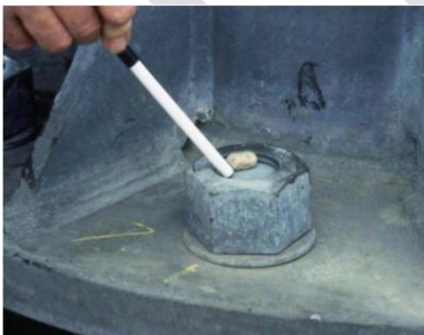
Figure 8.10.6: Anchor bolts and leveling nuts, anchor nut without fully engaged threads
