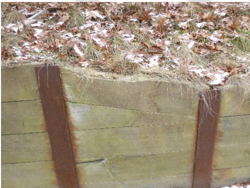
Figure 8.3.18: Section loss at top of wall
