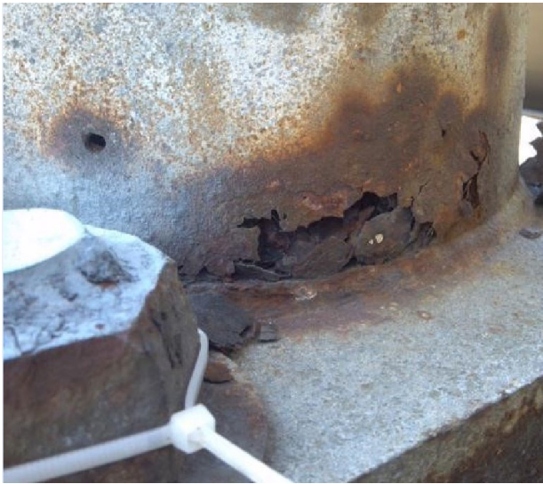
Figure 8.11.16: Base plate, pole corrosion and section loss at base weld
