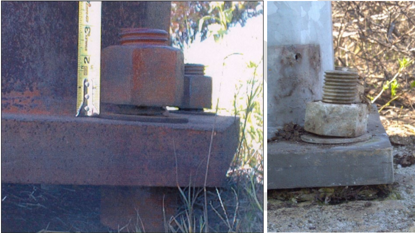
Figure 8.11.10: Anchor bolt and leveling nut foundation, gap between anchor nut and washer in corroding base unit (left), gap between anchor nut and washer with bolt out of plumb and debris between upright base and concrete foundation (right)
