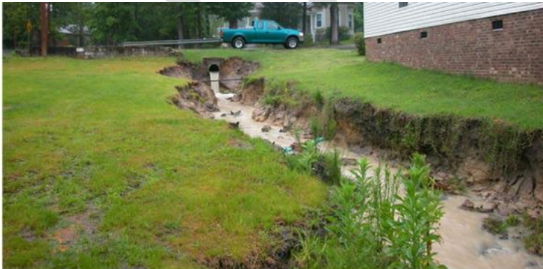
Figure 8.2.19: Bank erosion
