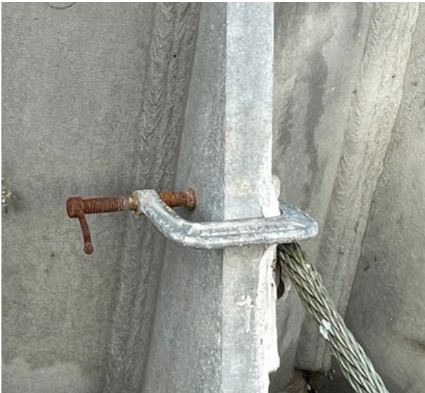
Figure 8.10.9: Corrosion in bonding clamp along bolt of base plate stiffener
