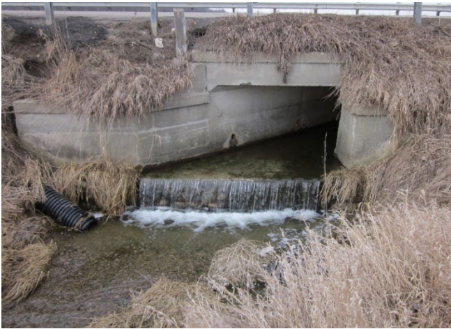
Figure 8.2.15: Vertical alignment issue leading to stream degradation
