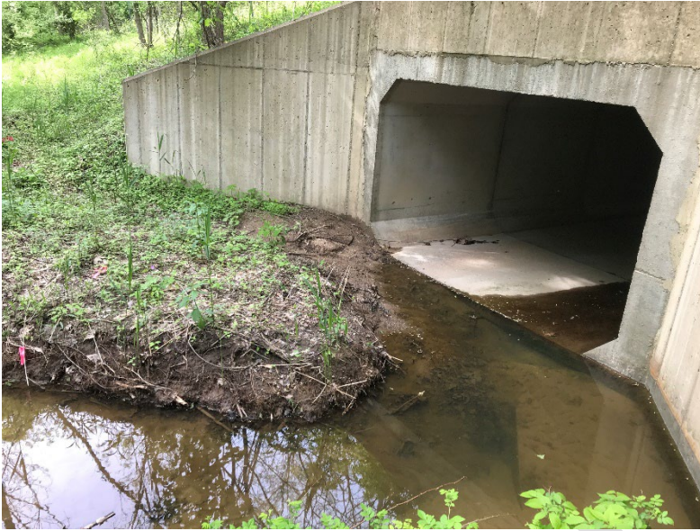
Figure 8.2.13: Stream channel poor horizontal alignment
