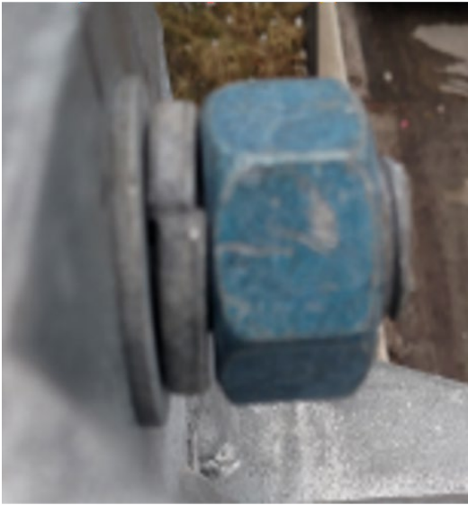
Figure 8.10.12: Vertical structure connection, loose bolt/lock washer not fully compressed
