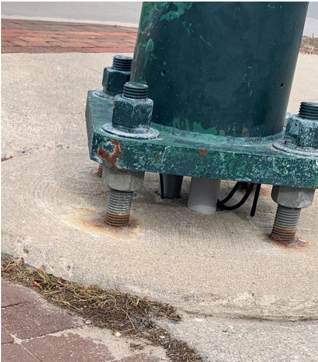
Figure 8.9.7: Four anchor bolt foundation with excessive standoff distance and corrosion
