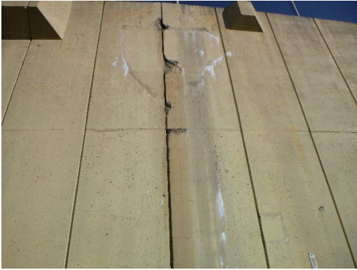
Figure 8.3.14: Efflorescence accumulation
