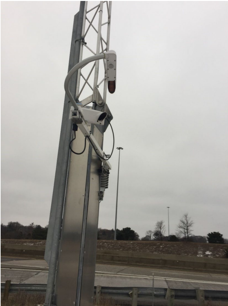
Figure 8.14.6: ESS tower vertical support column with ITS attachments
