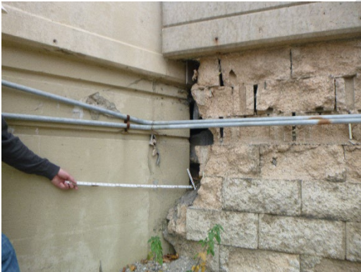
Figure 8.3.23: Masonry breakdown
