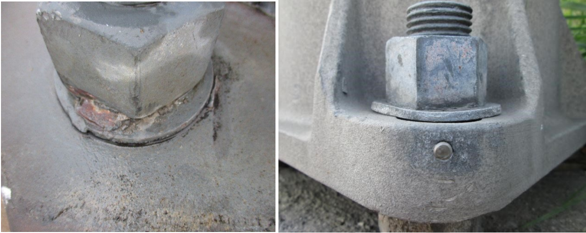
Figure 8.11.11: Anchor bolt and leveling nuts foundation, nut tack welded to washer (left), incorrect washer type – plate washers intended to cover slotted holes (right)
