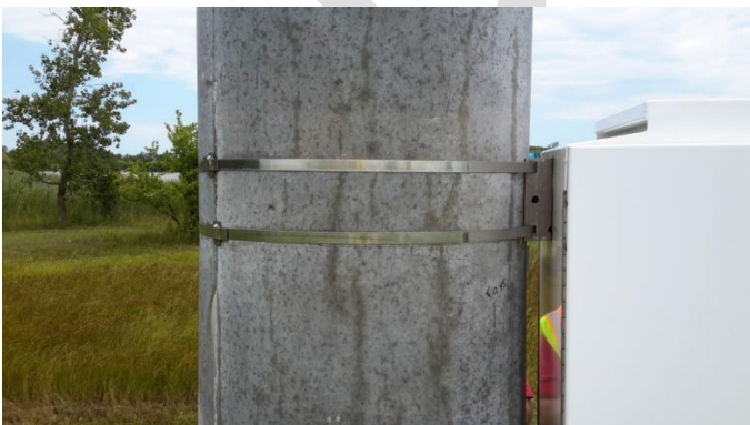
Figure 8.6.7: Band clamp connection to metal enclosure
