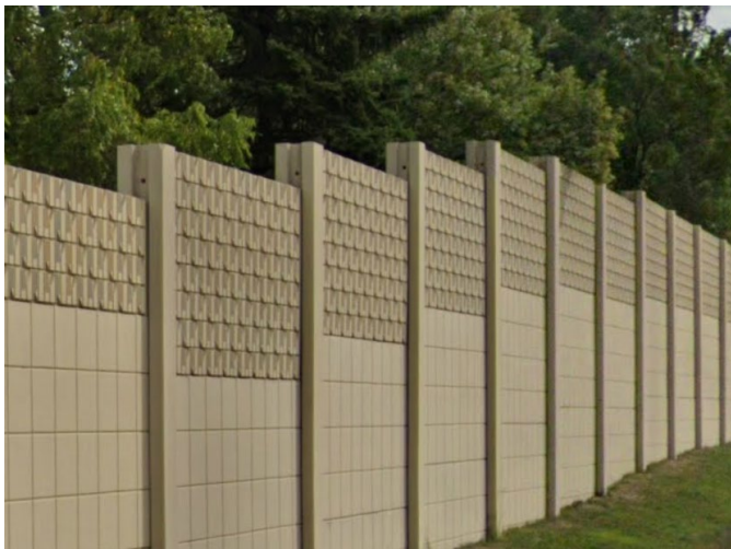
Figure 8.8.6: Noise wall with vertical support columns
