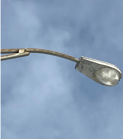
Figure 8.11.22: Luminaire and luminaire arm element, evidence of galvanizing damage
