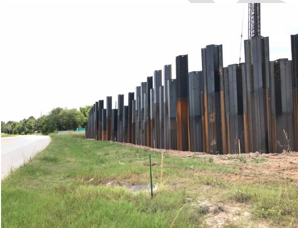
Figure 8.3.28: Steel protective coating missing
