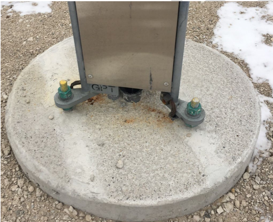
Figure 8.14.4: ESS tower foundation with triangular anchor bolt pattern
