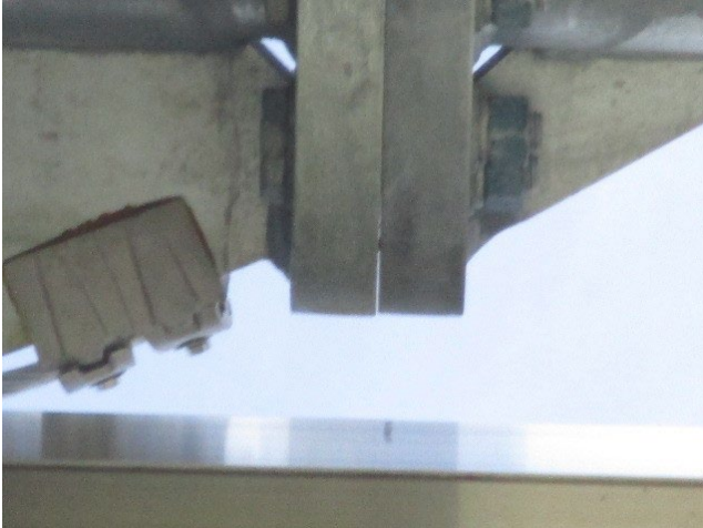
Figure 8.10.14: Horizontal structure connection, gap between arm connection flanges
