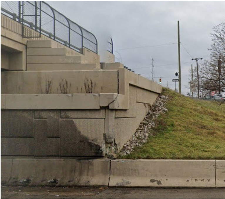
Figure 8.3.16: Impact damage
