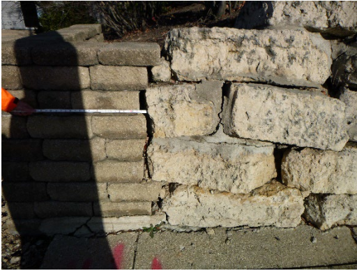
Figure 8.3.24: Wall misalignment
