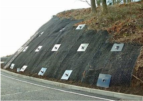
Figure 8.3.31: Typical soil nail wall
