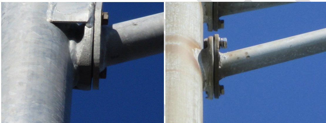
Figure 8.11.21: Frangible and non-frangible pole structure vertical structure connections, gap at arm flange (left), loose arm connection bolt (right)
