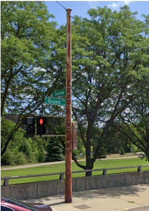
Figure 8.5.12: Embedded Pole with heavy corrosion, concrete sidewalk covering embedment material
