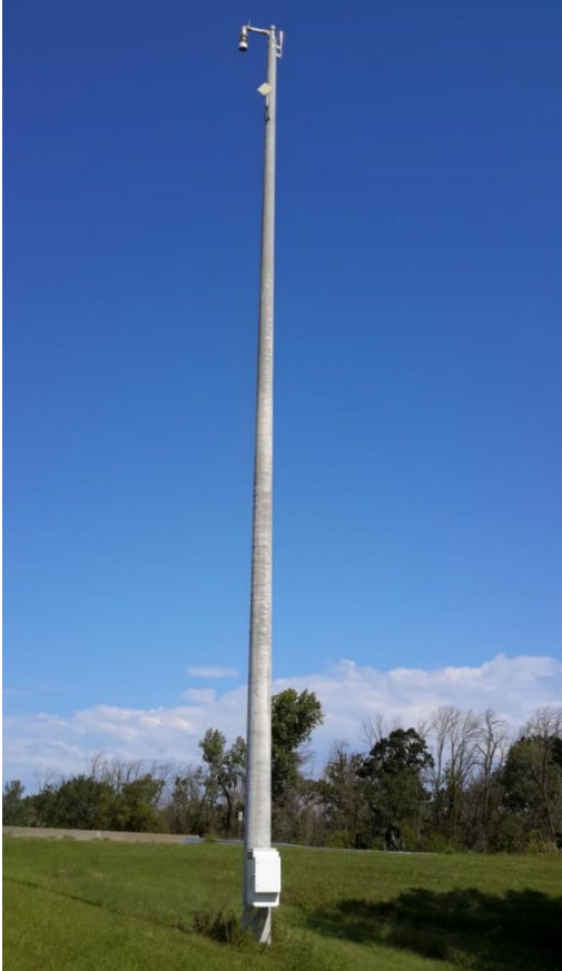
Figure 8.6.1: Spun Concrete Pole
