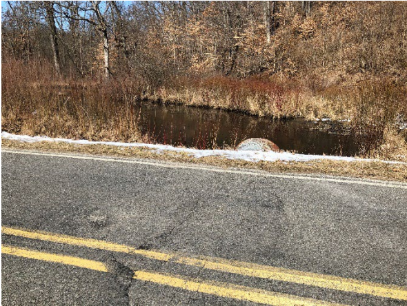
Figure 8.2.5: Transverse cracking of pavement above culvert
