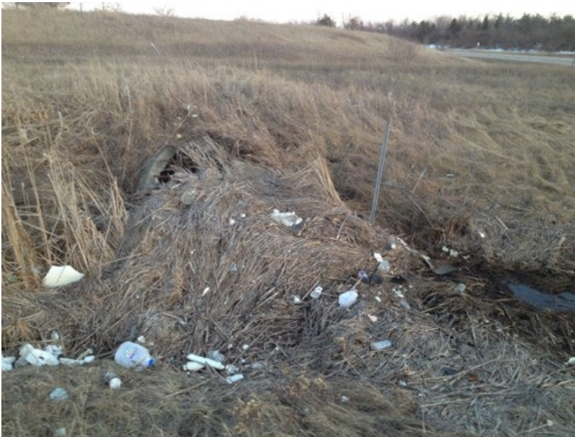
Figure 8.2.17: Blocked inlet
