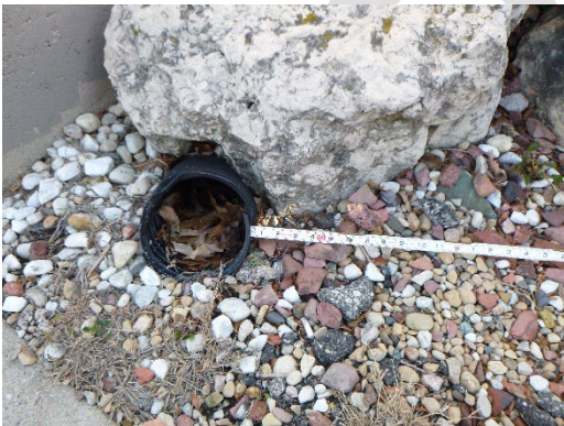
Figure 8.3.42: Drainage outlet is partially clogged with leaves and debris
