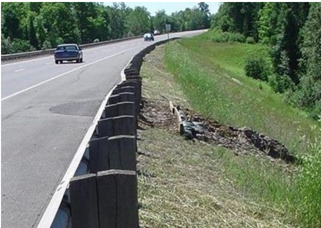
Figure 8.2.9: Example of embankment failure above a culvert
