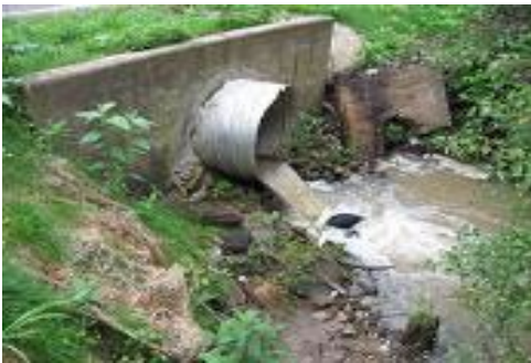
Figure 8.2.16: Vertical alignment distress; may have progressing washout due to high flow
