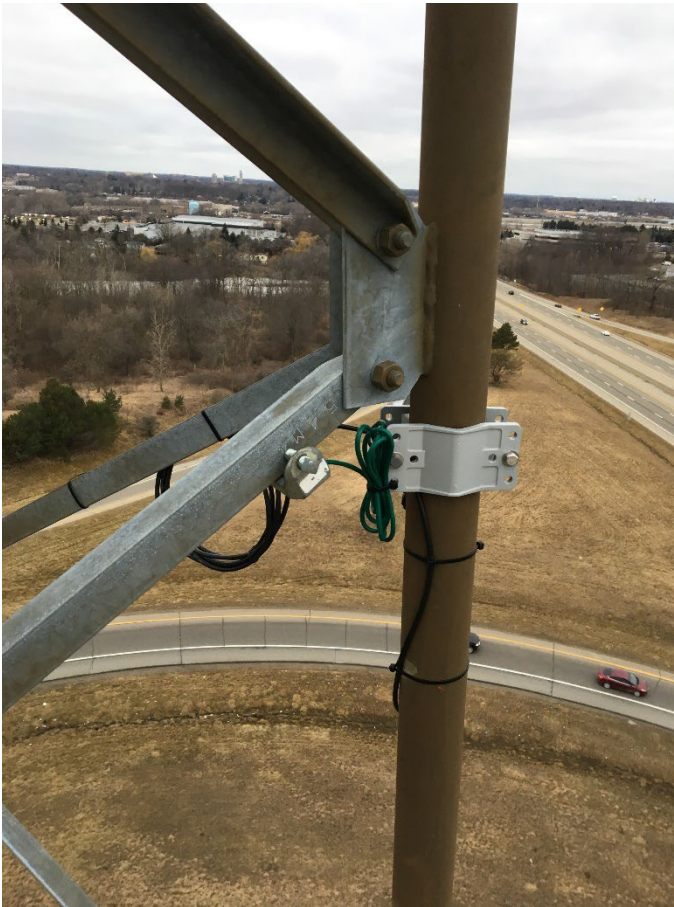
Figure 8.13.5: Bracing showing vertical structure bolted connection to vertical support
