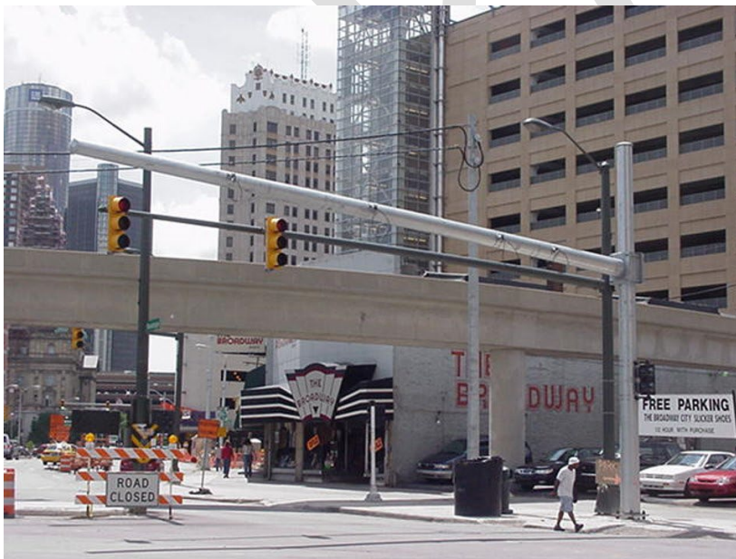
Figure 8.9.1: MDOT Category I Mast Arm, note previous design in background before removal
