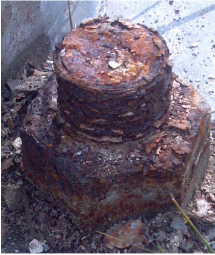
Figure 8.11.9: Anchor bolt and leveling nuts foundation, non-frangible base anchor bolt corrosion
