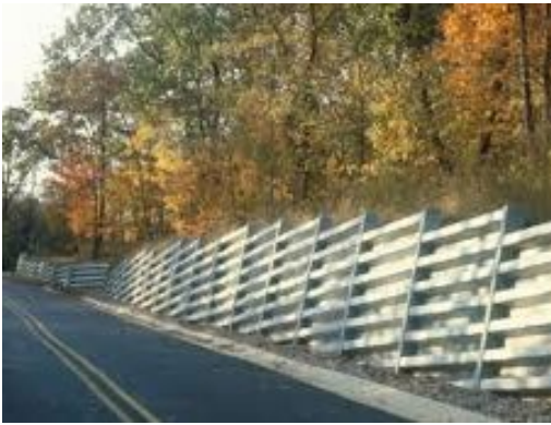
Figure 8.3.26: Typical metal bin wall
