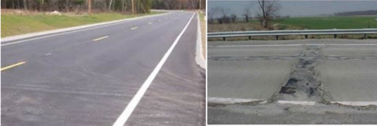
Figure 8.2.3: Approach roadway, without observable distress (left), clear distress over culvert (right)
