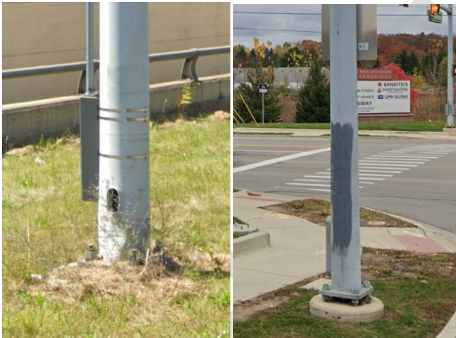
Figure 8.7.12: Impact damage and missing hand hole cover (left) and graffiti/coatings repair (right)
