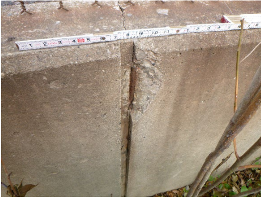
Figure 8.3.10: Concrete spall with corroded reinforcing
