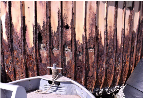
Figure 8.3.27: Steel corrosion and section loss
