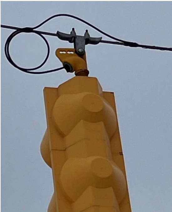
Figure 8.7.18: Span wire hanger
