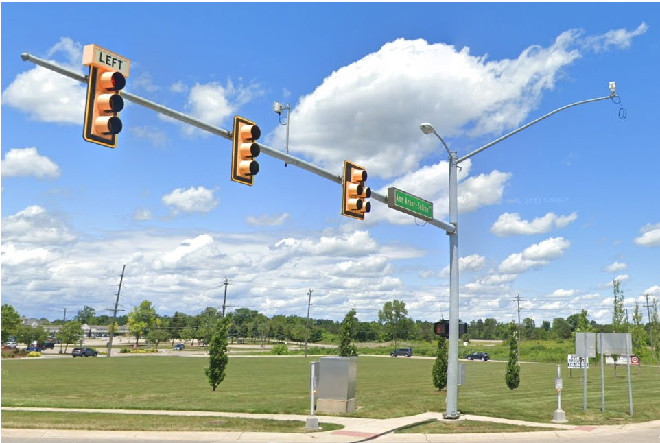
Figure 8.9.16: Mast arm structure supporting signals, sign, luminaire, camera, and sensor
