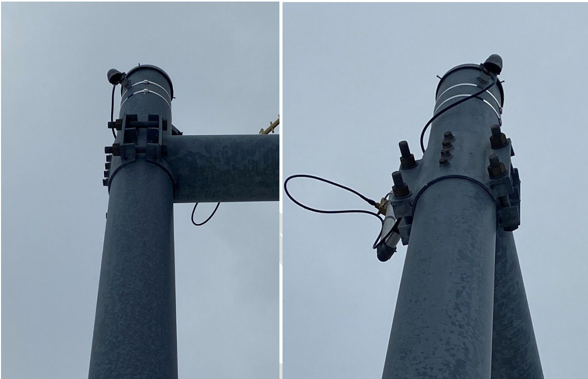
Figure 8.9.10: Mast arm to pole vertical structure connection, saddle clamp type
