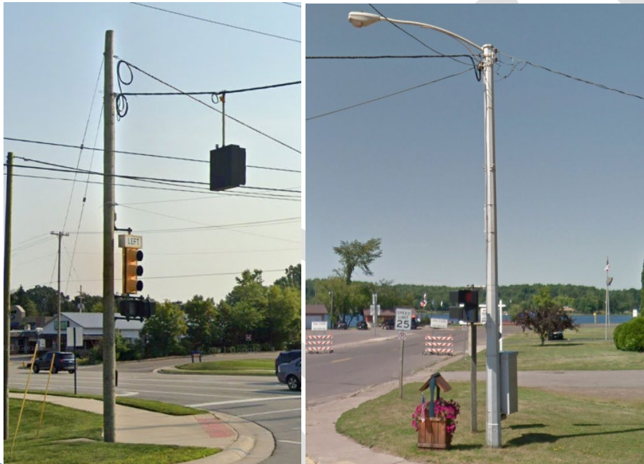
Figure 8.5.1: Embedded wood pole (left) and embedded steel pole (right)
