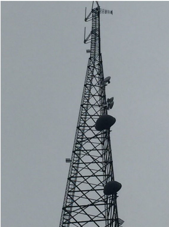
Figure 8.13.4: Communication tower with vertical supports and diagonal and horizontal bracing
