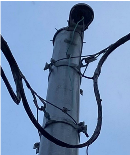
Figure 8.7.13: Steel strain pole band clamp connections for span wires
