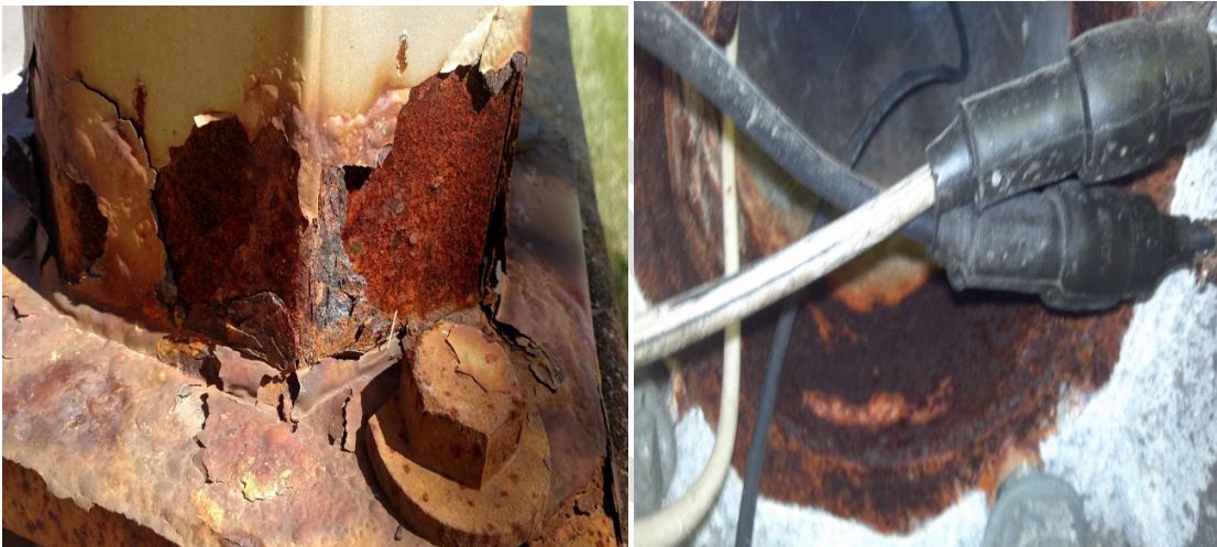
Figure 8.11.17: Non-frangible pole structure vertical support column (upright), coating system failure and corrosion in upright at base weld (left), corrosion inside column (right)
