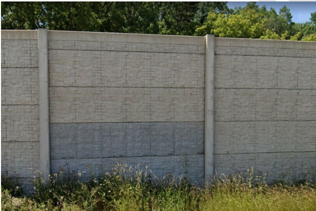
Figure 8.8.8: Noise wall with vertical joints at posts and horizontal contacts between panels
