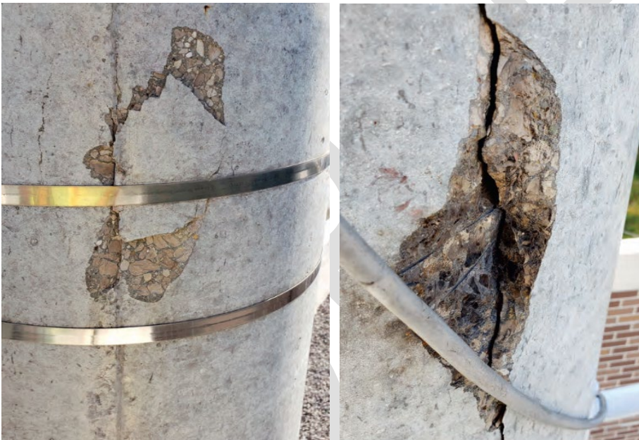
Figure 8.6.6: Spalls (left), major cracking and spalls (right)
