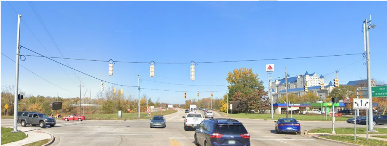
Figure 8.7.1: Steel strain poles with box span configuration
