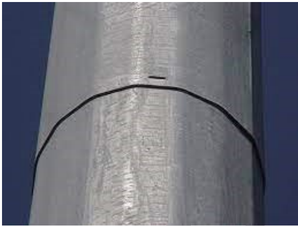
Figure 8.12.6: HMLT pole splice
