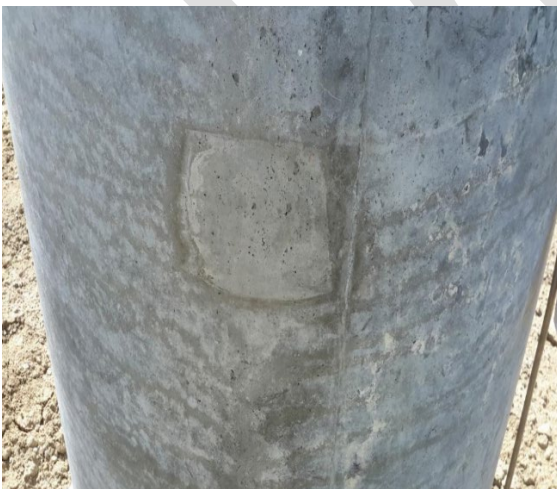
Figure 8.6.4: Sound patch area
