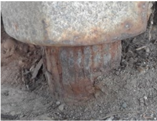
Figure 8.10.5: Anchor bolts and leveling nuts, corrosion in anchor bolt below upright base with section loss
