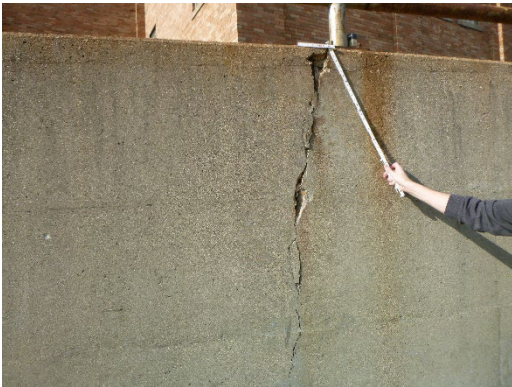
Figure 8.3.11: Spalled and delaminated concrete
