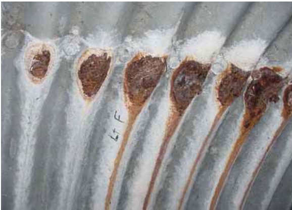
Figure 8.2.34: Corrosion of a metal culvert
