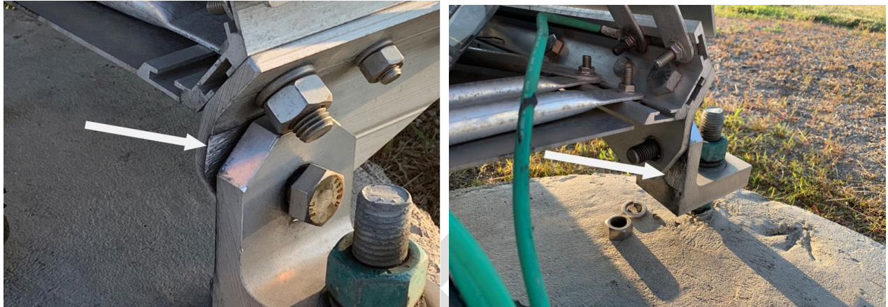
Figure 8.14.8: Evidence of wear on metal due to oscillation along with loose connection
