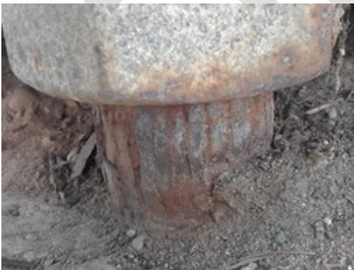
Figure 8.4.7: Cantilever or truss structure anchor bolts and leveling nuts, corrosion in anchor bolt below upright base with section loss
