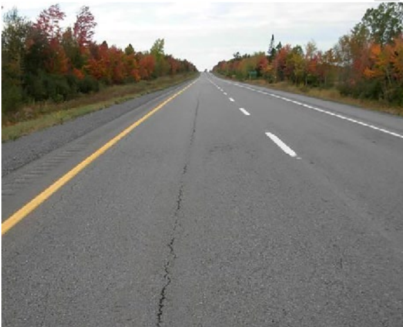
Figure 8.2.6: Longitudinal cracking
