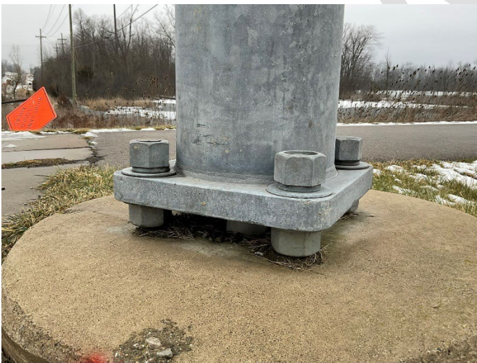
Figure 8.7.9: Anchor bolt negative projection – the top of the anchor bolt is not flush or higher than the top of the nut
