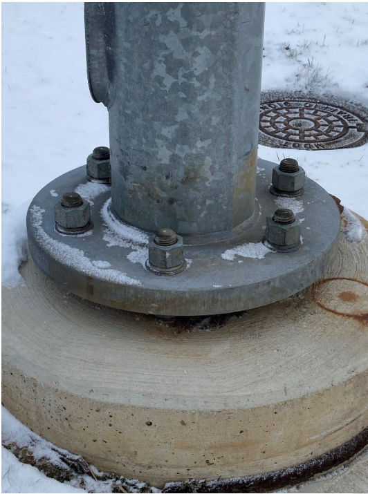
Figure 8.9.6: Six anchor bolt concrete foundation
