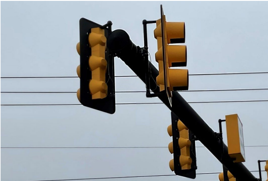
Figure 8.9.15: Mast arm signal and sign attachment connections
