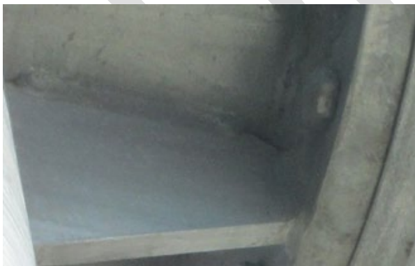
Figure 8.4.12: Vertical structure connection, missing flat washer on head side of bolt
