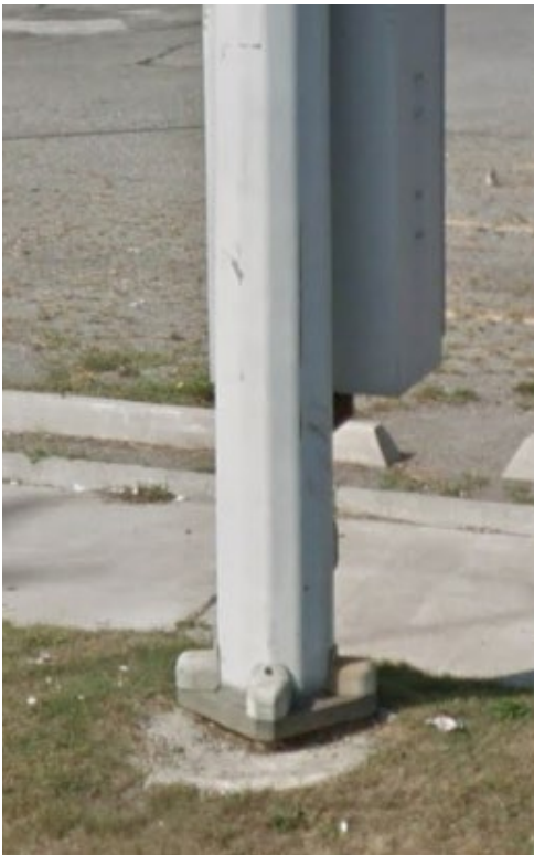
Figure 8.7.4: Steel strain pole (multi-sided) structure with four anchor bolts (left) and six anchor bolts (right)
