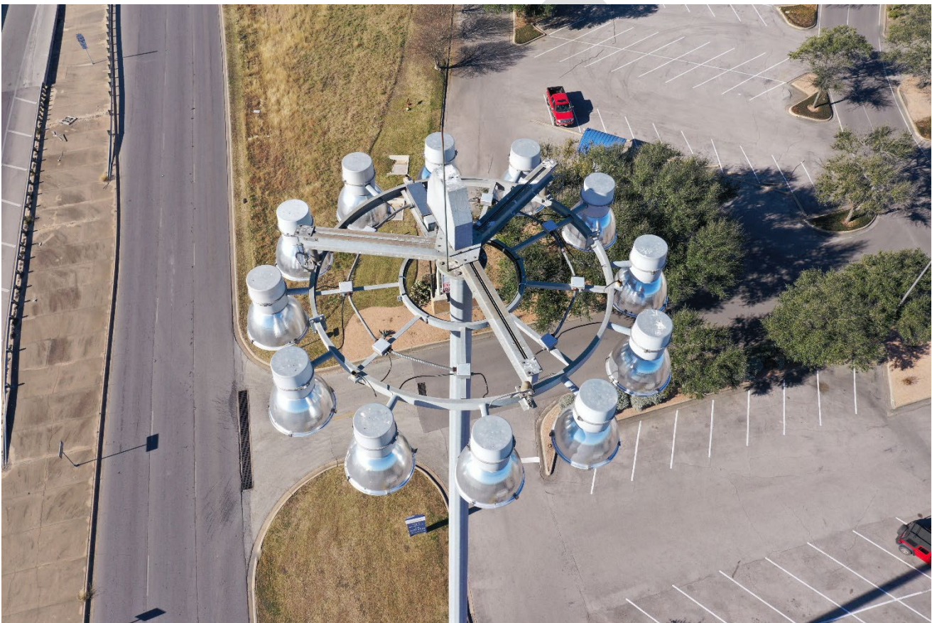
Figure 8.12.1: High-Mast Lighting Tower, aerial view of tower and lighting array from UAS
