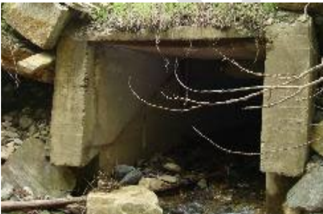
Figure 8.2.14: Vertical alignment issue leading to foundation undermining
