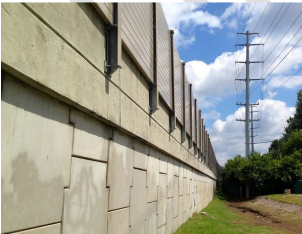
Figure 8.8.11: Noise wall attached to retaining wall
