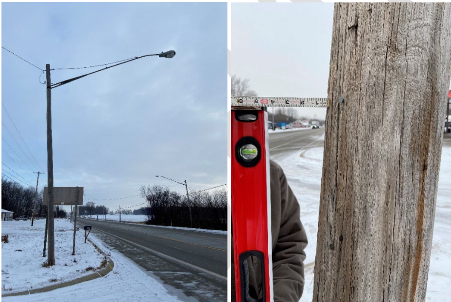
Figure 8.5.10: Measuring pole misalignment with a 4 ft. level
