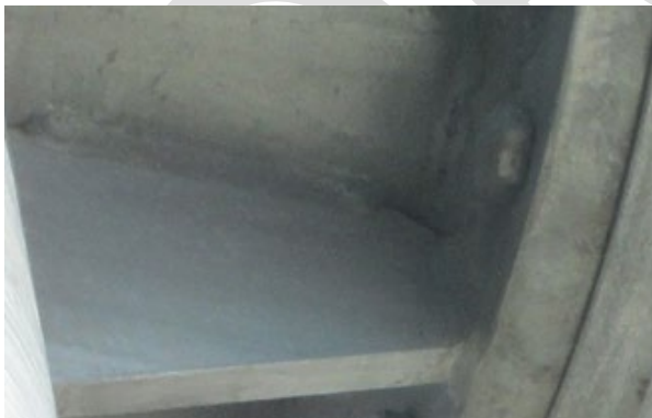
Figure 8.10.11: Vertical structure connection, missing flat washer on head side of bolt
