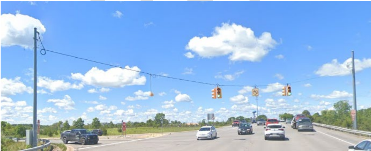
Figure 8.7.2: Steel strain poles with single diagonal span configuration
