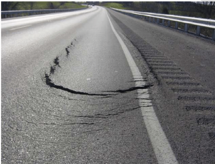
Figure 8.2.8: Slippage cracking
