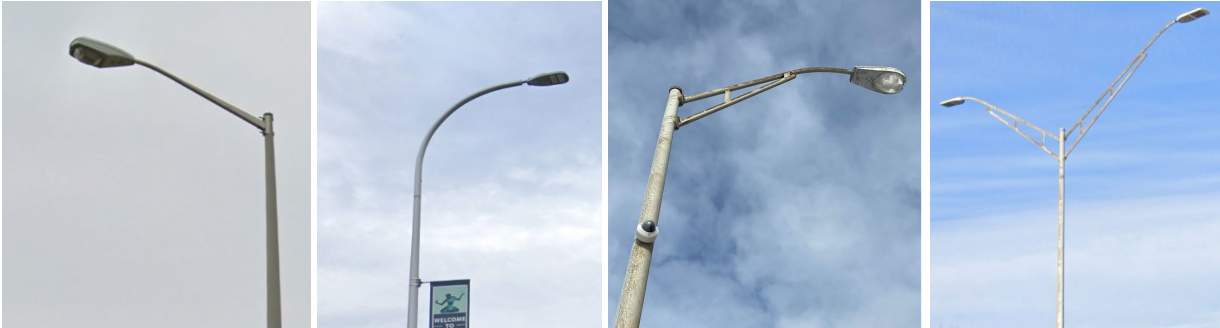
Figure 8.11.1: Pole structure arm types (numbering from left), single member (1), Davit member (2), single truss arm (3), double truss arm member (4)
