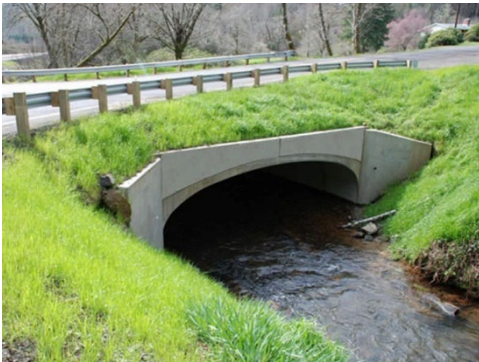
Figure 8.2.23: Concrete headwall and wingwall
