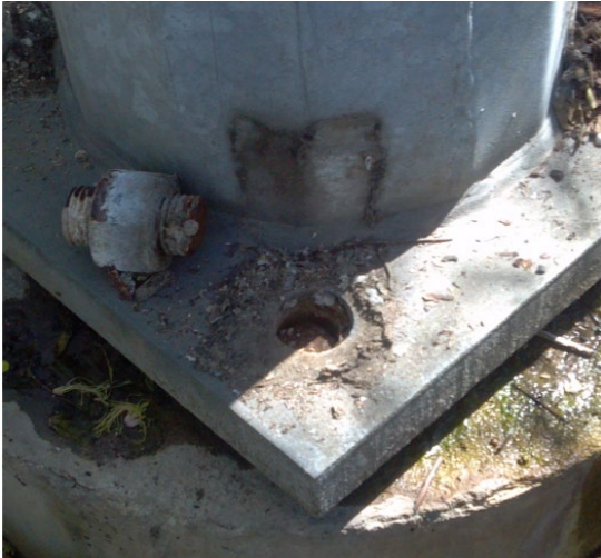
Figure 8.11.7: Anchor bolt and leveling nuts foundation, severed anchor bolt and nut of non-frangible base
