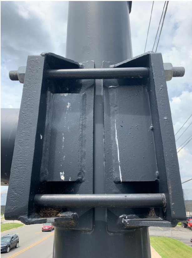
Figure 8.9.12: Mast arm vertical structure connection, note missing vertical weld on gusset plate
