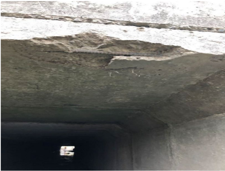
Figure 8.2.25: Spalled concrete at headwall
