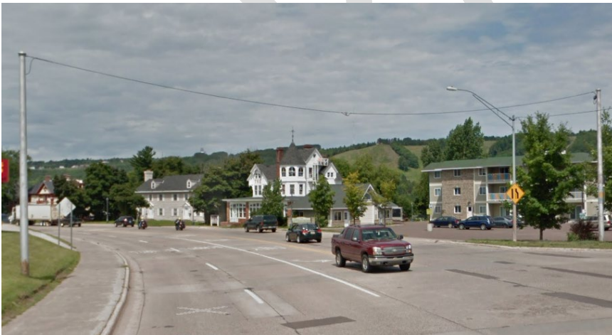
Figure 8.5.3: Embedded steel poles with single span configuration
