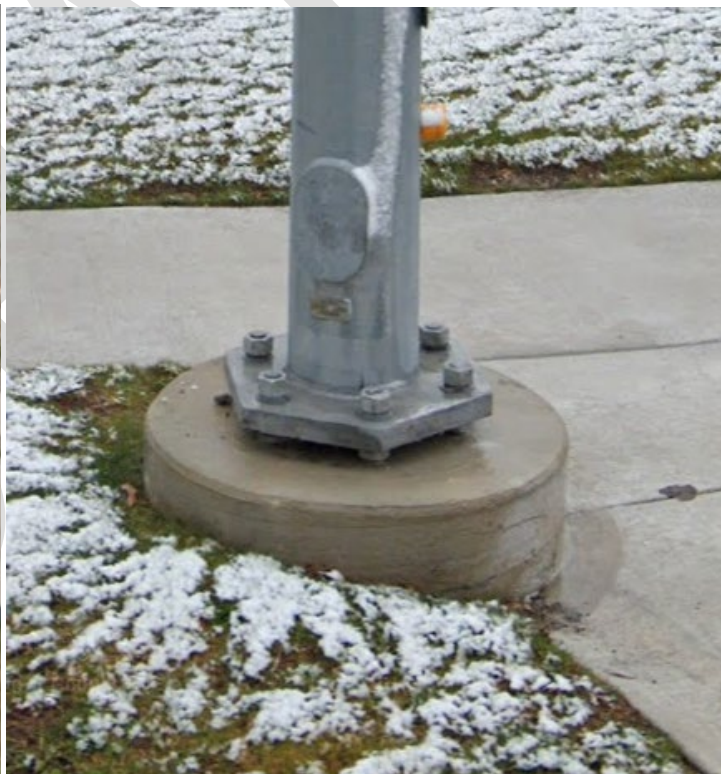
Figure 8.7.4: Steel strain pole (multi-sided) structure with four anchor bolts (left) and six anchor bolts (right)
