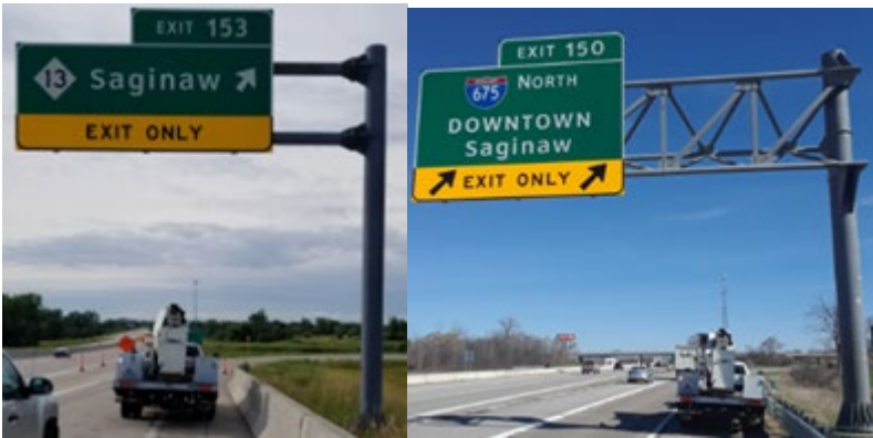
Figure 8.4.1: Cantilever structure, two-arm (left) and tri-chord style (right)
