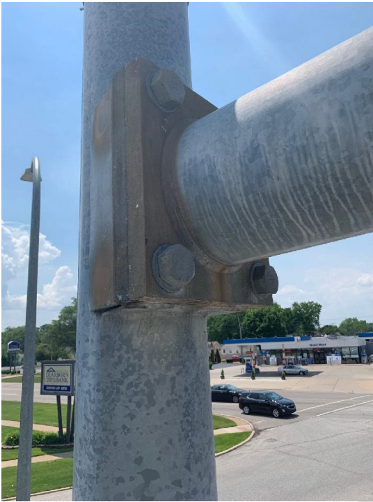
Figure 8.9.11: Mast arm to pole vertical structure connection, welded box type
