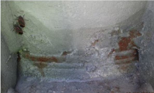
Figure 8.10.8: Vertical supports, rust underneath galvanizing repair
