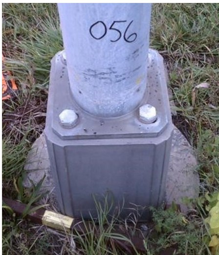
Figure 8.11.13: Frangible base connections, exposed bolt hole
