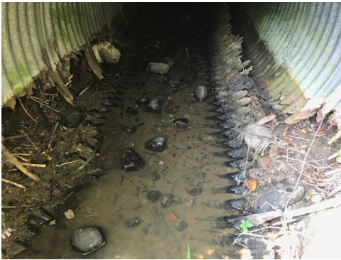
Figure 8.2.36: Abrasion wearing away corrugated metal pipe corrugations
