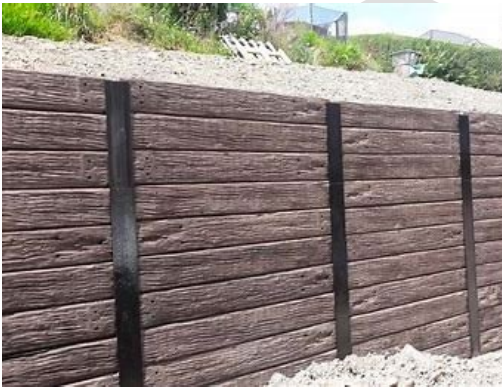
Figure 8.3.37: Vertical support steel
