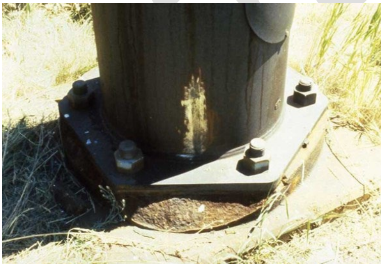
Figure 8.12.4: HMLT concrete foundation, spalling deterioration
