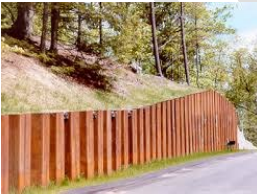
Figure 8.3.25: Typical sheet pile wall
