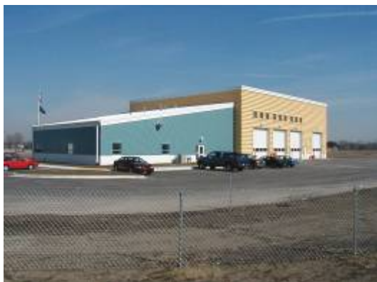
Blue Water Bridge Salt Storage and Maintenance Facility in Port Huron
