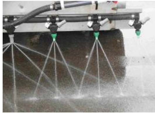
Application of Anti-icing Solution photo courtesy of Cryotech Deicing Technology
